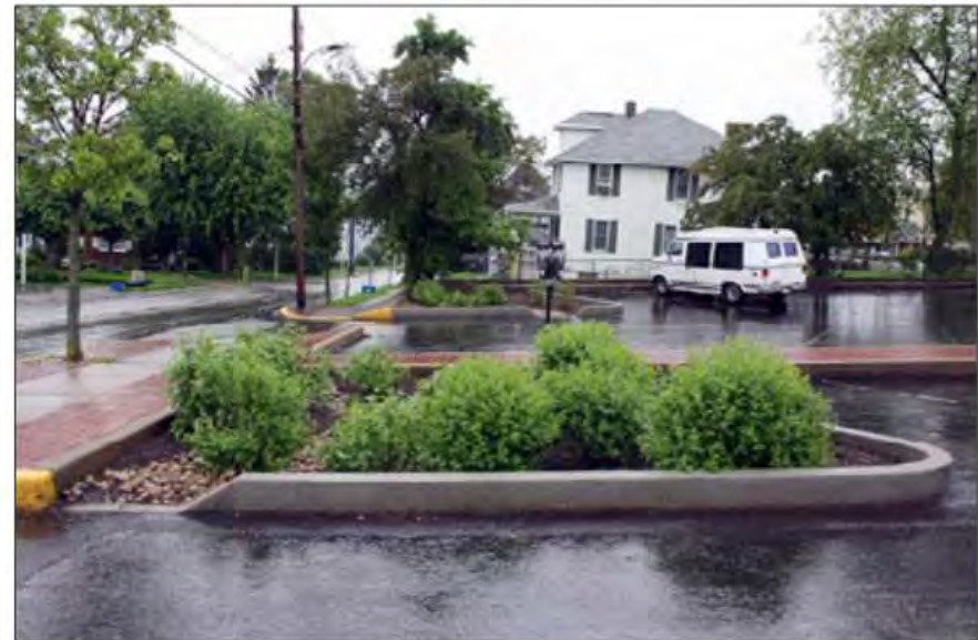
Two years after installation and numerous rain events, the parking lot rain gardens successfully capture and treat runoff from each storm.
