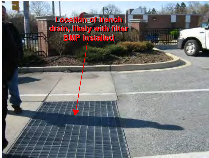
Photograph 2. Rite Aid – Location where City SWM Program staff believed an inlet filter BMP was installed.
