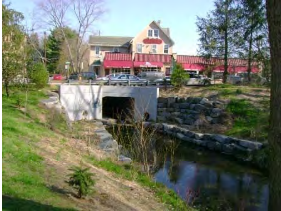
Photograph 71. Stony Run Stream Restoration – View of results from Phase II activities.
