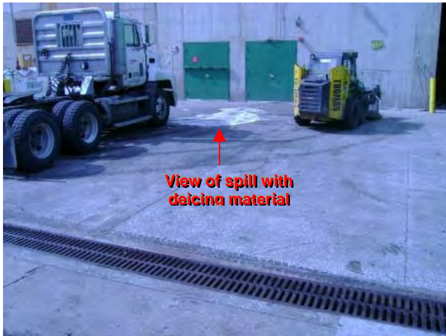
Photograph 60. Northwest Transfer Station – View of an apparent petroleum spill at the loading dock. The inspectors noted that deicer had been placed on the spill in an apparent attempt to clean up the spill.
