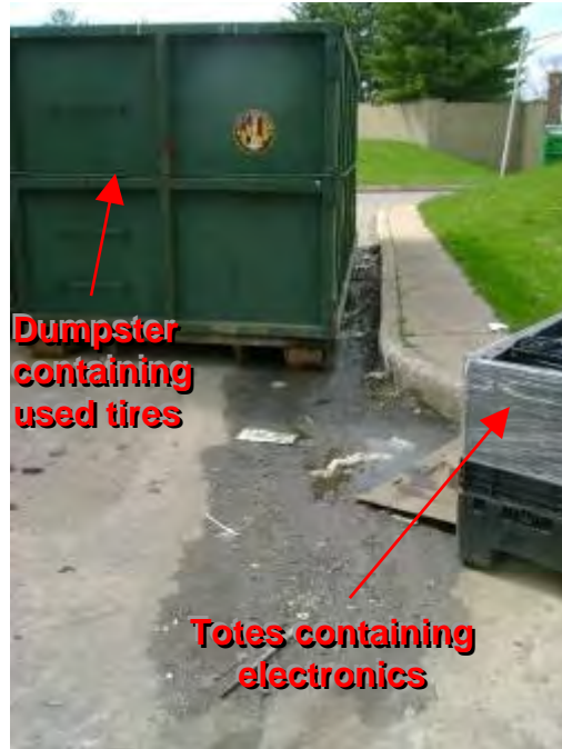
Photograph 51. Northwest Transfer Station – View of drainage area for storm drain. NOTE: Poor housekeeping and lack of BMPs to protect storm drain.
