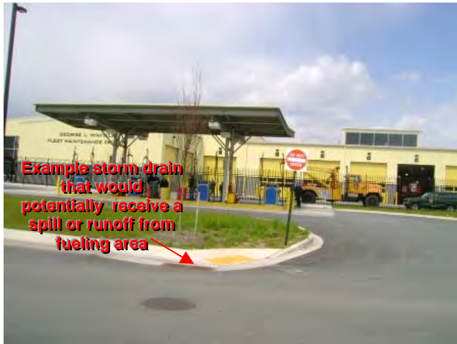
Photograph 46. Central Garage – View of new City vehicle fueling facility located outside of facility fenceline.
