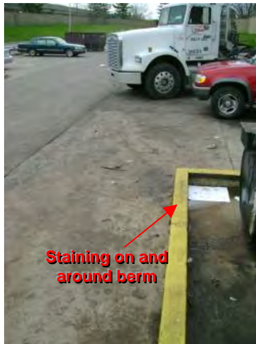
Photograph 48. Northwest Transfer Station – View of staining on and around outside of berm indicating that oil-laden stormwater had overtopped the berm.
