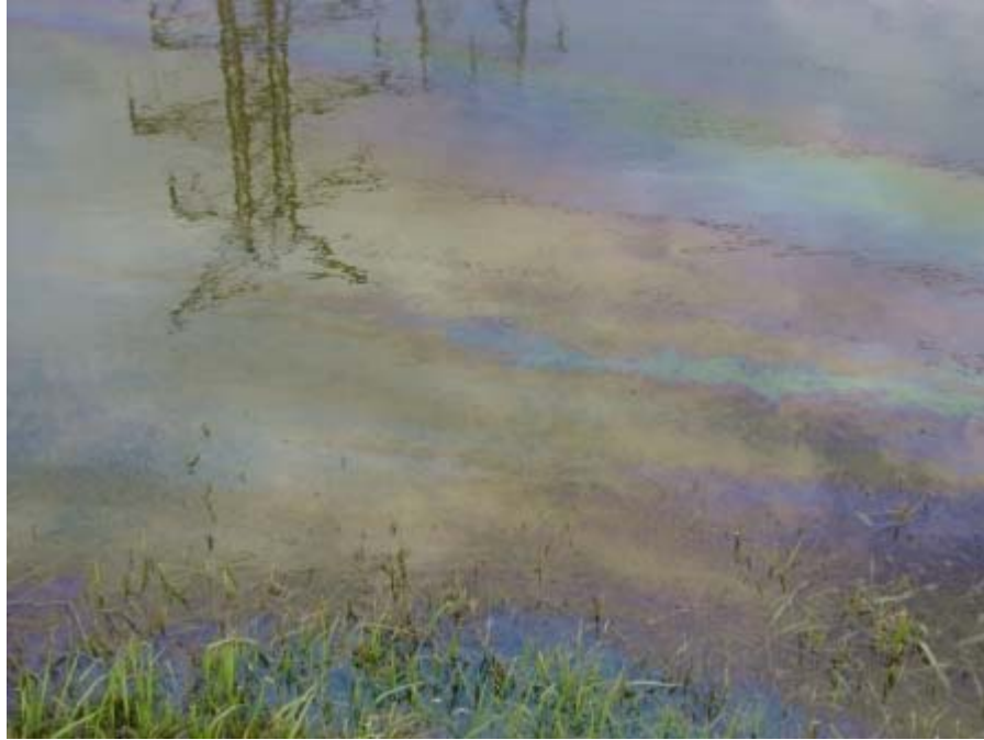
Photograph 43. Central Garage – Close up of sheen on water in pretreatment forebay.
