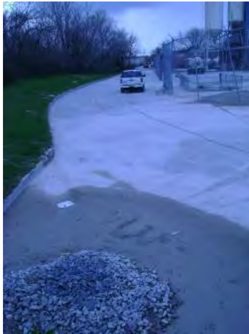
Photograph 12. S&G Concrete – Drain covered with filter fabric and stone.
