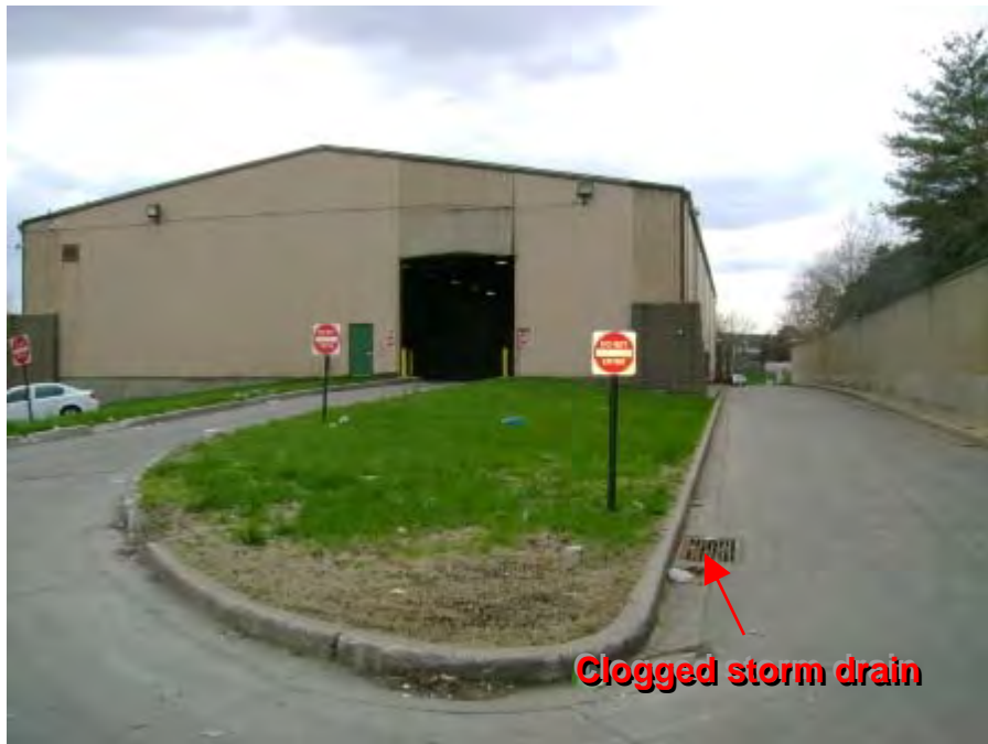
Northwest Transfer Station – View of recycling processing building exit. Storm drain in lower right is approximately 75% full of debris and sediment.
