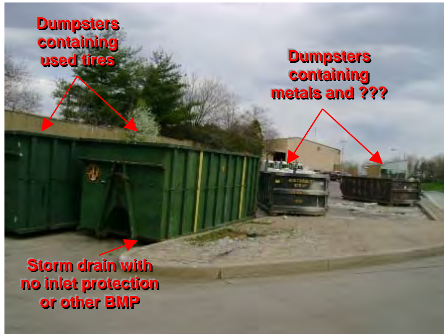
Photograph 52. Northwest Transfer Station – View of drainage area for another storm drain. (NOTE: Poor housekeeping and lack of BMPs to protect storm drain)
