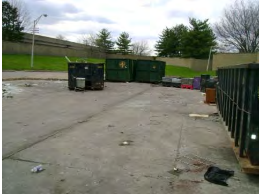
Photograph 49. Northwest Transfer Station – View of recyclable drop off area. Dumpsters contain metals, cardboard, and tires while totes contained electronics. Poor housekeeping was noted as well as a failure to provide BMPs such as inlet protection for storm drains.
