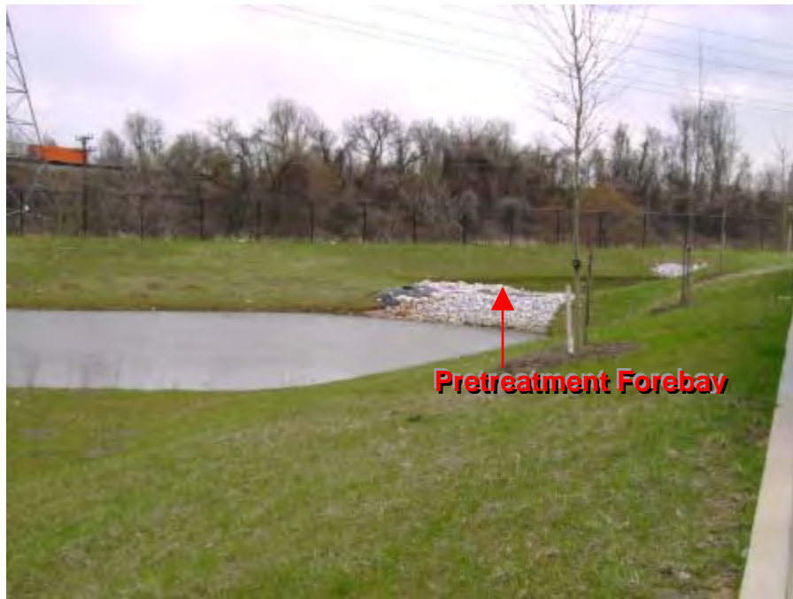
Photograph 40. Central Garage – View of storm water pond and pretreatment forebay.
