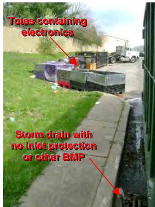
Photograph 50. Northwest Transfer Station – View of drainage area for storm drain. (NOTE: Poor housekeeping and lack of BMPs to protect storm drain)
