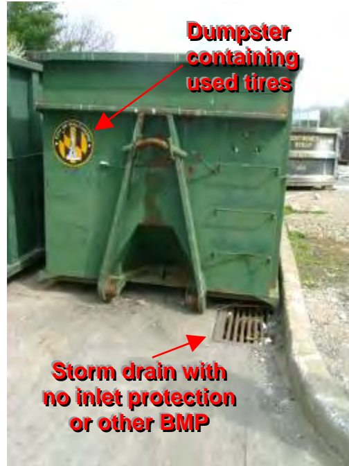
Photograph 53. Northwest Transfer Station – Close up of storm drain with no inlet protection from previous photo.
