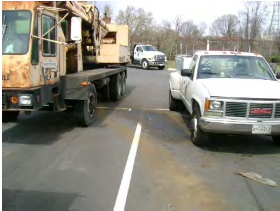
Photograph 28. Central Garage – Example of staining on paved area.
