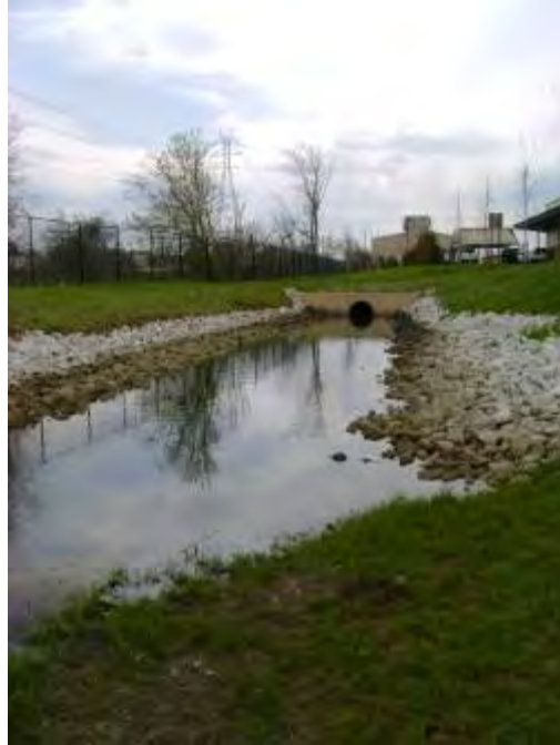
Photograph 41. Central Garage – View of pretreatment forebay with staining noted around the perimeter and a sheen on top of the water.
