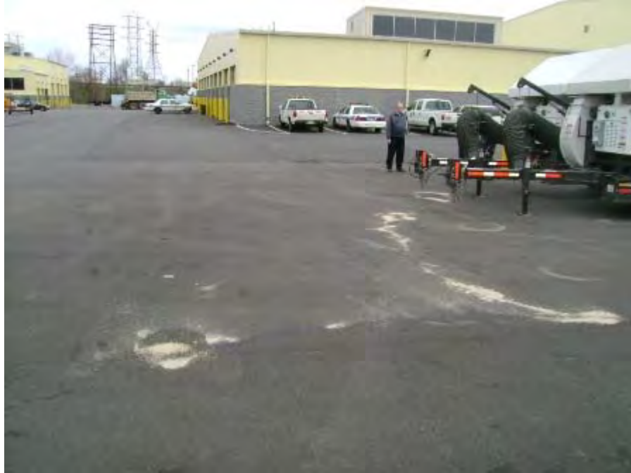
Photograph 35. Central Garage – View of oil absorbent placed on pavement to clean up a small spill.
