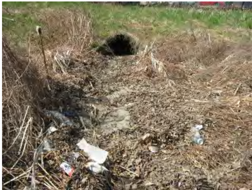
Photograph 4. American Red Cross (SWM No. 32) – View of fugitive trash and fine debris accumulation at inlet.
