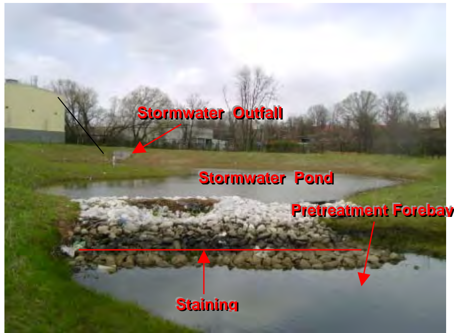
Photograph 38. Central Garage – View of stormwater pond and outfall. (NOTE: Oil stains around pretreatment forebay)
