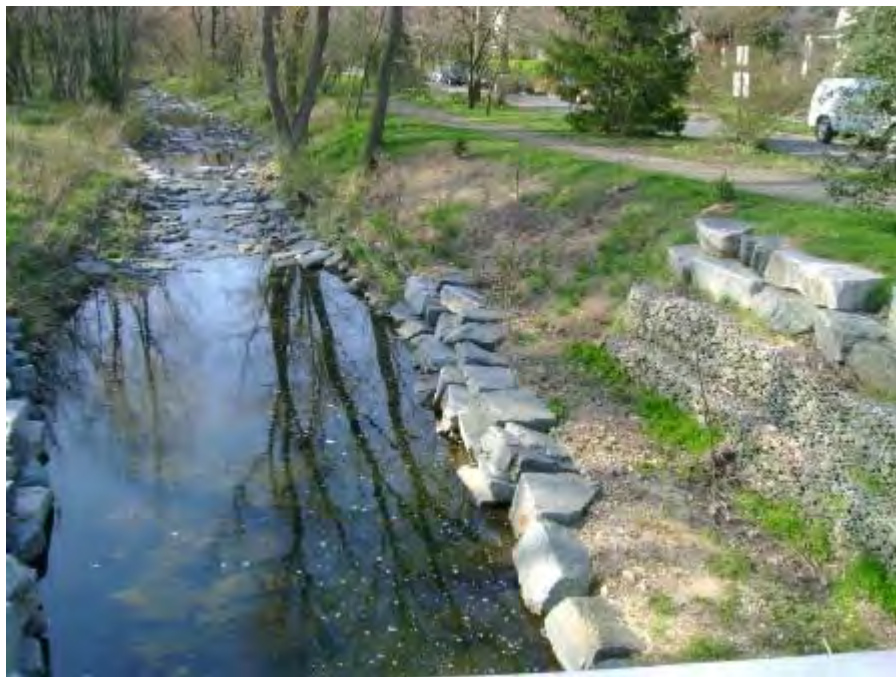
Photograph 70. Stony Run Stream Restoration – View of results from Phase II activities.
