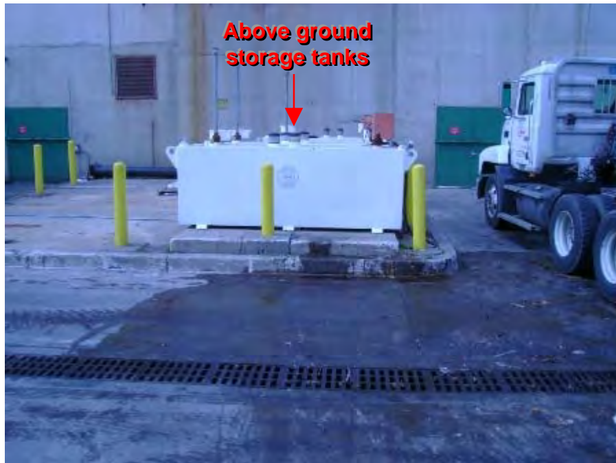
Photograph 62. Northwest Transfer Station – View of a large spill in the loading dock area (separate from spill with deicing material) to a trench drain. The facility representative stated that he was not aware of the cause of the spill, but did state that the three above ground storage tanks were not in use.
