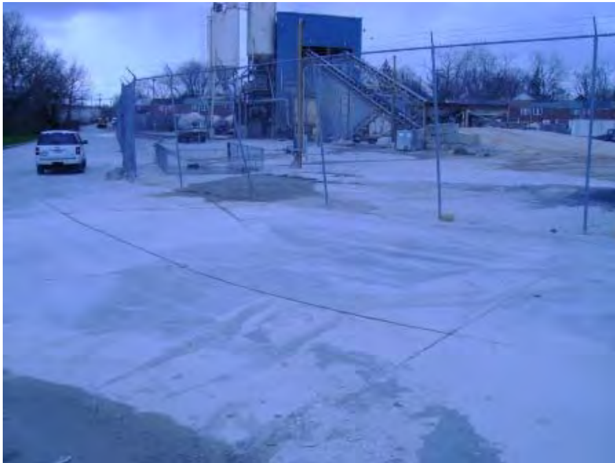
Photograph 14. S&G Concrete – View of facility from storm drain.
