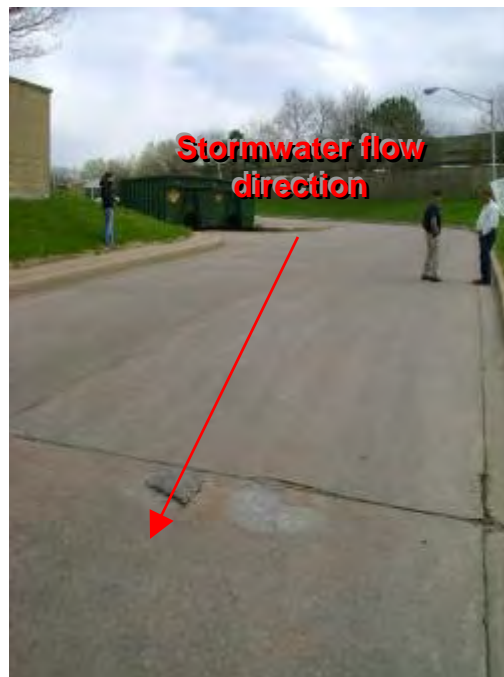
Photograph 54. Northwest Transfer Station – View of recycling area from facility entrance.
