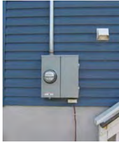
Elevated utilities in Yardley Borough, Bucks County, PA (from PEMA)
