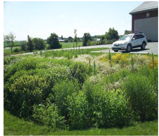
Retro-fitted Detention Basin
