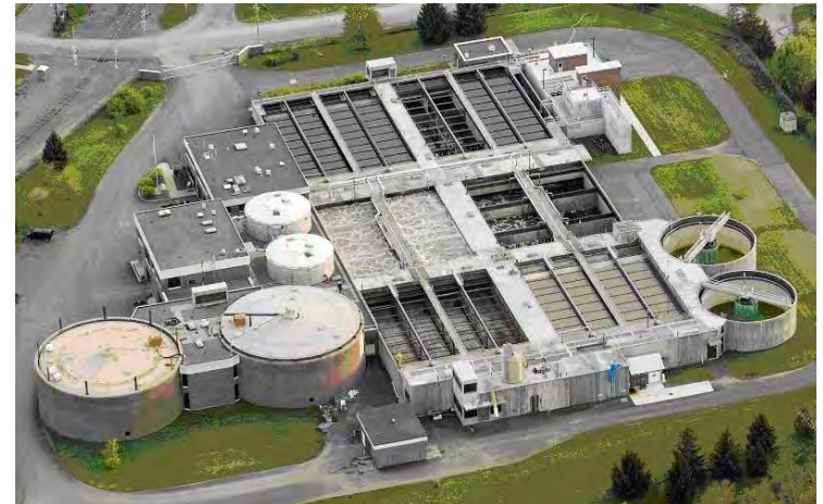
Conventional Sewer Plant
