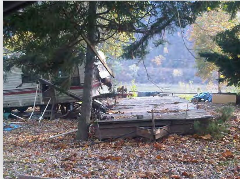
Tunkhannock Township, Wyoming County, PA (from FEMA Region III) A recreational vehicle washed into a manufactured home.
