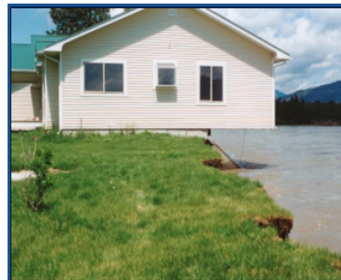
Clark Fork River, outside of Plains, Montana. Originally house was 30-40 feet from river bank and 1" above BFE.
