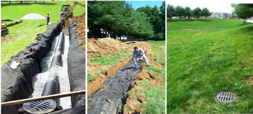
Figure 3: Example of Infiltration Trench Installation
