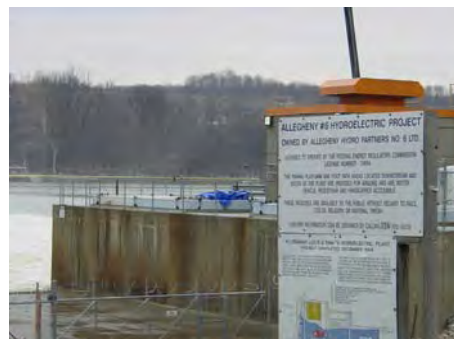
Hydroelectric Plant at Lock & Dam 6
