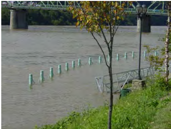
Flooding at Kittanning's Riverfront Park
