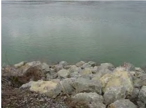
Streambank stabilization project at the mouth of Cowanshannock Creek
