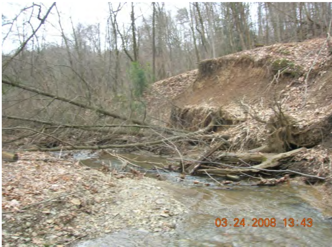
Photo 1: At a tributary of the North Fork, this slope failure and bank erosion was observed. (NF-T2W7)
