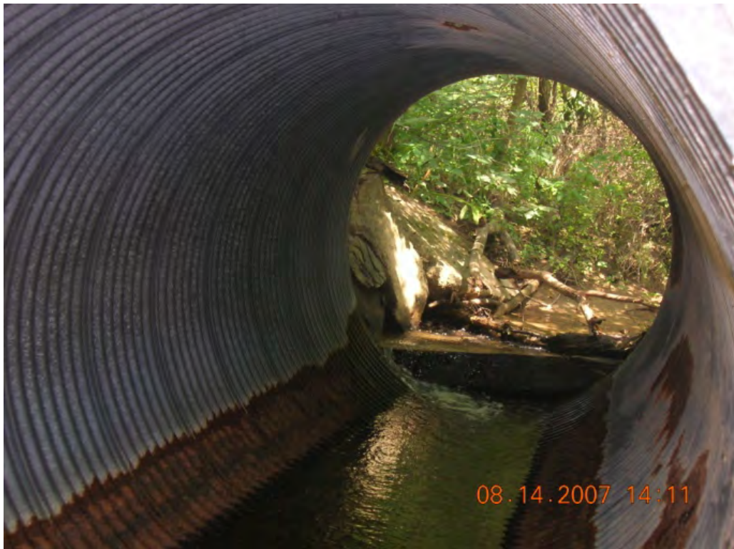
Photo 3: A culvert under a State Gamelands access road acts as a fish impasse. (EF-18)
