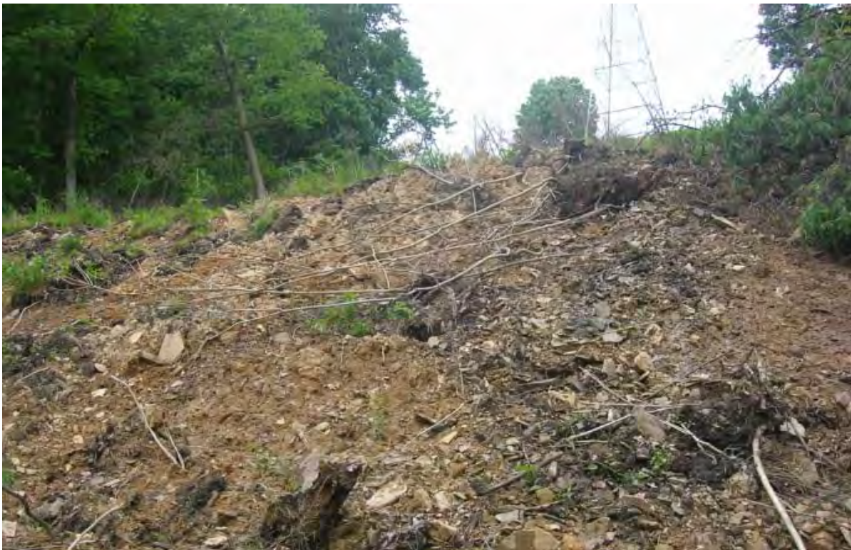
Photo 3: A landslide occurring along a power line, dumping sediment into the stream. (BSC-T1W7)
