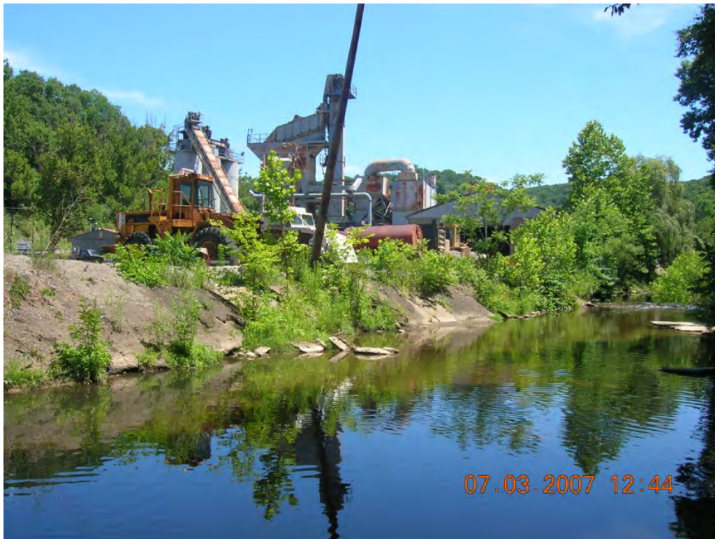
Photo 1: Hanson-Sewickley Creek Plant located right up on stream bank. (BSC-34)
