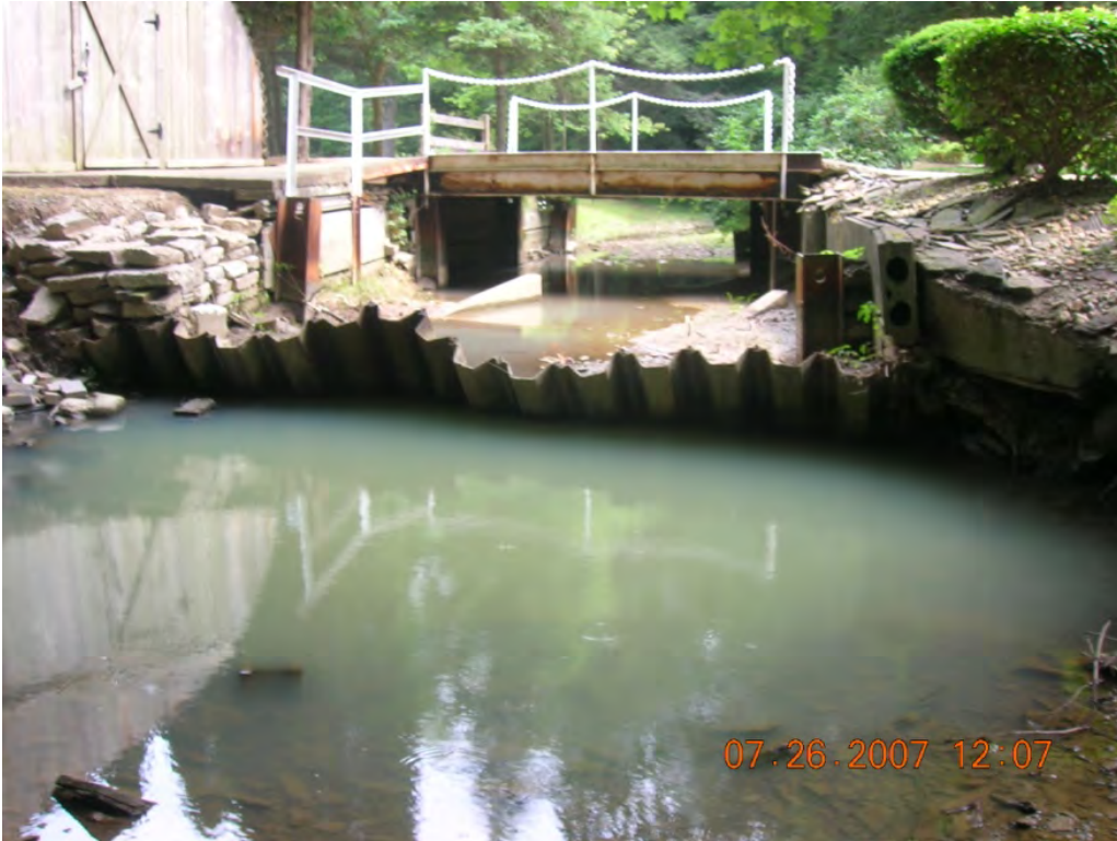
Photo 4: Here a homeowner placed a piece of metal in the stream, creating dam, but also a fish impasse and downstream sedimentation. (BSC-92)
