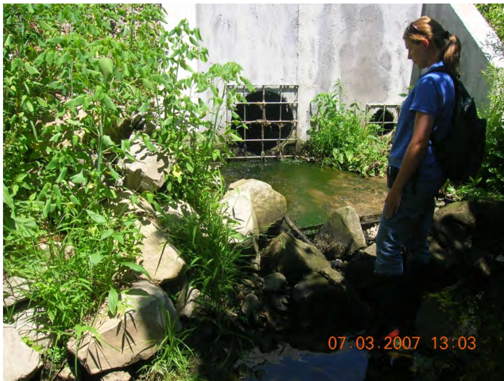
Photo 3: Greenish-black discharge from sewage plant. (BSC-36)
