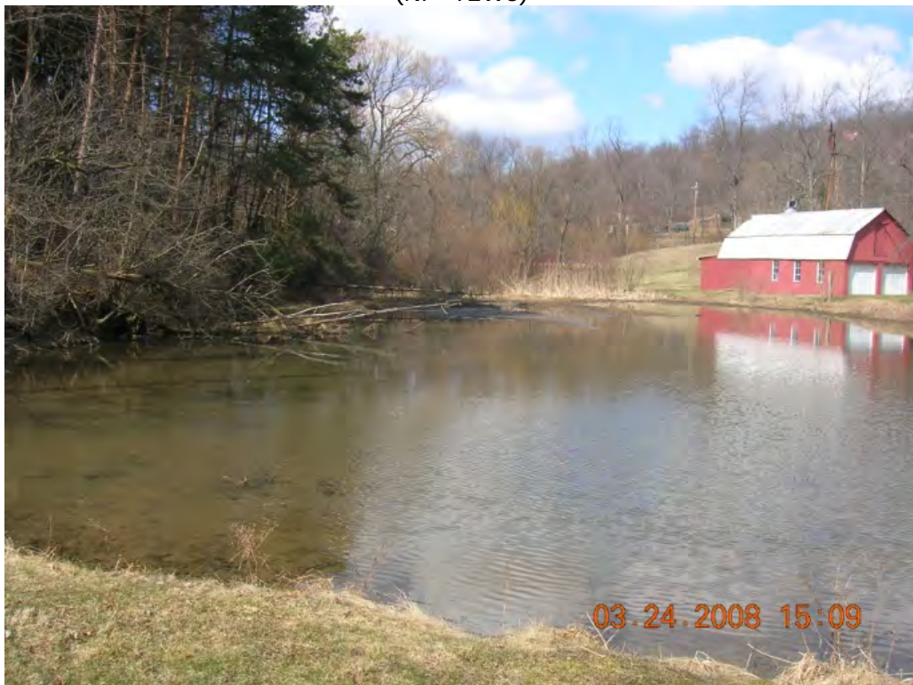
Photo 3: A pond along the tributary filled with excess sediment. (NF-T2W14)
