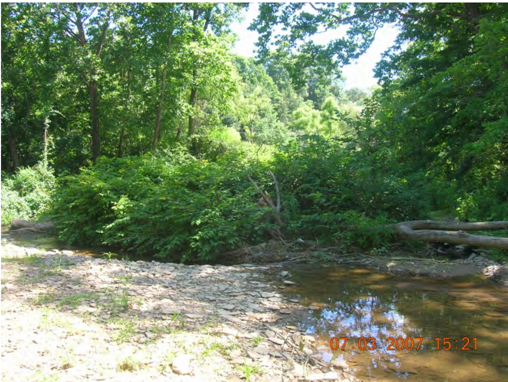
Photo 3: Large sediment build up and debris jam at a sanitary sewer crossing. (BSC-48)
