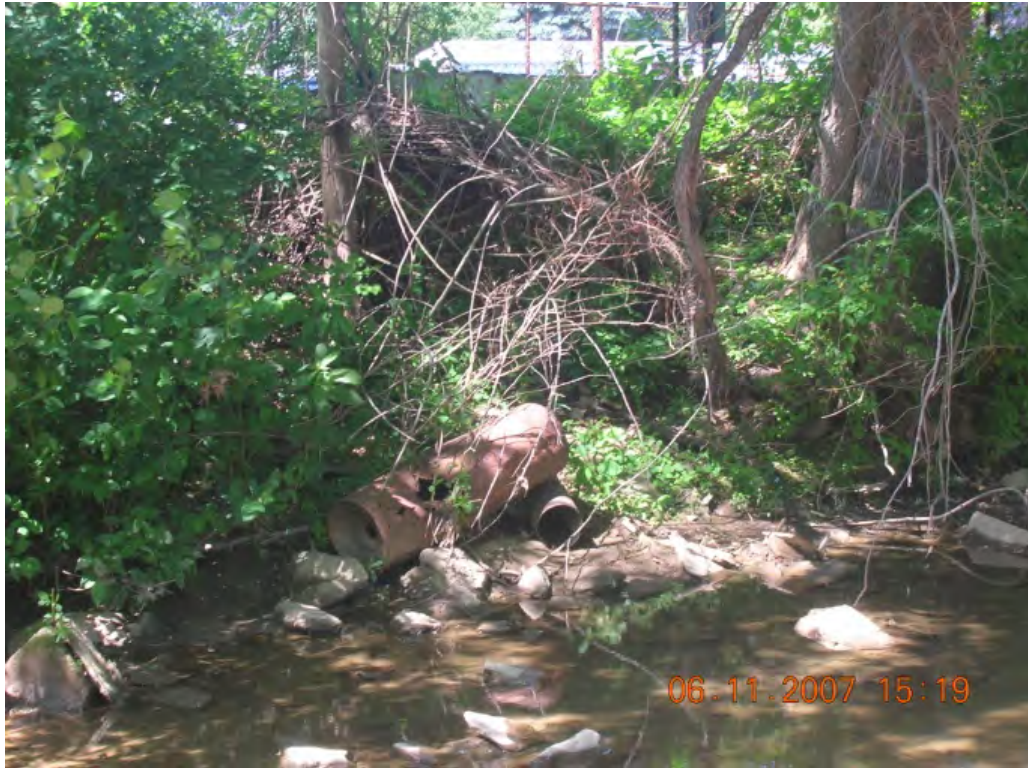
Photo 1: Sewage plant discharge from trailer court. (BSC-25)
