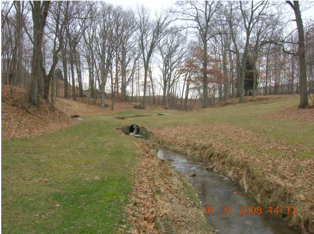
Photo 1: An improper attempt at bank stabilization using concrete blocks. (NF-37)
