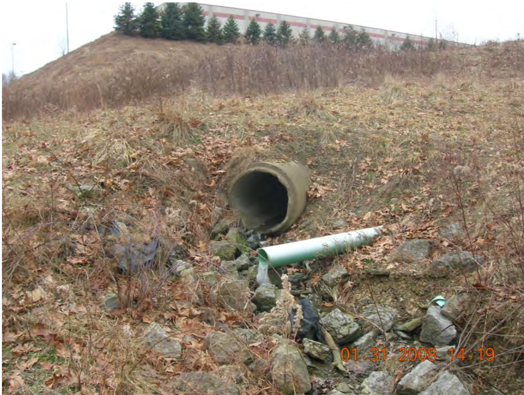
Photo 2: Storm water pond outlet from industrial park above that empties into the North Fork. (NF-38)
