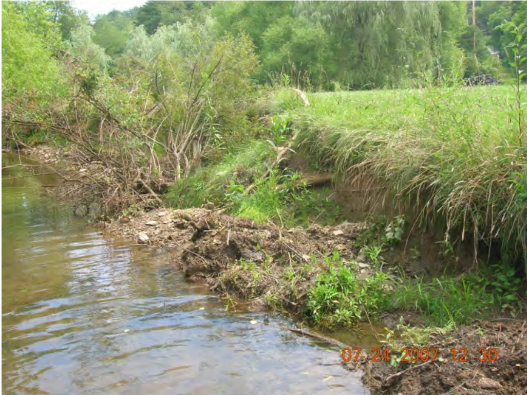
Photo 1: Bank erosion and massive slope failure in a homeowner's front yard. (BSC-67)
