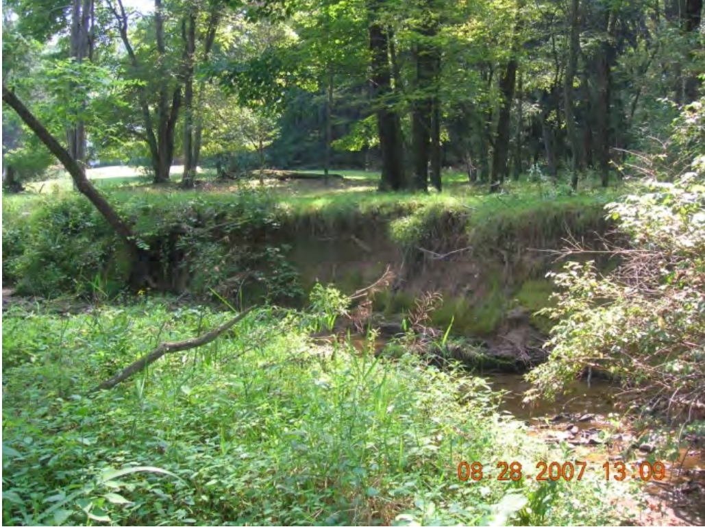
Photo 2: Bank erosion on a section of the East Fork just upstream of the Gamelands border. (EF-22)
