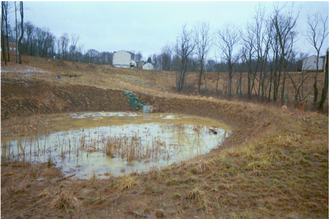
Photo 4: E&S Basin in Whispering Pines development. (NF-T5W11)
