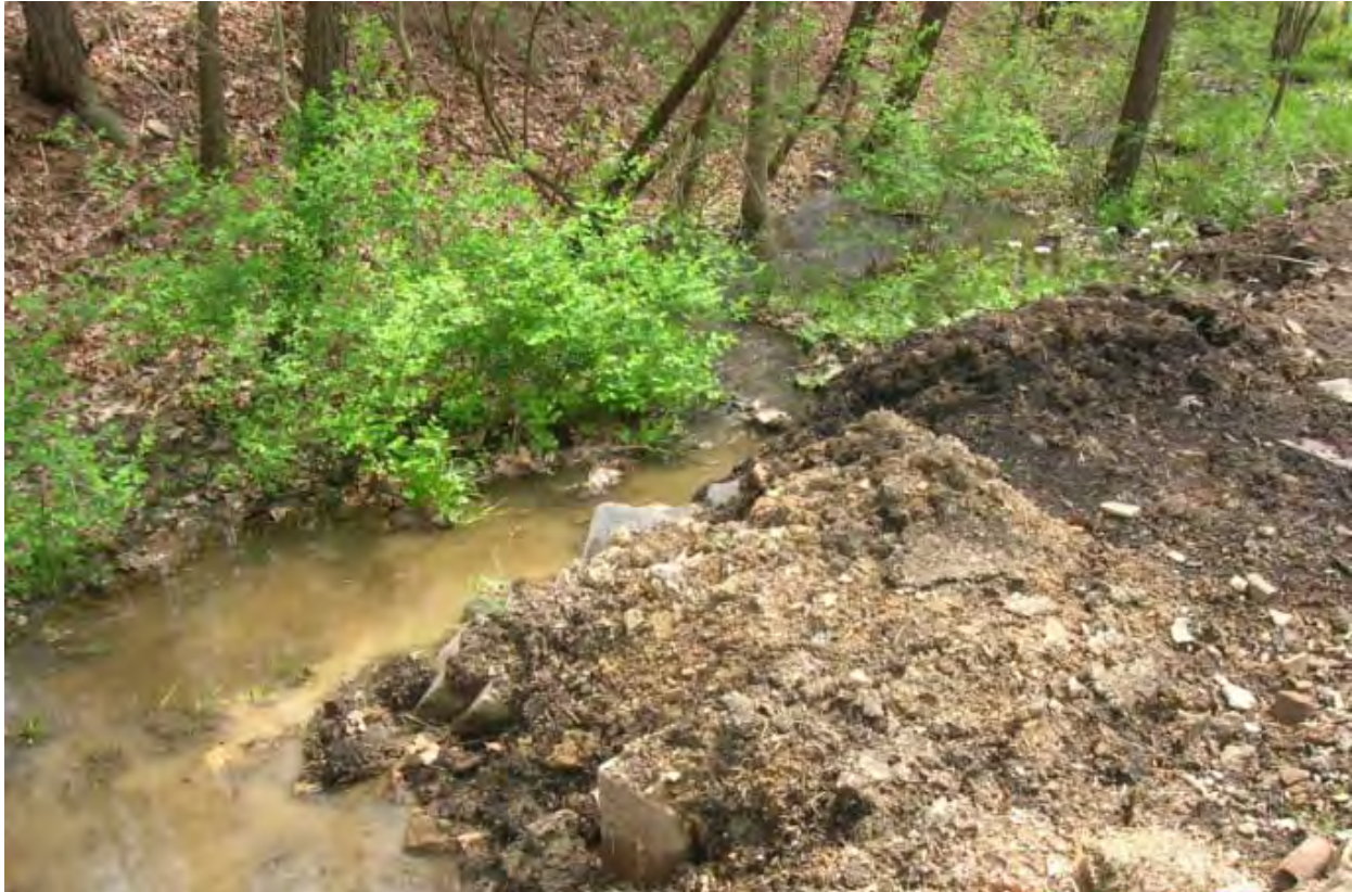
Photo 1: Mulch pile and disturbed ground encroaching on tributary off of Markman Park Road. (BSC-T3E2)
