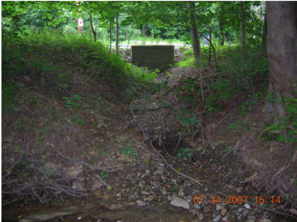
Photo 1: Drainage area coming off of road bringing in excess sedimentation. (BSC-84)
