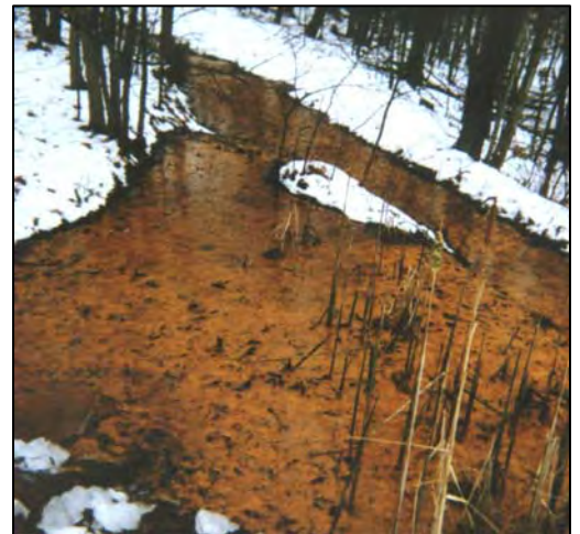
Existing treatment pond TB1 (Left) receives mine discharges MC1, MC2, and MC3 which emanate from the "McIntire" site. The effluent of TB1 (Right) used to be the headwaters of tributary #15. The natural formation of iron minerals at low pH, plugging old piping (Center), has been incorporated into the passive system design.
