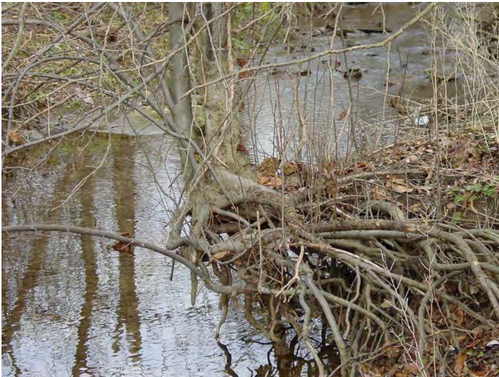
Figure 7 - Increased water velocity and increased bank scour results in the undercutting of trees.
