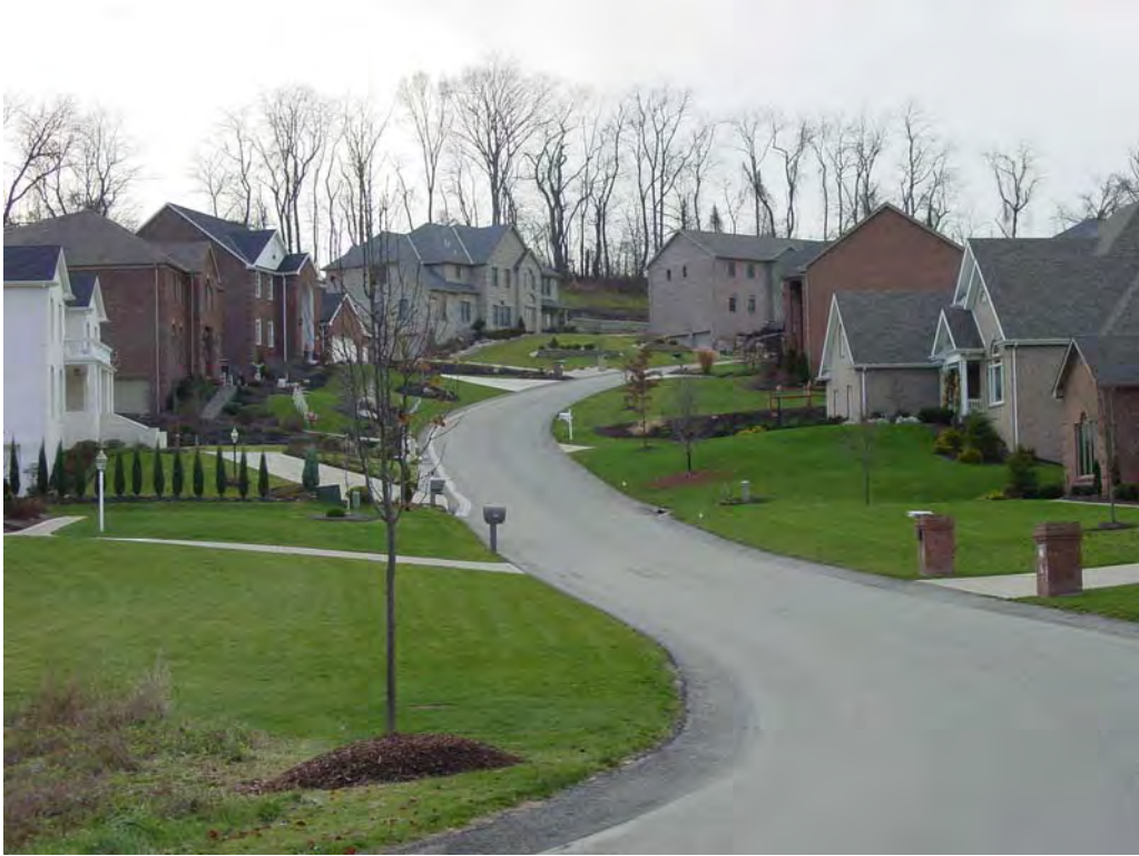
Figure 12 - Example of development on steep slopes with little or no runoff controls or retention.
