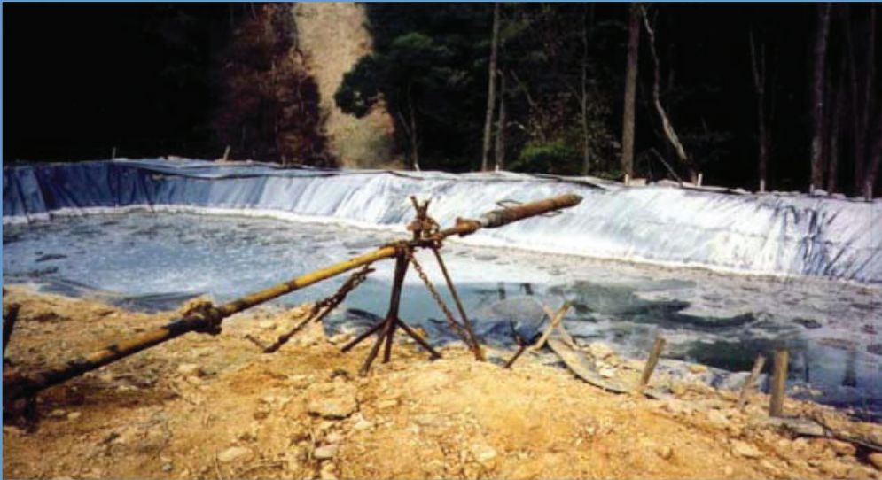
Figure 12: On-Site Storage of Fracturing Fluid Prior to Disposal
