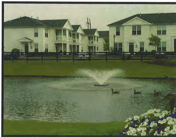
Retention basins are one type of stormwater BMP
