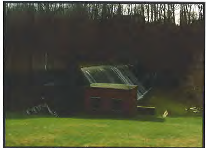
Canonsburg Lake Dam, 2007
