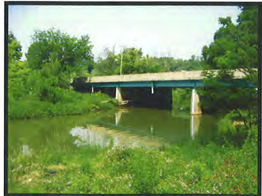
U.S. Route 19 bridge over Little Chartiers Creek
