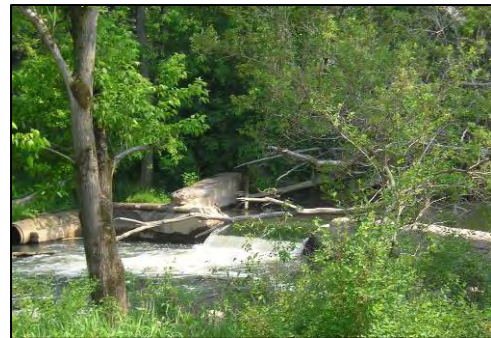
Breached dam on Thorn Creek below Saxonburg Water Treatment Facility
