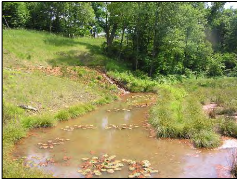
Passive AMD treatment system at Lutherlyn
