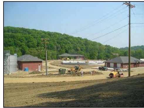
Constructing the new Saxonburg sewage treatment facility, summer 2007
