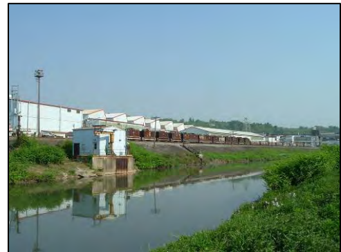
AK Steel Corporation Butler Works
