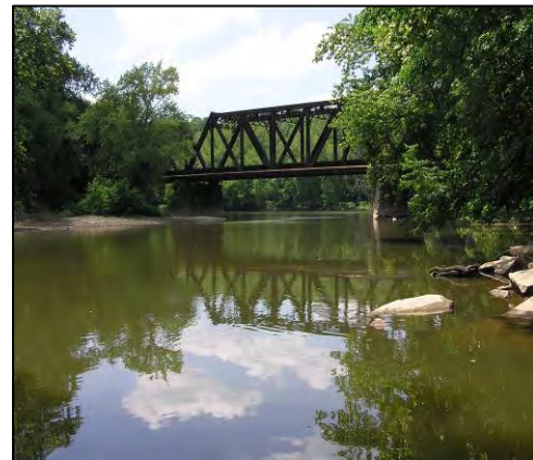
Connoquenessing Creek drains into the Beaver River just beyond the railroad bridge
