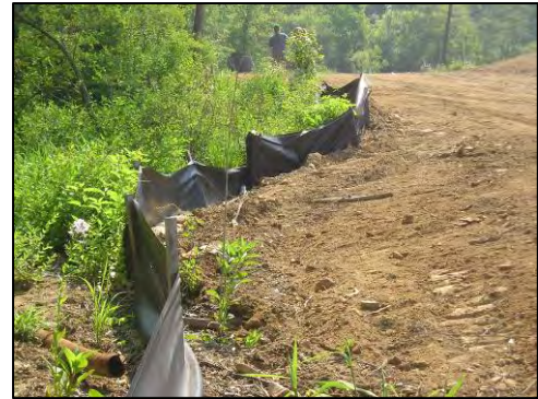
Siltation fences, as depicted in the photo, are a best management practice used to contain loose soil at construction sites
