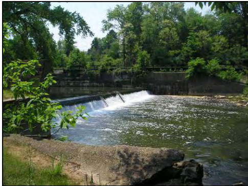
Porter's Cove Dam, one of several dams Wild Waterways Conservancy has proposed for removal reestablishing Connoquenessing Creeks natural flow
