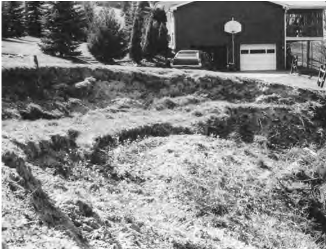
Figure 11. Slump failure and the steep scarp at the head above the disrupted ground. Photograph by R. P. Briggs.
