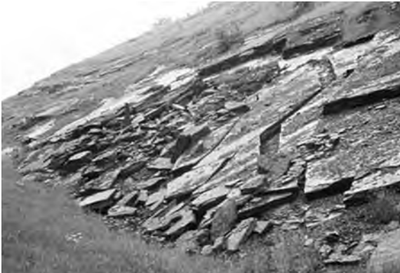
Figure 17. Sandstone bedrock in this highway cut dips steeply from right to left. Blocks in the top layer of rock have broken loose from the intact rock and are slowly sliding downslope along a bedding surface. A wide drop zone keeps the rock from sliding onto the highway.
