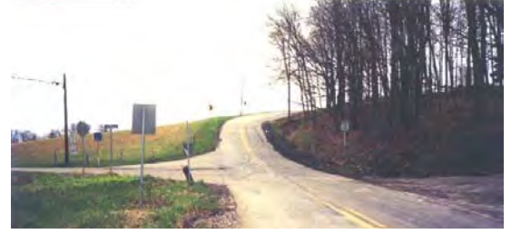
SR 3002/SR 3005 intersection looking east
