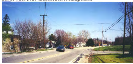
SR 857/SR 3029 intersection looking north
