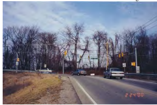
New Salem Road/Matthew Drive intersection looking north
