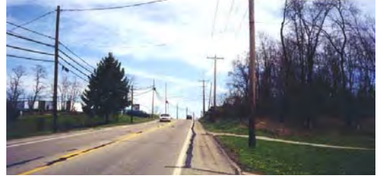
SR 119/SR 3010 intersection looking north
