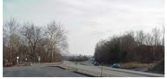
SR 51/SR 1043 intersection looking south
