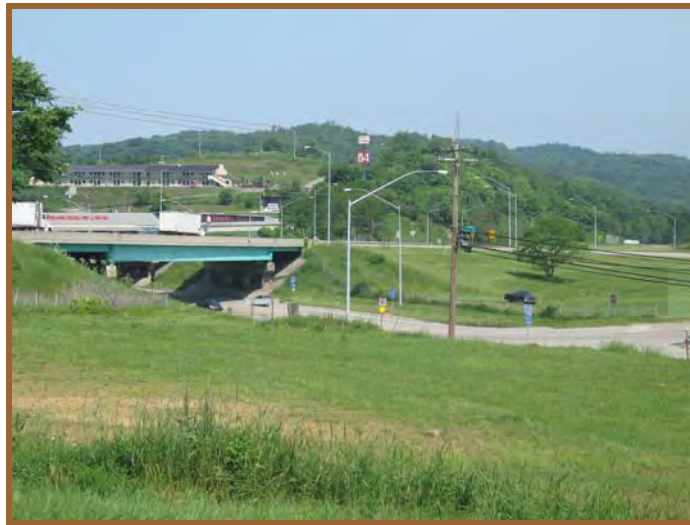
Waynesburg Interchange (Mackin, 2006)
