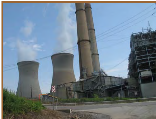
Hatfield Power Plant (Mackin, 2006)
