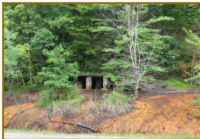
Abandoned Mine Drainage (Mackin, 2007)
