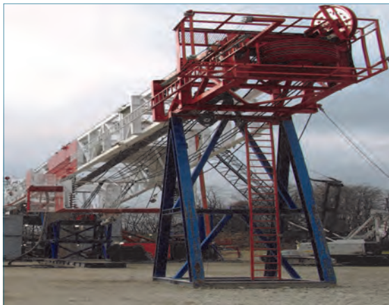
Figure 11.6: Marcellus Shale drilling operation, Butler County
