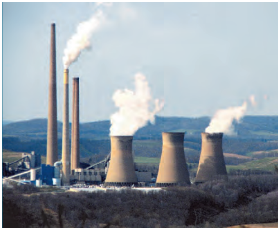
Figure 11.2: Homer City Generating Station, Center Township
