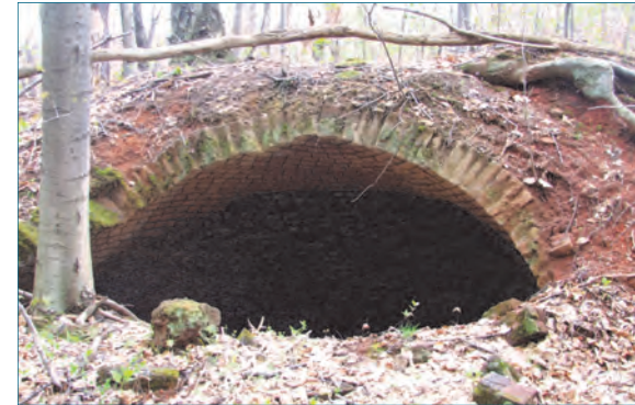
Figure 10.8: Graceton coke ovens, Center Township
