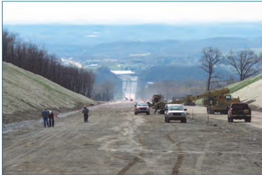
Figure 3.12: US Route 22 improvements, Burrell Township
