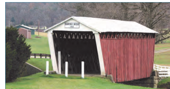
Figure 10.12: Harmon Bridge, Washington Township
