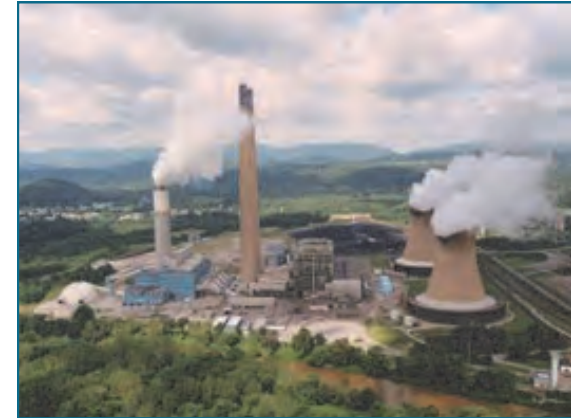
Figure 4.25: Conemaugh Generating Station, West Wheatfield Township (Source: www.genon.com)
