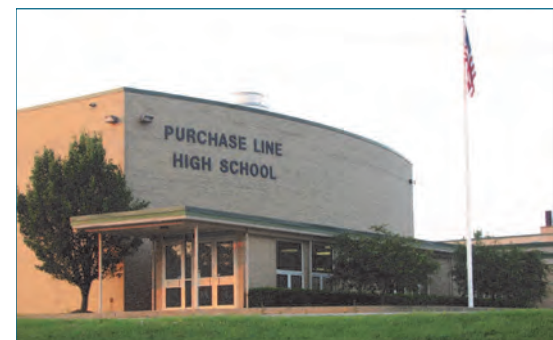
Figure 4.6: Purchase Line High School, Green Township
