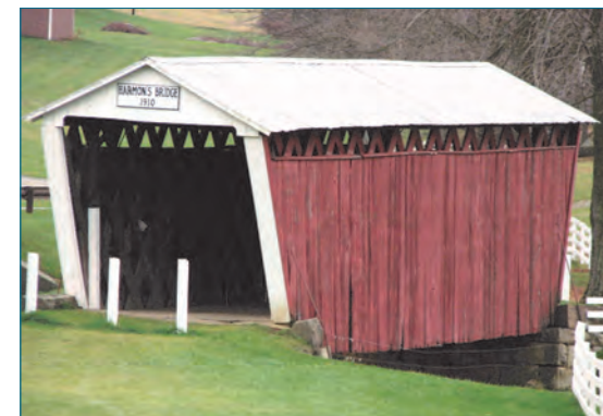
Figure 3.15: Harmon Bridge, Washington Township
