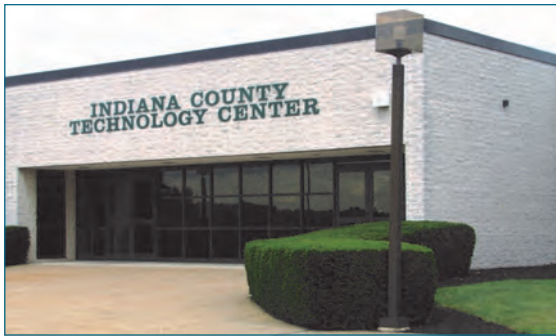
Figure 4.13: Indiana County Technology Center, White Township
