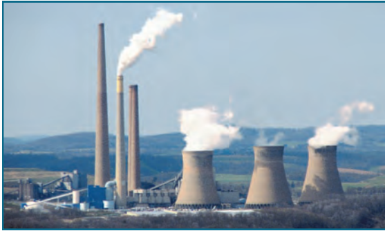
Figure 2.6: Homer City Generating Station, Center Township
