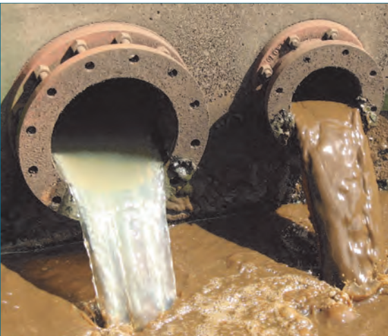
Figure 5.6: BMA oxidation ditch, Burrell Township
