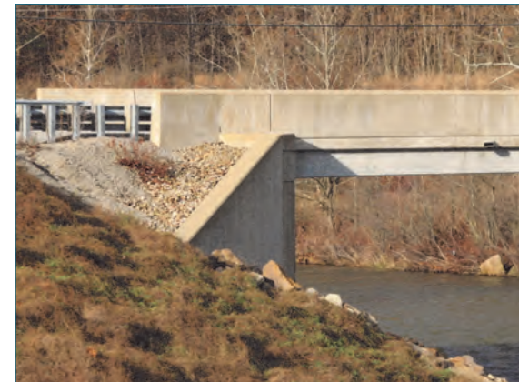
Figure 6.3: Josephine Bridge, Burrell Township
