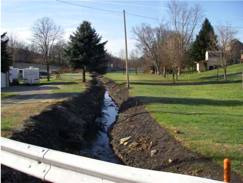
Photo 13: Stauffer Run - Alverton
