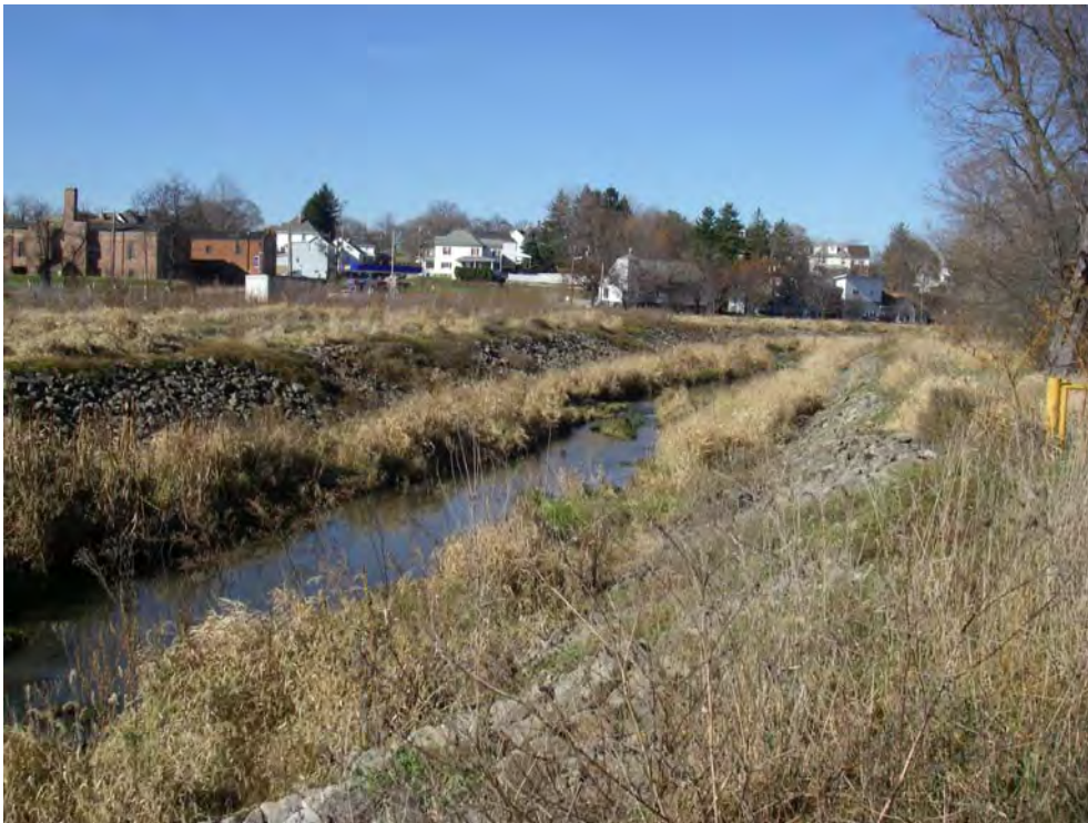
Photo 14: Stauffer Run - Scottsdale flood control project
