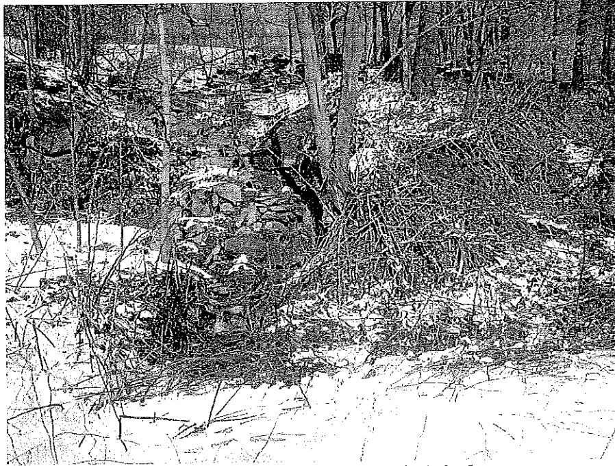
Figure 17. Picture of the Slick Hill Discharge.
