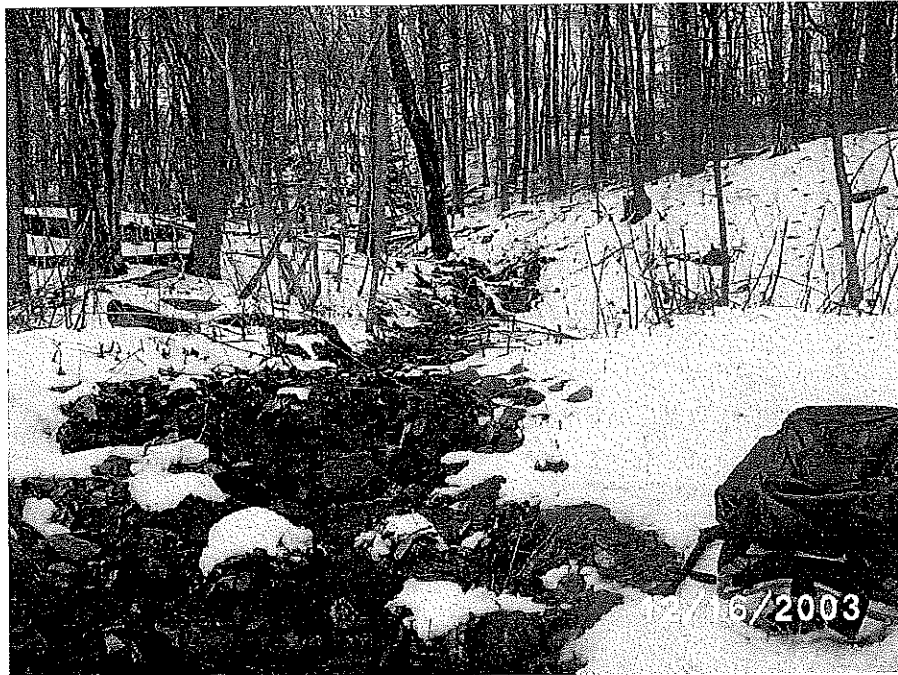
Figure 24. Picture of the Discharge Downstream of Trux.
