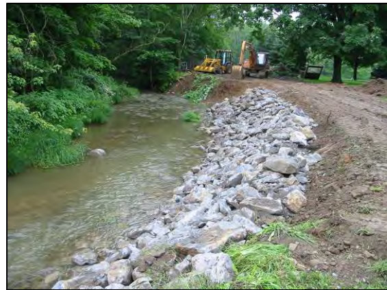
Streambank stabilization project at Falcon Park, construction phase, June 2003
