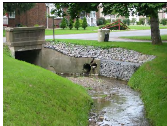
Streambank stabilization project on Tub Mill Run required as a result of excessive stormwater runoff
