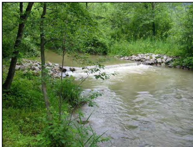
Stream habitat improvement project on Cherry Run
