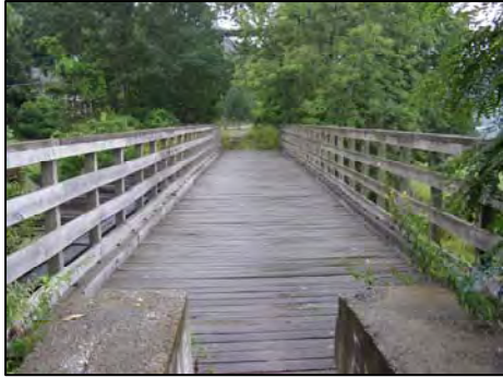
Armstrong Trail bridge over Mahoning Creek near Templeton, Pa.
