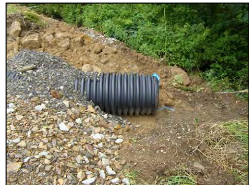
Newly installed culvert pipe under Mottarn road
