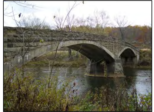
Madison-Mahoning Township Bridge located near Thayerton, PA
