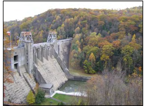
Mahoning Creek dam located 21.6 miles upstream from the Allegheny River
