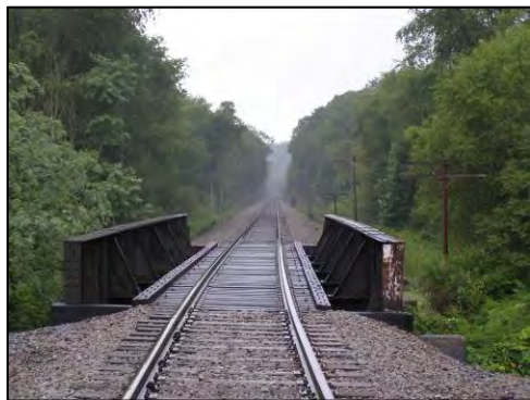
Railroad bridge over South Fork Pine Creek near Echo, PA
