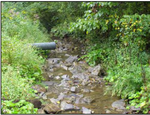
Stormwater pipe that enters into Hays Run
