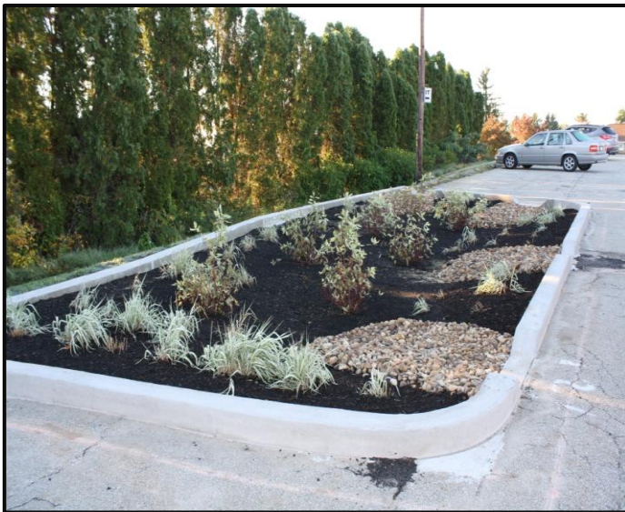
Figure 9: A rain garden in a parking lot to capture stormwater from an impervious parking lot (Source: Westmoreland Conservation District)
