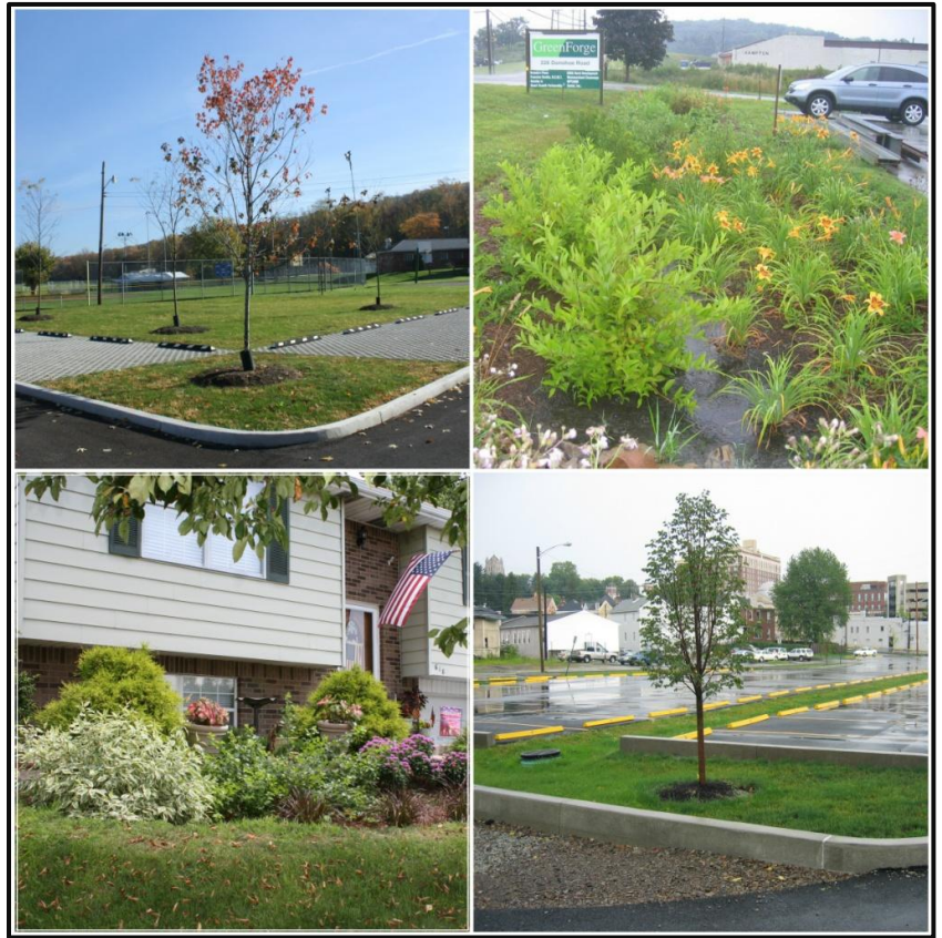
Figure 12: Local examples of Structural BMPs. Derry Borough parking with porous pavers (top left), a rain garden at Green Forge (top right), a residential rain garden (bottom left), and an adjustment to a parking lot in Greensburg. (Source: Westmoreland Conservation District)
