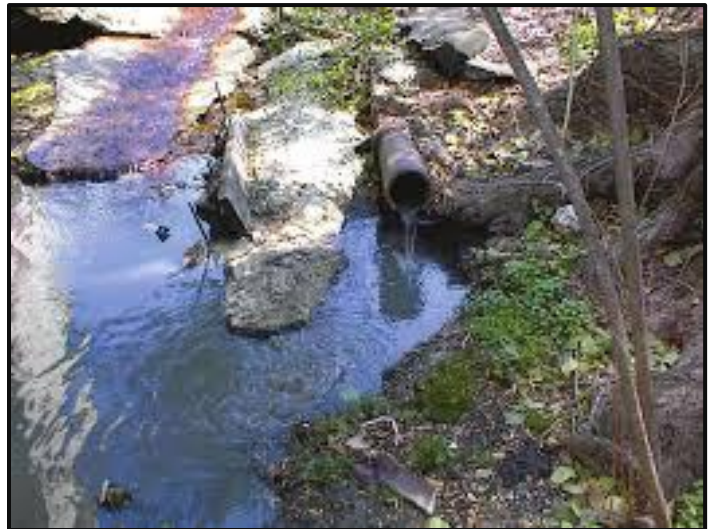
Figure 5: Illicit discharge (Source: EPA IDDE Manual: https://www3.epa.gov/npdes/pubs/idde_manualwithappendices.pdf )
