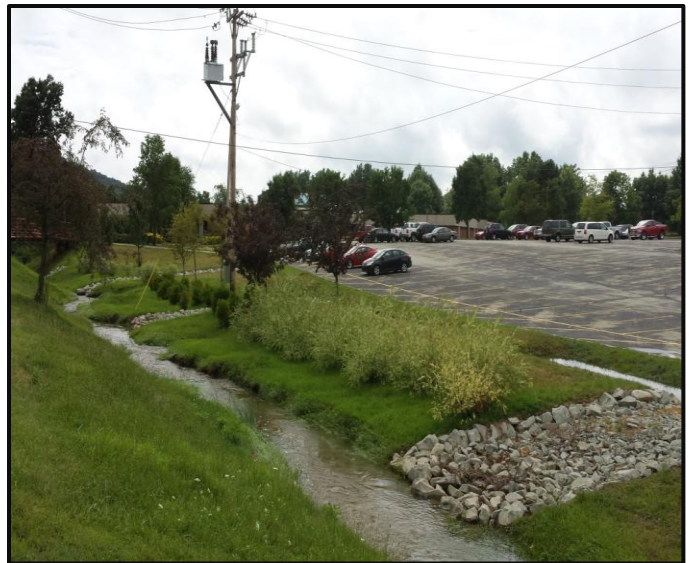
Figure 10: Infiltration swale at Westmoreland County Community College
