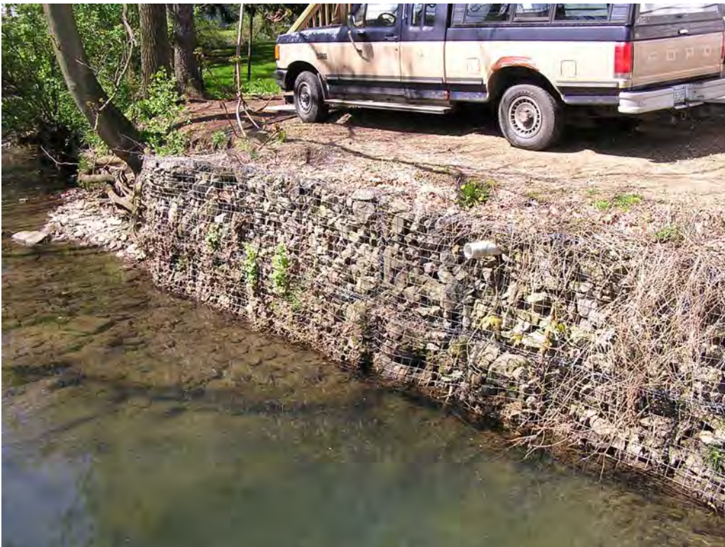
Figure 3-4: Stream Bank Stabilization in the Marsh Run Watershed
