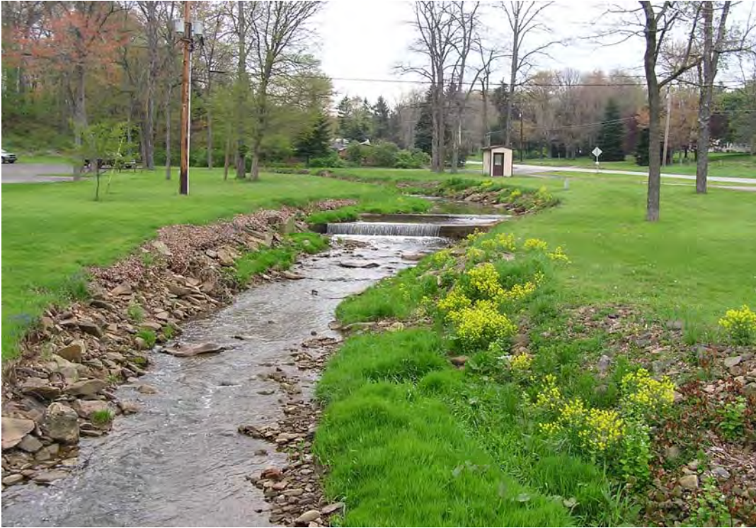
Figure 3-7: Channel Modification and Stream Bank Stabilization on the McCarthy Run Mainstem
