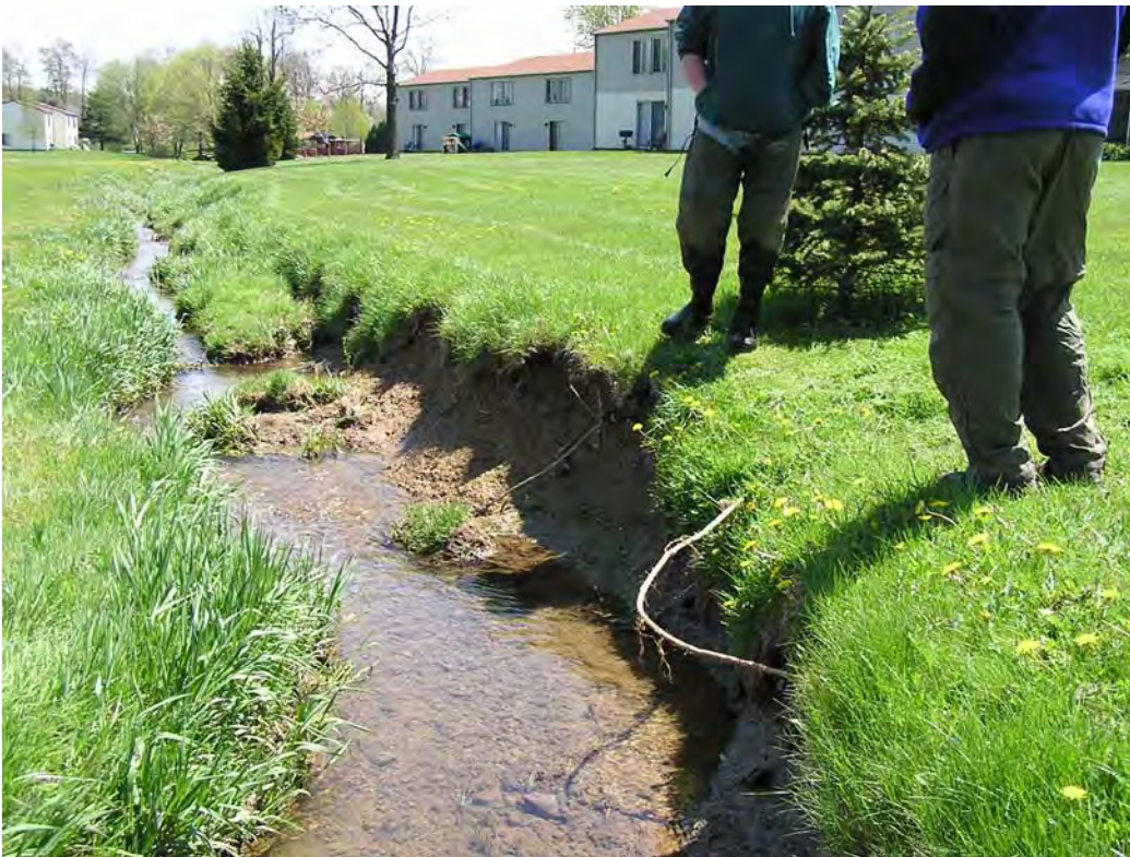
Figure 3-6: Stream Bank Erosion in the Headwaters of McCarthy Run
