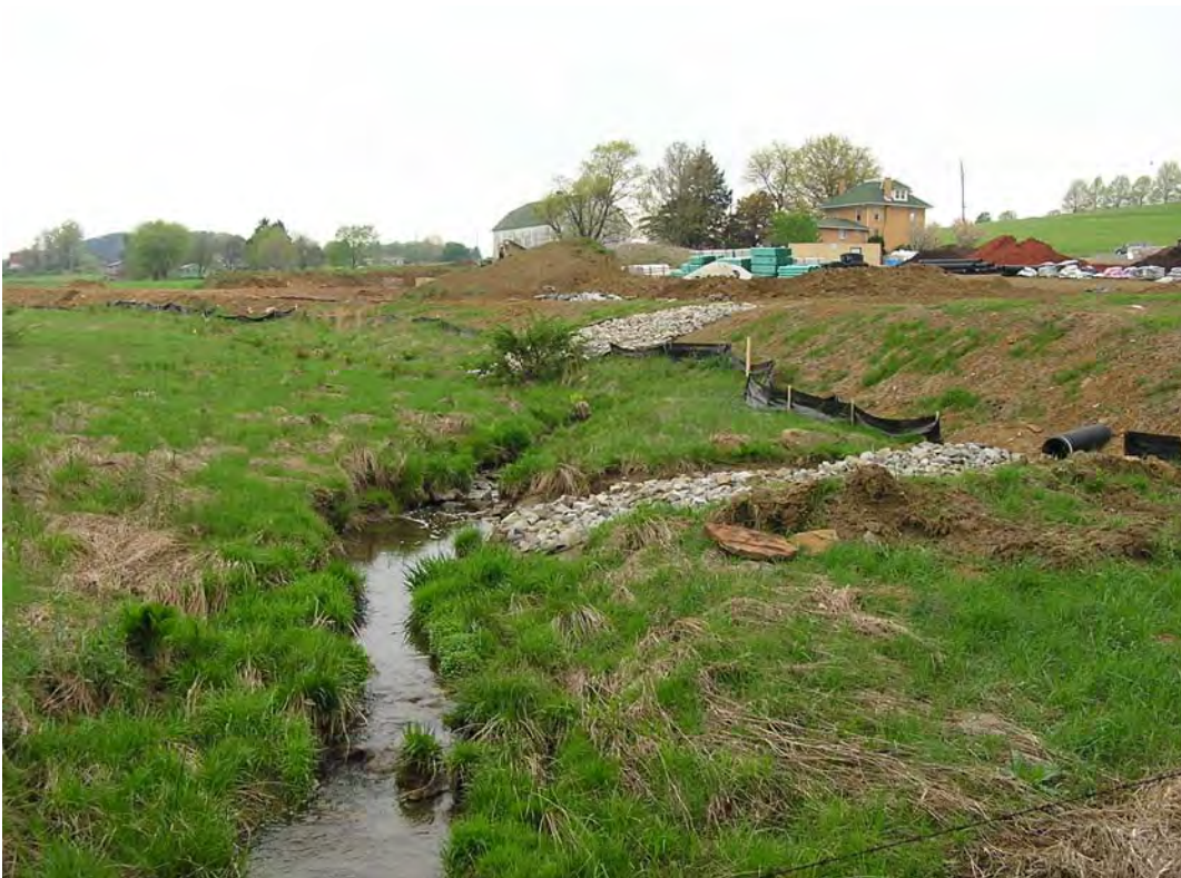
Figure 3-8: Bank Erosion and Exposed Soil in the McCarthy Run Watershed
