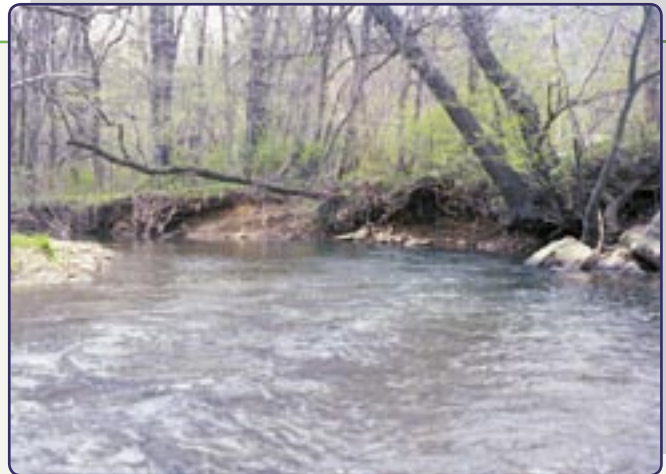
Bank erosion in the Mallard Lane area.
