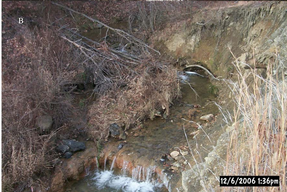
Figures 3A & 3B. Areas of streambank erosion and stream bottom sedimentation that will be restored via reclamation of original stream channel, surface contouring, and revegetation. ultimately arrive at downstream TMDL point NB15 via increased rates of geochemical cycling kinetics. However, the post-project loading from the site to the unnamed tributary to the North
