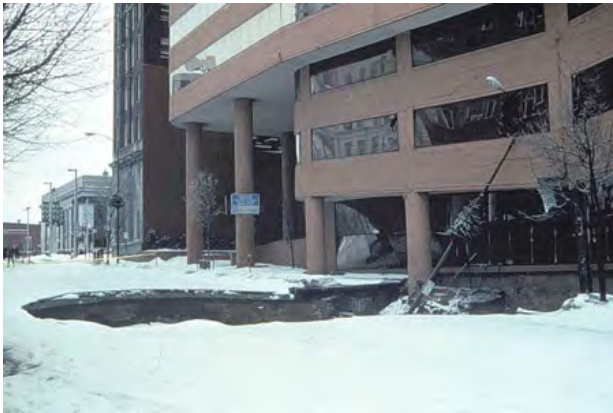
Sinkhole at Corporate Plaza Building in Allentown, Lehigh County, PA in February, 1994 (Photograph by William E. Kochanov . PA DCNR, 2009).
