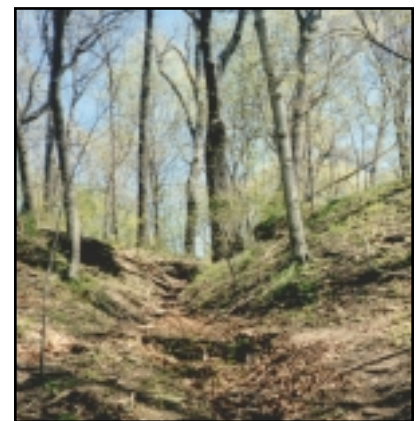
Erosion occurs throughout the Park and is due to the geology, soils and the intensive use.
