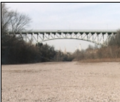
Construction is currently underway for new athletic facilities within Junction Hollow.
