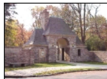
Restored gatehouses at the Reynolds Street entry to Frick Park - just one of the pilot projects undertaken by the Pittsburgh Parks Conservancy
