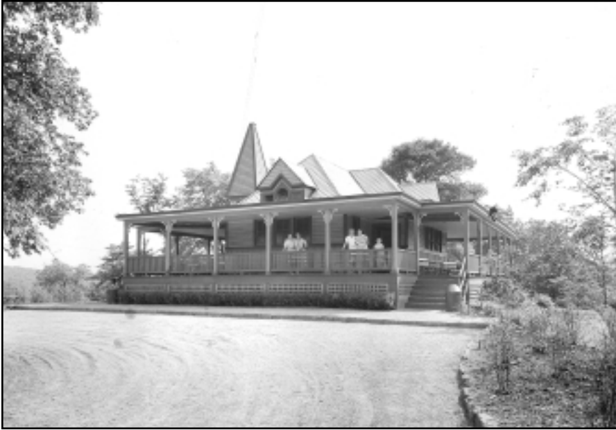
The Chapel was once a beautifully ornate structure. Sadly, much of this detail has been lost. Restoration should include the structure as well as the surrounding landscape.
