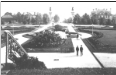
Restoration of the Entry Gardens in Highland Park
