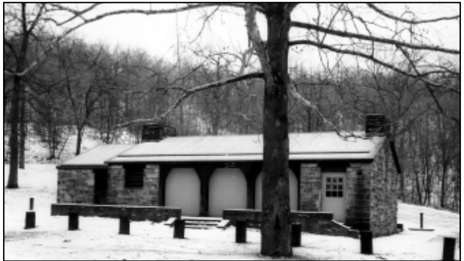
Valley Refuge shelter should be rehabilitated.
