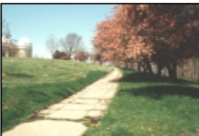
The walkways and landscaping around the Observatory have deteriorated and should be restored.
