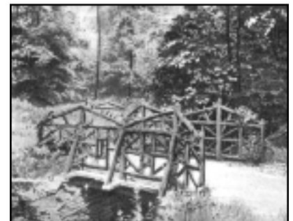
The pedestrian infrastructure has undergone many changes over the years - these rustic wooden bridges were replaced with the stone bridges that still exist today.
