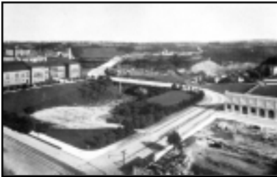
Prior to constructing Schenley Plaza, the entrance road wound past Forbes Field (under construction on the right) and over the Bellefield Bridge that spanned St. Pierre Ravine. The bridge was buried when the ravine was filled in.
