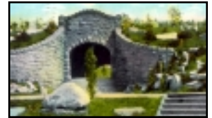
The pedestrian underpass in Highland Park typifies the rugged craftsmanship of features in the parks
