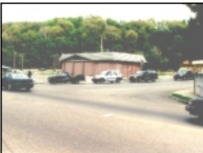
A new gas station (to replace this one) at the corner of Butler Street, is currently under construction. The character should be compatible with the rest of Highland Park and the Pittsburgh Zoo.
