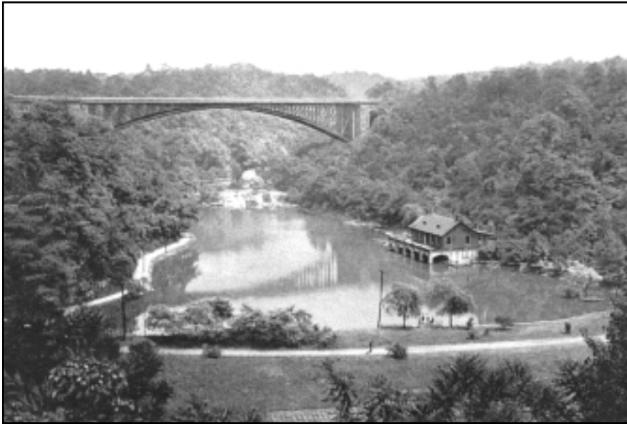
Historic view of Panther Hollow Lake. The Lake supported many activities, including boating. The former boat house is the structure to the right.
