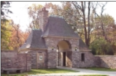
Restored Reynolds Street Gatehouse in Frick Park
