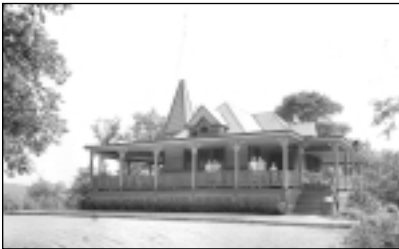
Restoration of the Chapel Pavilion and surrounding landscape in Riverview Park
