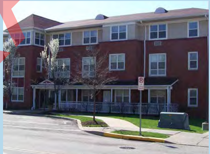
OAK HILL APARTMENTS Source: Graves Design Group
