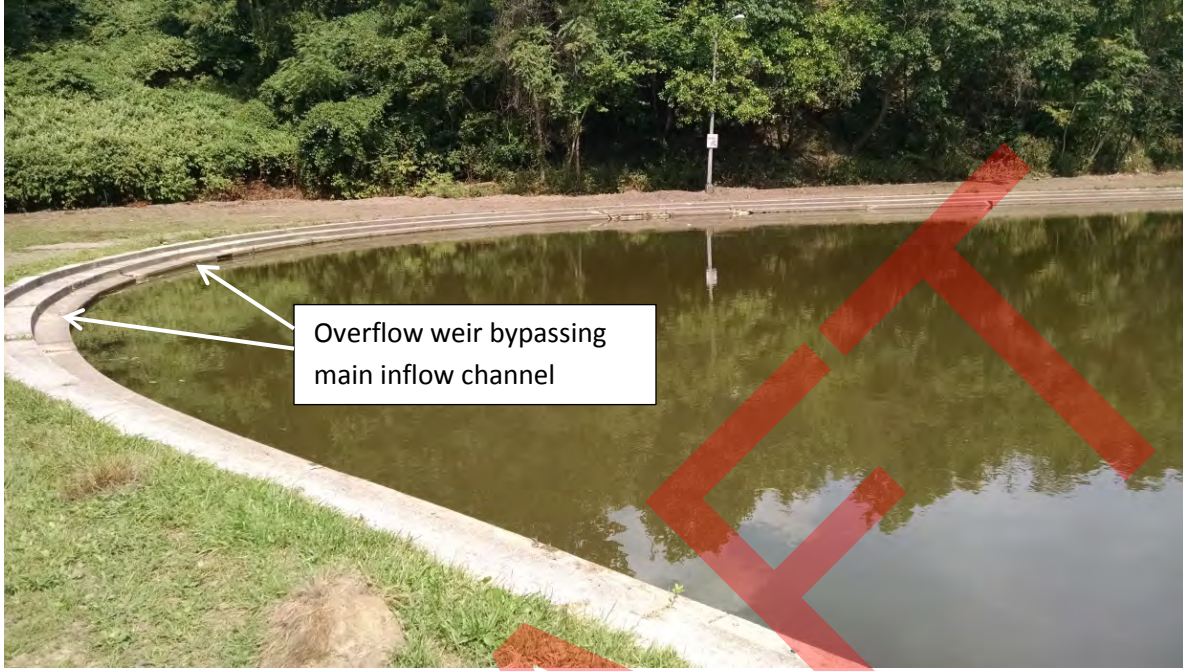
Figure 5-15: Panther Hollow Lake Overflow Weirs Diverting Water to the Lake Overflow Pipe
