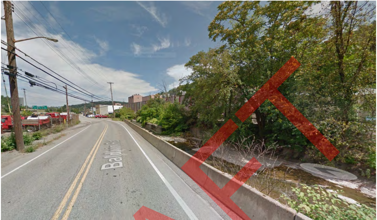
Figure 4-6: Streets Run Just Upstream of the GalvTech Building
