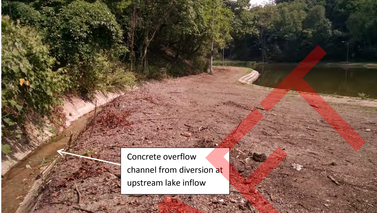
Figure 5-14: Overflow Channel Downstream of the Stream Inflow Diversion at Panther Hollow Lake
