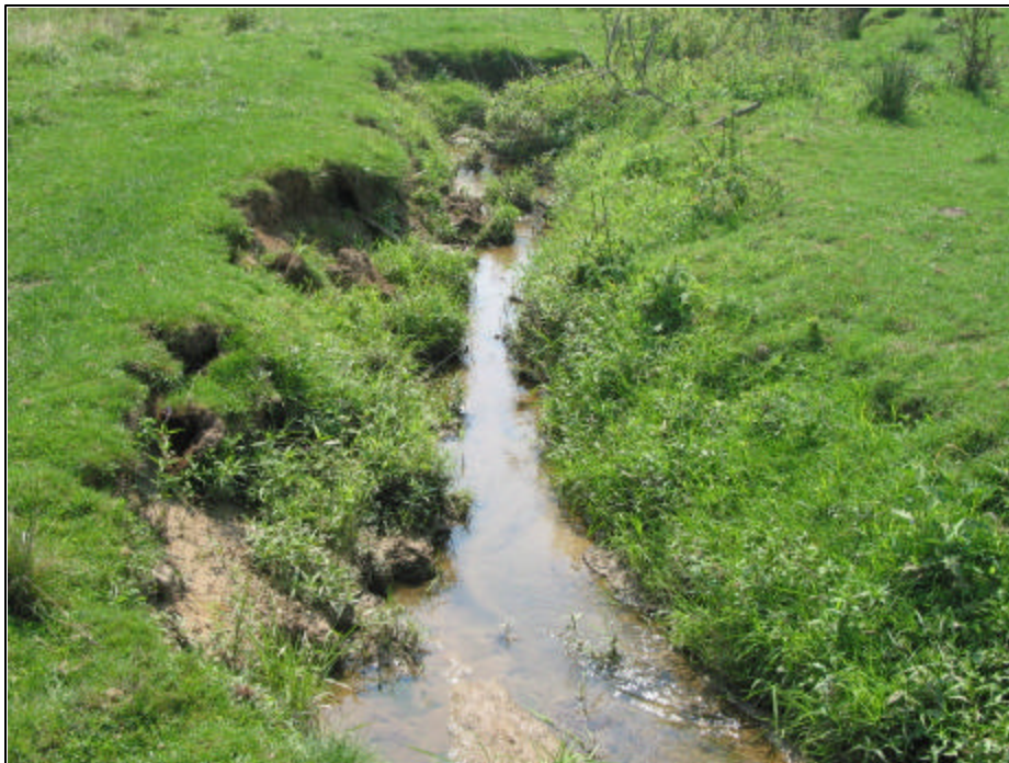
Figure 7. Decaying streambank of Patterson Creek (Armstrong County).
