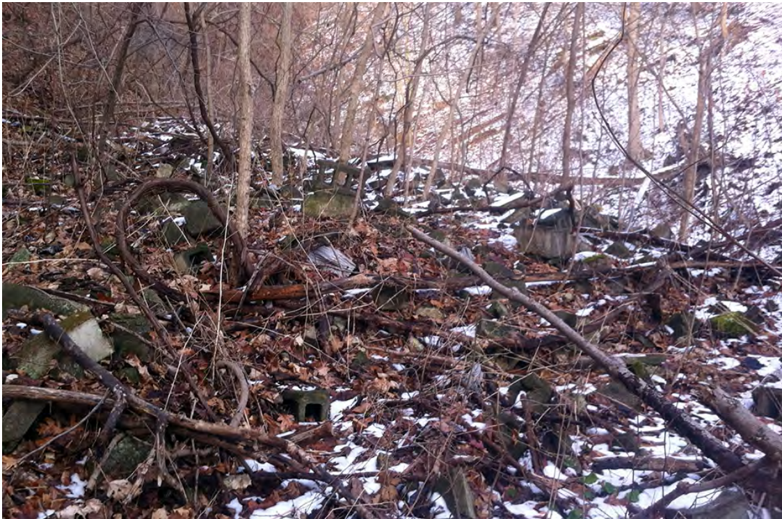
PCLT06 - Just upstream of the erosion gully is a large construction debris dump on the left ascending floodplain.
