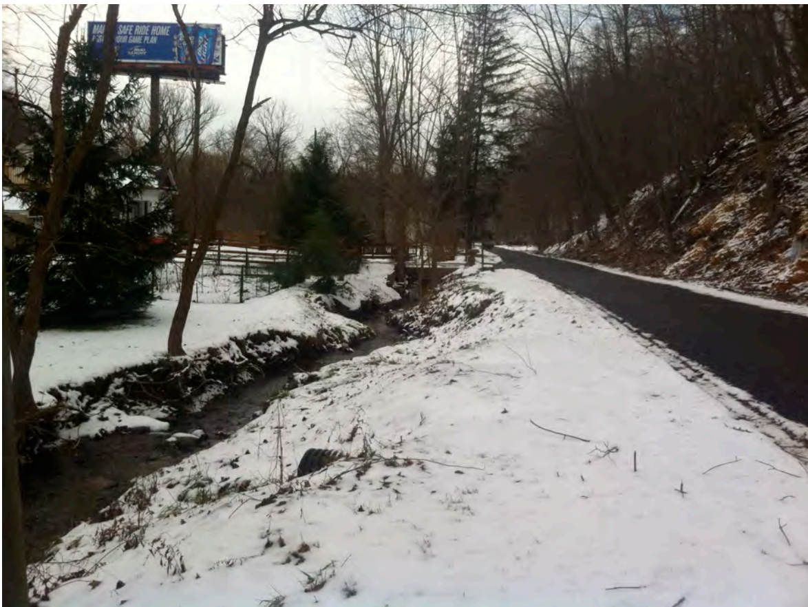
SCR13 - Scotia Run along McGrew Rd. Storm water from drainage channel on opposite side of road enters Scotia Run in foreground. Scotia Run is culverted under private driveway and pedestrian bridge in middle of photo. Large billboard along Rt51 in upper left. Looks like homeowner has built levee along stream in front of house.
