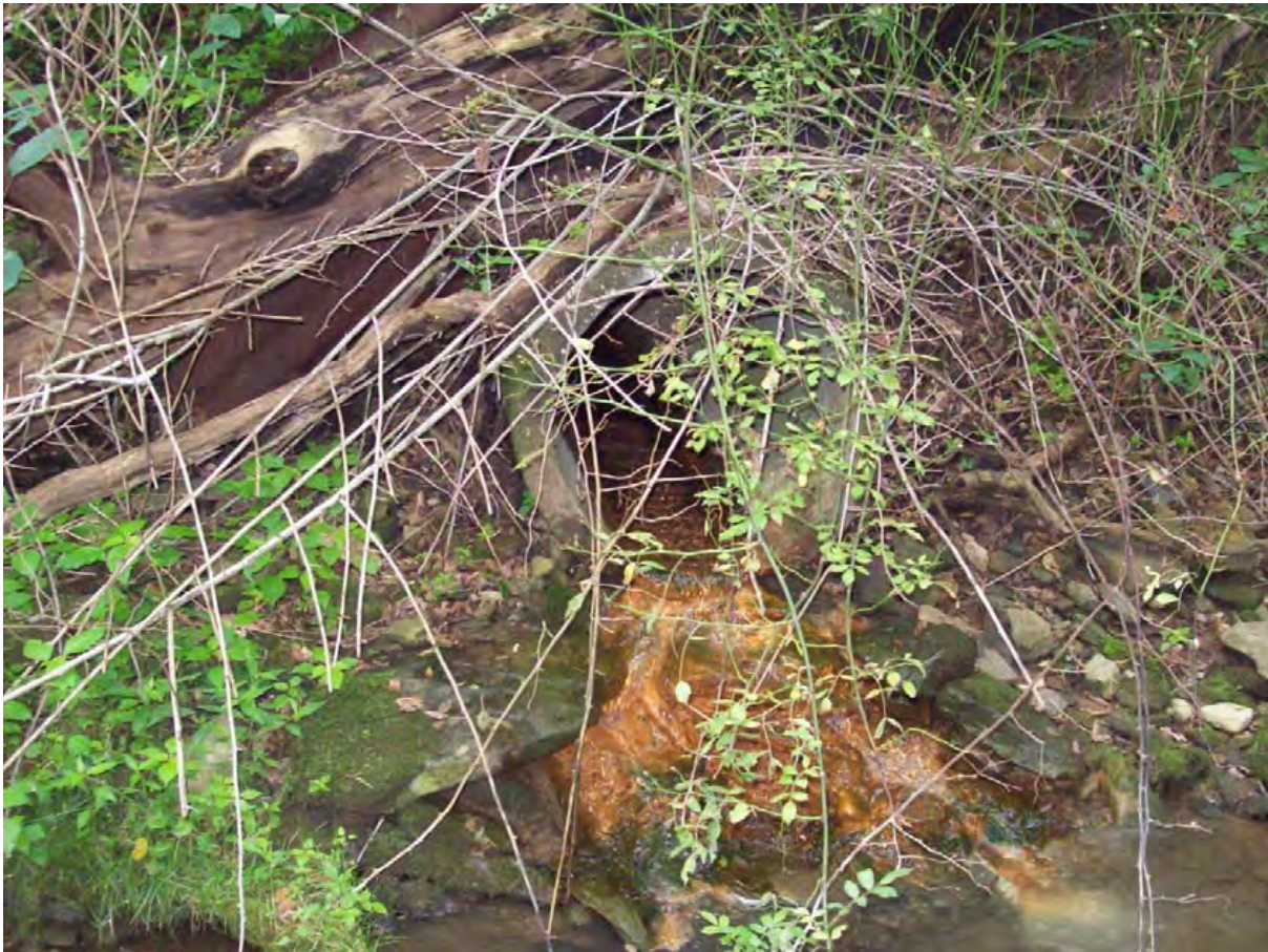
TFT05 – Culverted AMD discharge to Trax Farm Tributary in the lower reach of the stream.
