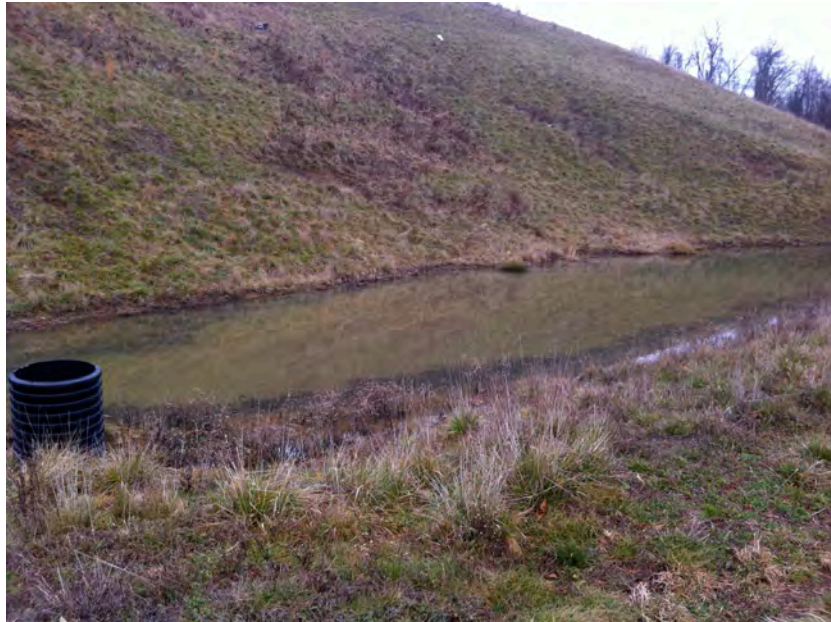
MRT07 – A stormwater detention basin that is part of the Hunter's Fields development along West Bruceton Road and Mineral Run in Jefferson Hills.
