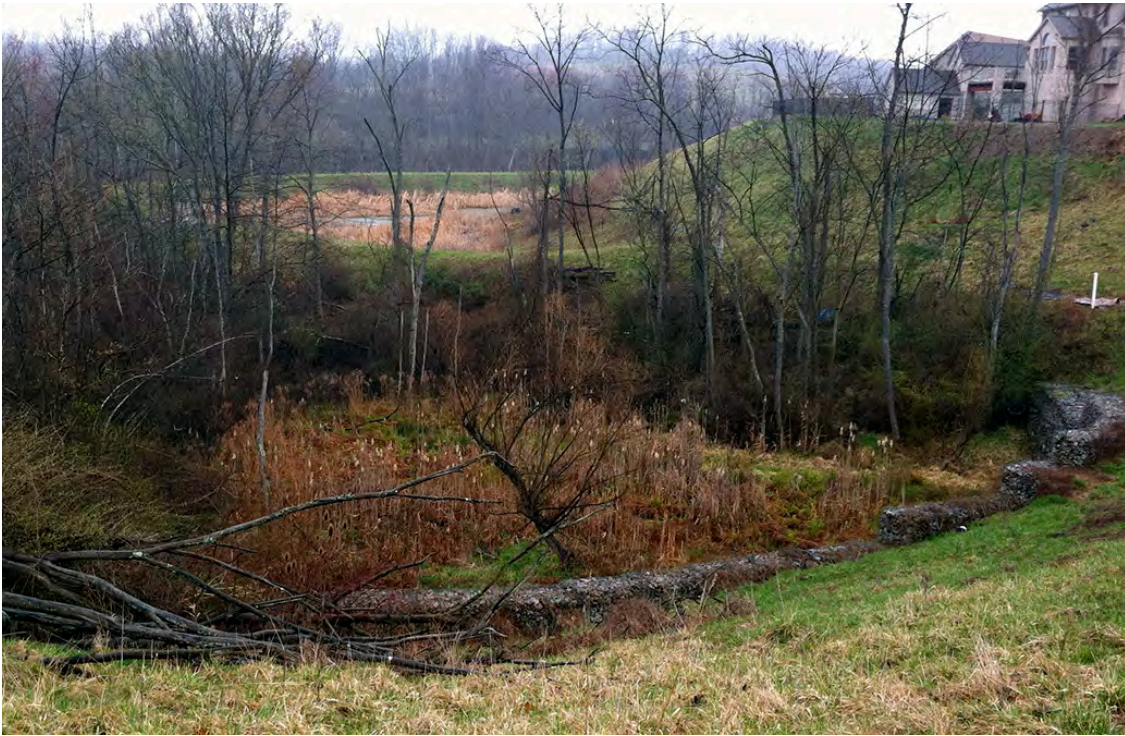
MRT17/MRT16 – An AMD discharge flows from under the gabion rip-rapped retaining wall and enters a wetland just west of Thomas Jefferson Dr and Jefferson Estates. In background is a stormwater detention basin that is impacted by AMD.
