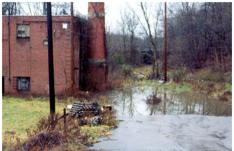
CR26 - Remnants of a nonfunctional bridge crossing of Catfish Run behind the fairgrounds buildings encroaches on the stream channel and is constantly creating debris jams that flood the surrounding area during heavy precipitation. Schoonmaker Hall and a sanitary sewer manhole also encroach on Catfish Run just upstream of this location.
