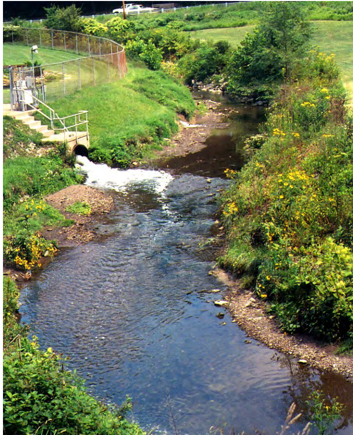
LR30/LR31 – Pleasant Hills Authority Sewage Treatment Plant outfall into Lick Run just upstream of Wallace Rd bridge. Further upstream a smaller outfall from the sewage plant can be seen entering Lick Run's left ascending bank.
