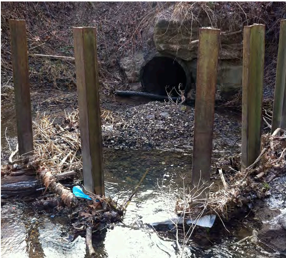
A debris jam within Lick Run along Cochran Mill Road has formed behind a sewer manhole within the stream channel. This is a common occurrence, compromises sewer infrastructure and often leads to raw sewage within the stream. The debris jam is comprised of assorted debris including litter and construction material.
