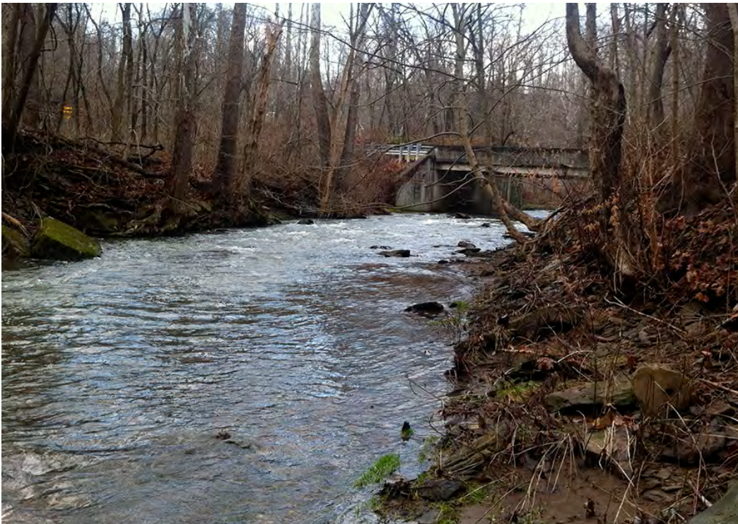
PF15 - Piney Fork passes under a bridge at the end of an entrenched meander along Piney Fork Rd near PennMont. PennMont was the interchange of the Pennsylvania Railroad and the Montour Railroad. Just upstream of the bridge are abutment remnants of a railroad crossing of the stream. Another bridge crossing of Piney Fork is located a few hundred feet upstream near the head of the meander.
