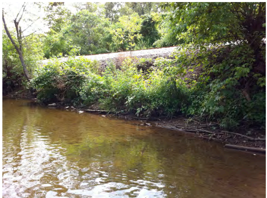
PCM07 – Wheeling & Lake Erie Railroad tracks alter the left ascending bank floodplain and limit vegetative growth in the riparian zone at many locations along the southern side of Peters Creek as seen here in the eastern portion of the Middle sub-watershed.
