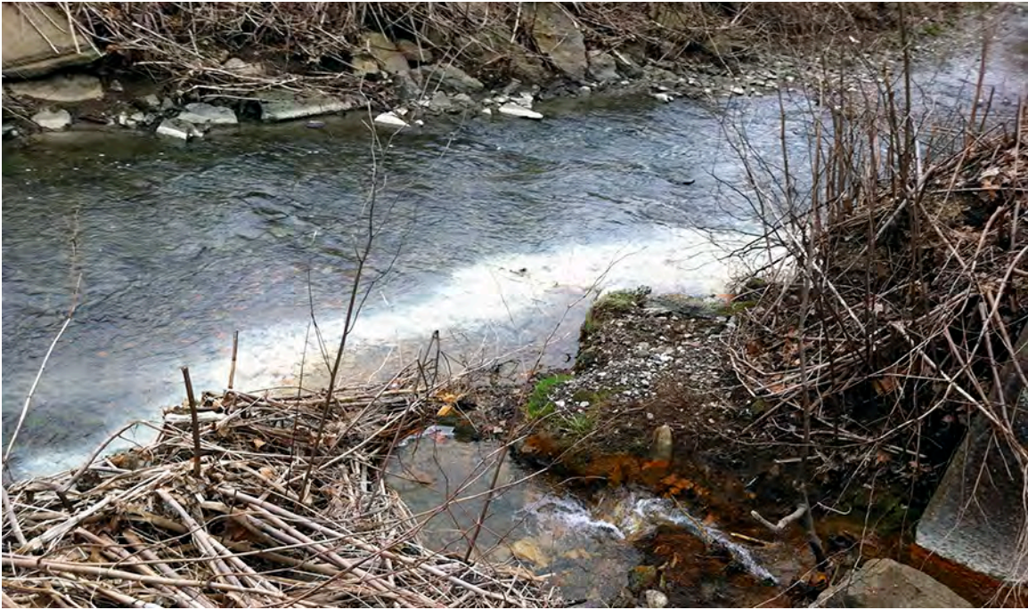
LR16 – AMD impacted tributary draining valley along Riggs Rd enters Lick Run's left ascending bank after being culverted under the Cochran Mill Rd tunnel. Severe erosion problems on the streams right ascending bank along the road from Snowden Rd junction to tunnel.
