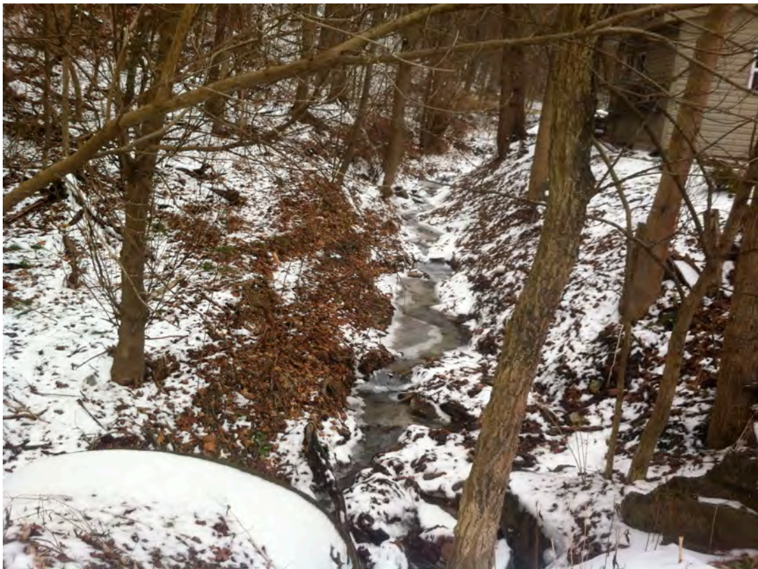
SCR07 – Tributary draining wooded valley to east of McGrew Rd is culverted under the road and under the back edge of Bowers lot. The tributary enters Scotia Run while it is culverted under the lot. The upper reaches of this tributary have been surface mined. This may contribute to the high conductivity levels of Scotia Run.
