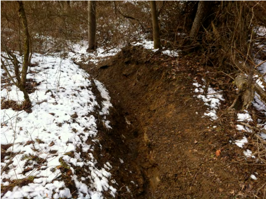
BR09 – An off-road trail on Beam Run's steep right ascending bank creates an erosion gully.
