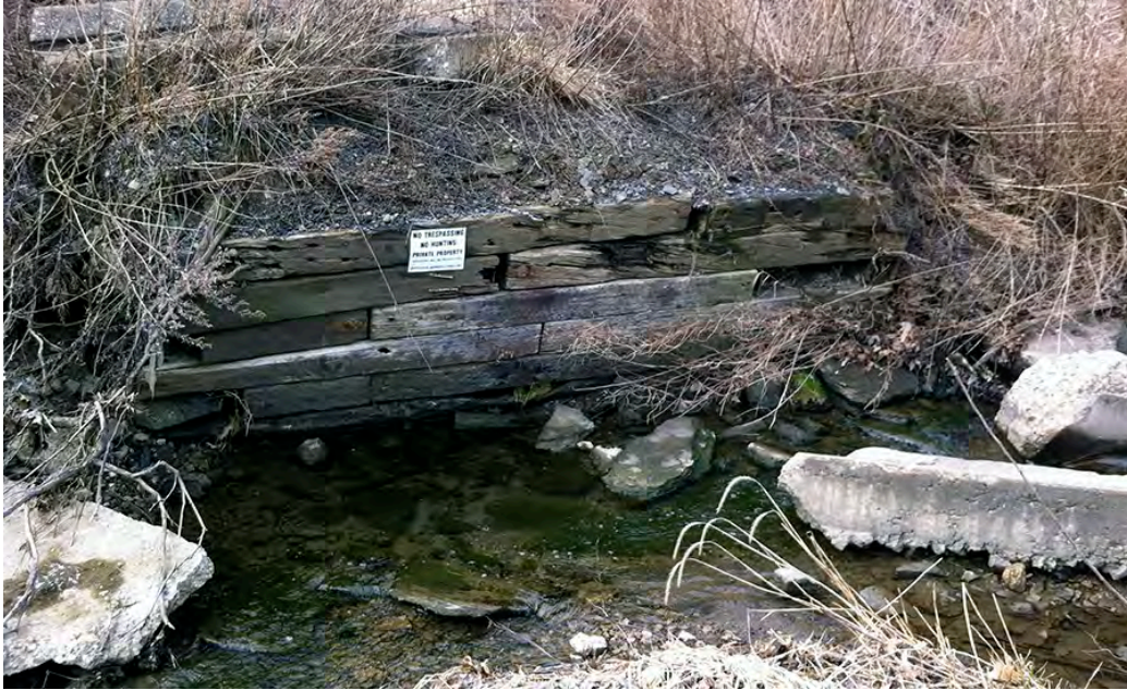
JMT05 – A number of issues are illustrated in this photo taken along the lower reach of the Jefferson Memorial Tributary. An overabundance of algal growth is evident as is encroachment from an old railroad tie wall along the streams left ascending bank, construction debris within the floodplain and concrete debris obstructing the stream channel.
