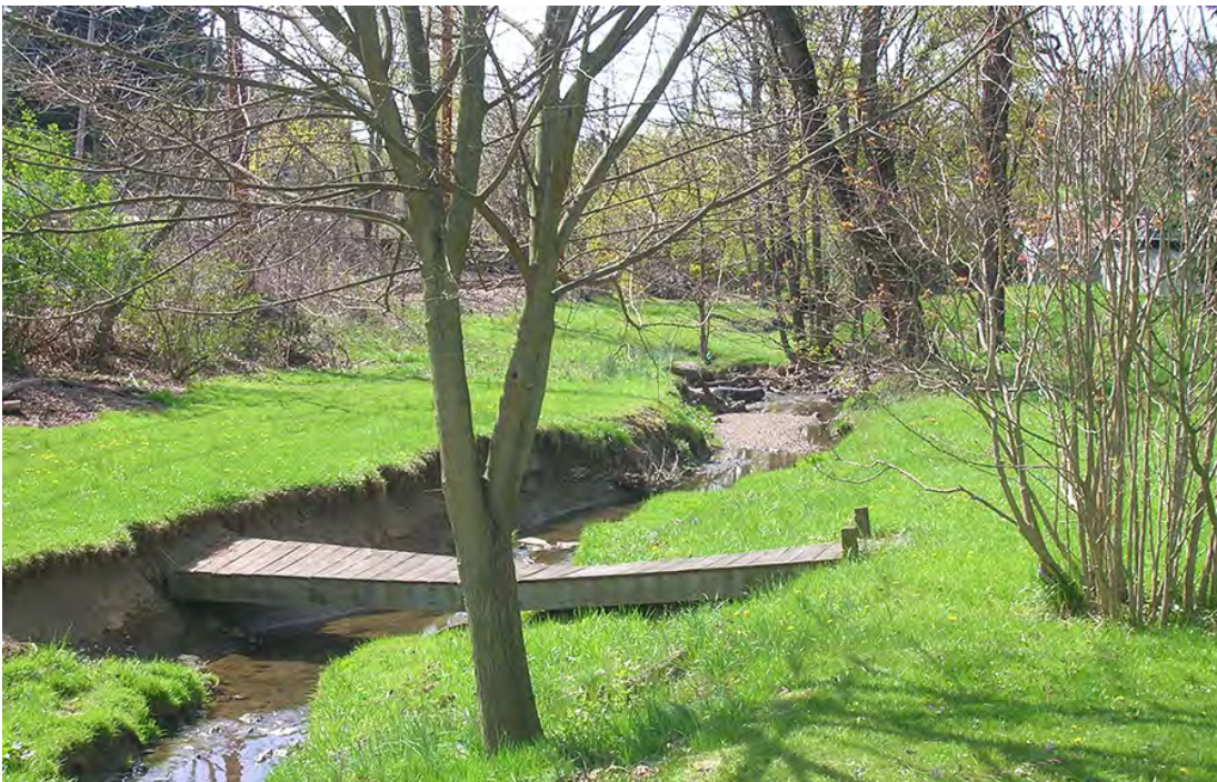
BRB26 – The Brightwood Road branch of Piney Fork is first daylighted just south of South Park Road. The stream appears to be culverted under a heavily developed older section of Bethel Park north of South Park Road and takes on great quantities of excess stormwater during precipitation events. The upper reaches of the daylighted stream are deeply incised and eroded. The stream continues to be impacted far downstream.
