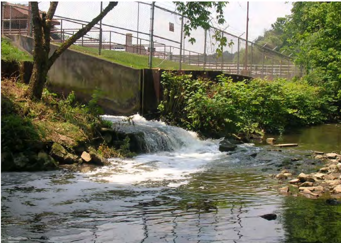
PF40 –The Piney Fork Wastewater Treatment Plant outfall into Piney Fork just downstream of Catfish Run's confluence with Piney Fork. The sewage treatment plant serves approximately two-thirds of Bethel Park and a portion of South Park Township. A small portion of Peters Township has also expressed interest in utilizing the facility.
