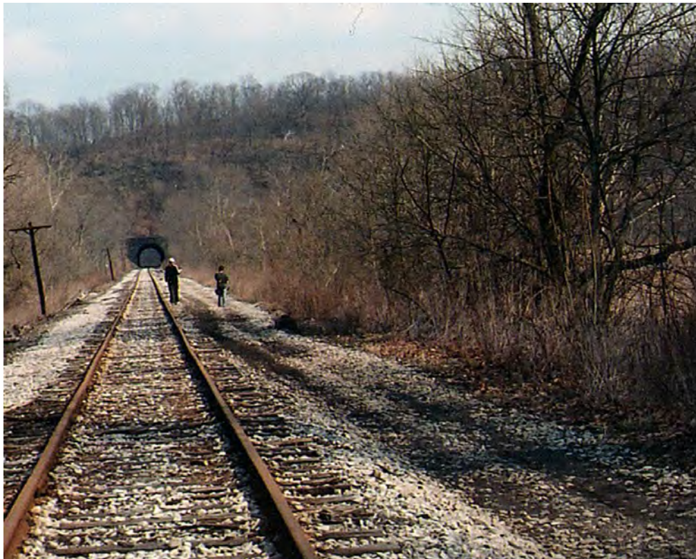
PCL26 – Looking east toward the western portal of the Ravensburg Tunnel from along the Wheeling & Lake Erie Clairton Branch tracks. Peters Creek flows along the tracks to the left and the Ravensburg Wetland is in the valley to the right of the tracks
