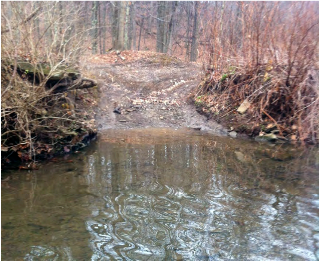
PF05 – One of numerous off-road stream crossings of Piney Fork just upstream of Corvette tunnel. These severe bank alterations are a conduit for stormwater and lead to excess siltation and increased erosion of the banks of Piney Fork. They also contribute to alteration of flow patterns within the stream channel.
