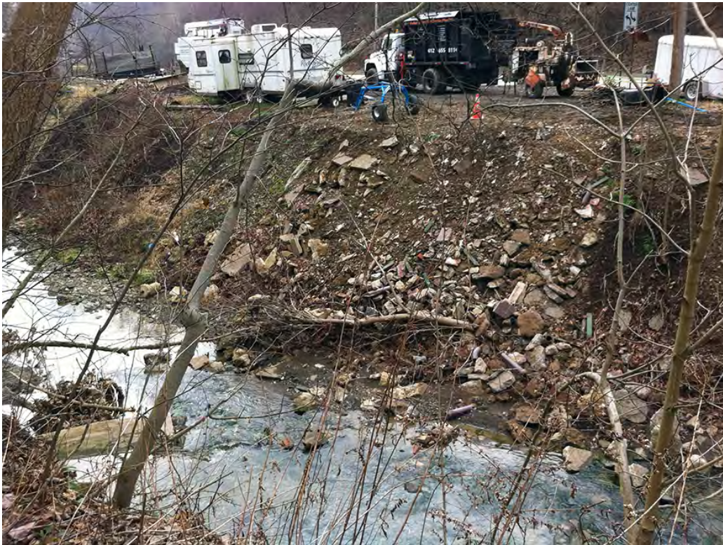
LW24 – Illegal dumping of construction material and other debris into Lewis Run from a landscape yard along Rt51.
