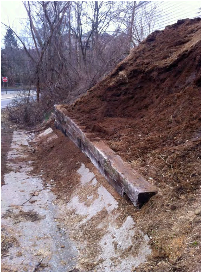
SH58 - Horse manure storage pile along McConkey Road. During rain events manure is washed into catch basin, across Stoltz Rd and into Sleepy Hollow Run.
