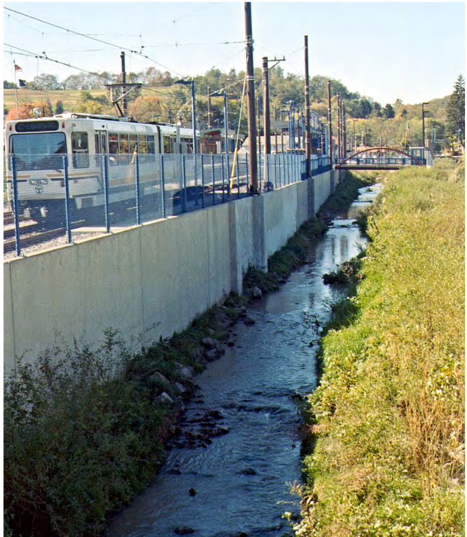
PF71 – Piney Fork, seen here channelized along the Library T-station, flooded on July 10, 2013 and inundated the station and adjacent Park & Ride Lot with 2-3 feet of water during a severe precipitation event. The infrastructure along the lower section of Piney Fork near Greenman Tunnel also incurred flood damage as a result of the storm. Piney Fork's channel was also significantly altered in this section by the flood.
