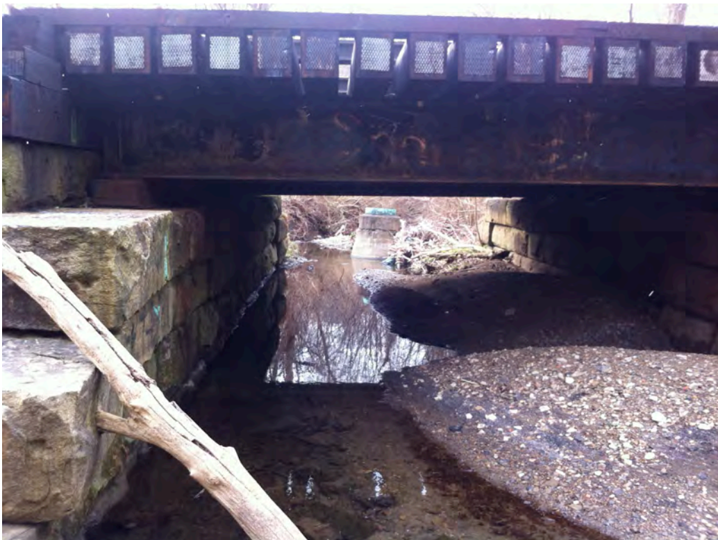
JMT10 - A sanitary sewer manhole within the channel of the Jefferson Memorial Tributary along Allegheny Valley Railroad tracks.
