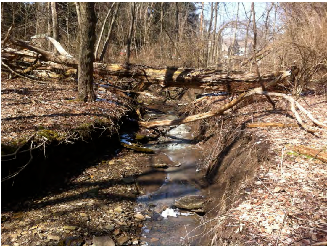
BR58 – White AMD precipitate evident on substrate of the main stem of Beam Run just downstream of the confluence of the Wakefield Road Tributary. The stream channel is deeply incised and the stream banks are eroded.
