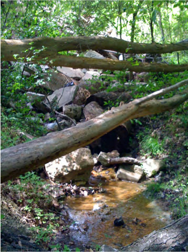
LR11 – Landowner along Snowden Road is pushing concrete construction debris into a tributary to Lick Run. The tributary also is impacted by abandoned mine drainage.
