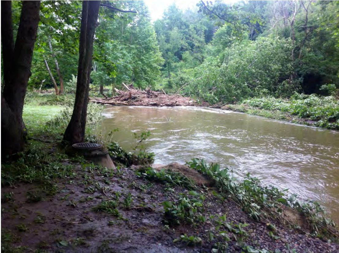
PCL23 – Debris jam deposited by floodwaters in July of 2013 dams Peters Creek below Natural Stream Channel Design Project.
