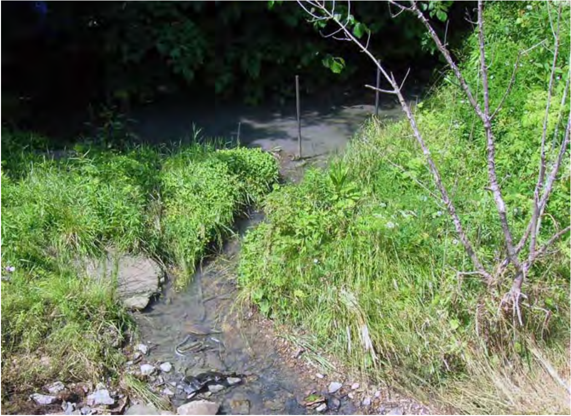
LR28 - A culverted AMD impacted discharge ponds along the Allegheny Valley Railroad tracks just downstream of Wallace Rd prior to entering Lick Run's left ascending bank.
