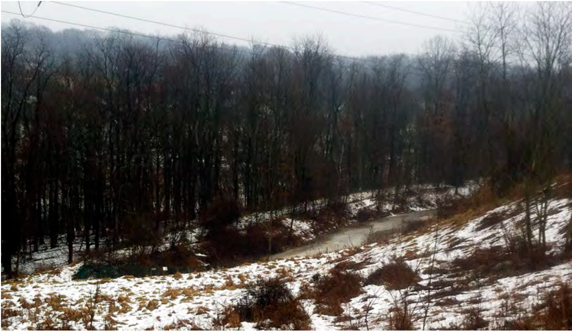
CR64 – A view of the stormwater detention basin associated with the Parkford Apartments off of Brownsville Rd. Catfish Run flows at the bottom of the steep wooded hillside behind the detention basin.
