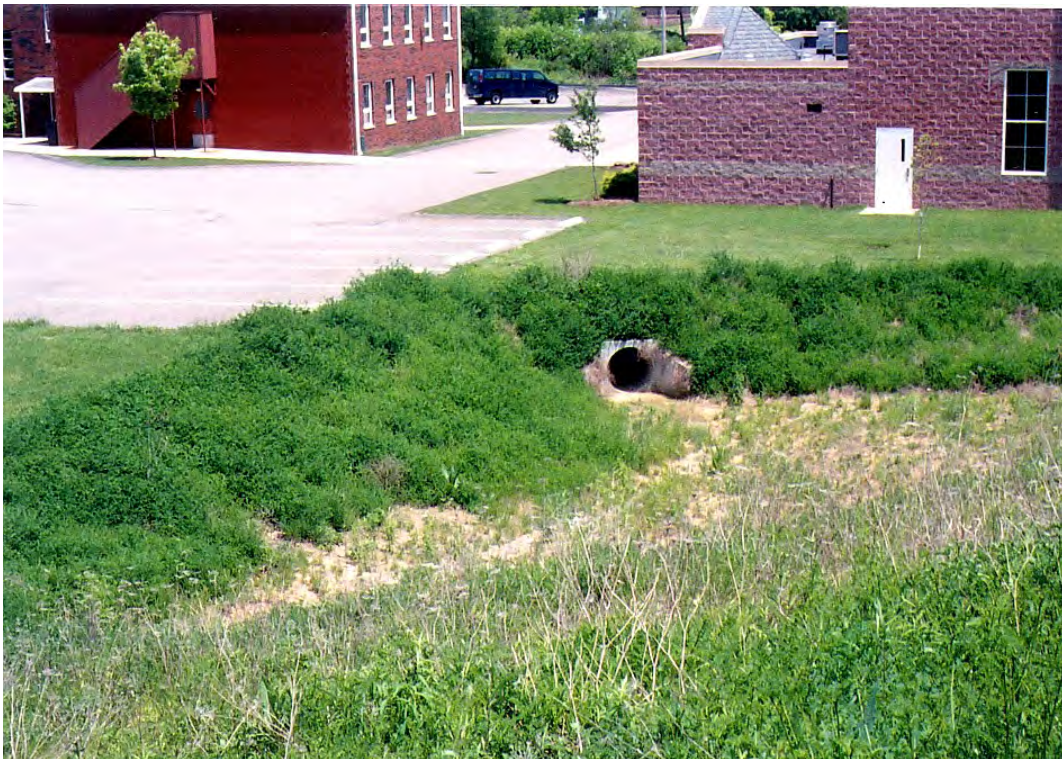
PCU146 – Stormwater runoff from Thomas Field and surrounding parkland along Linden Rd in Nottingham Township is culverted under a church lot and enters the extreme headwaters of Peters Creek's west branch.
