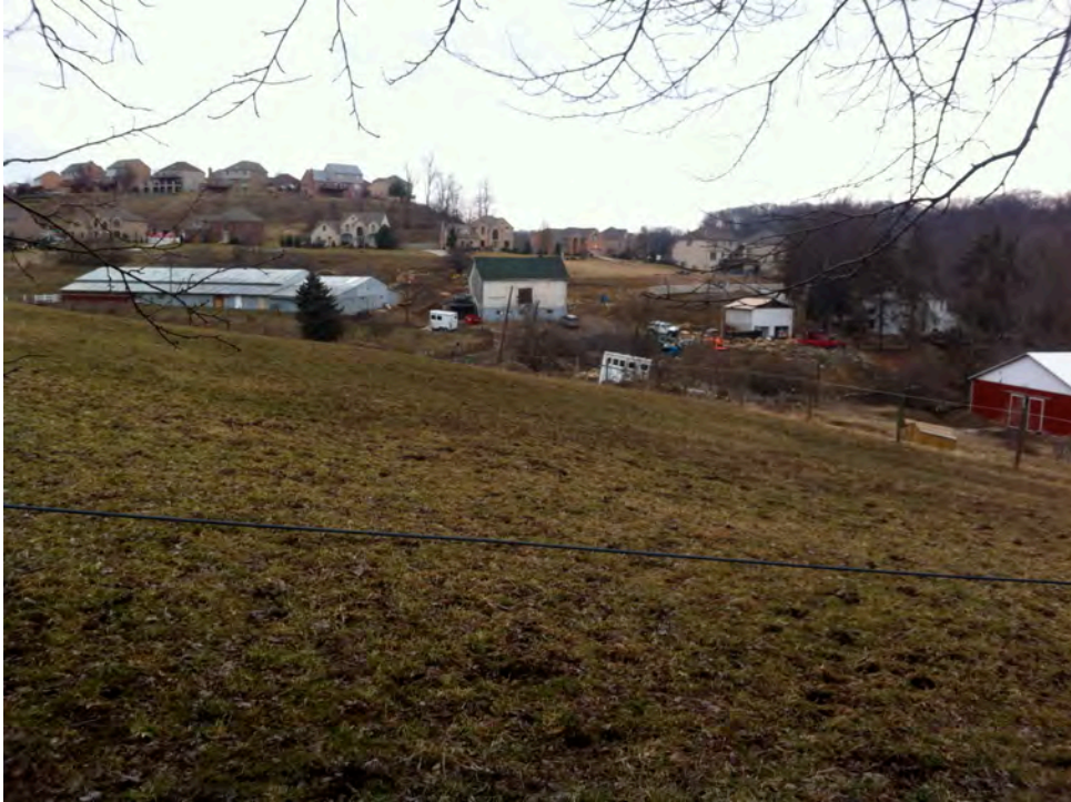
SH53 – A large detention basin helps to control stormwater runoff from Saddlebrook Dr. The basin is at left center of photo behind the pine tree. The outflow travels downslope toward right of photo behind red barn.
