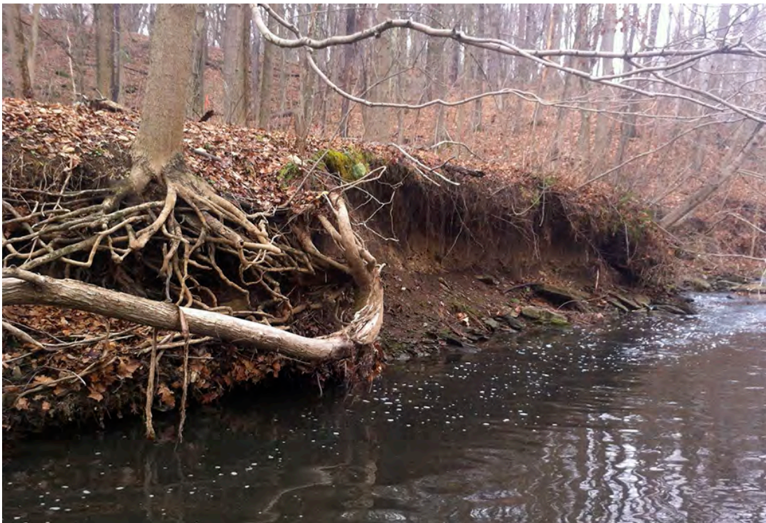
PF08 – Severe bank erosion along Piney Forks left ascending bank just downstream of a deeply incised stormwater channel. The stream is becoming increasingly detached from the floodplain along this section and the erosion is undercutting trees and adding to the sediment load of the stream.
