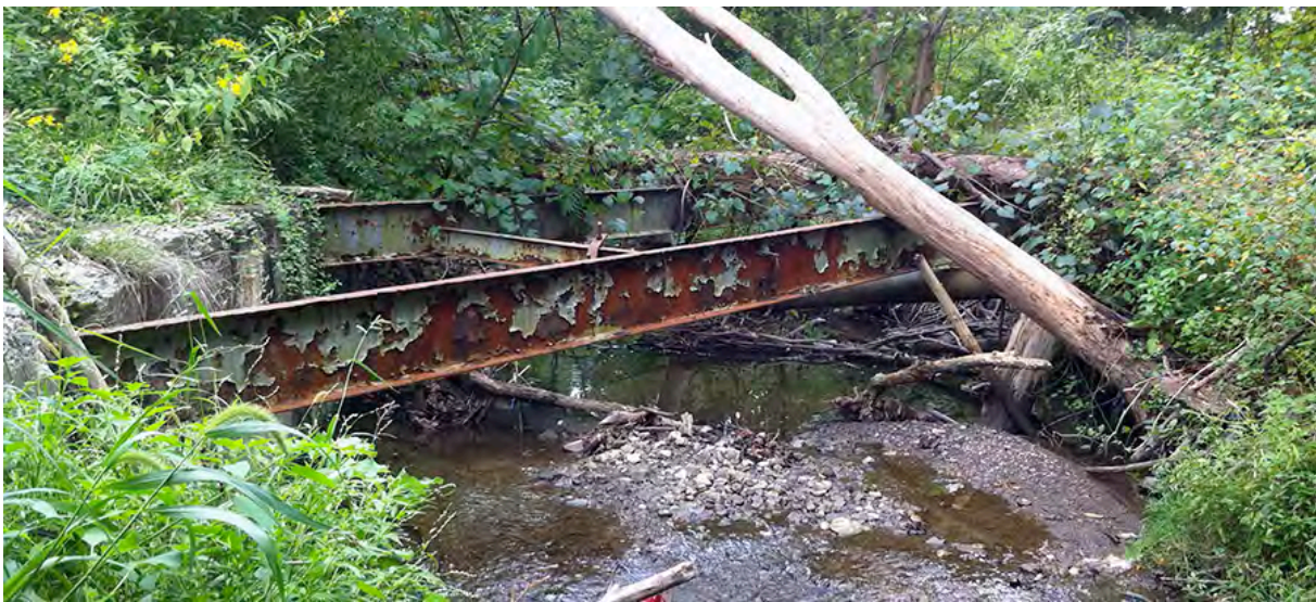
CR26 - Remnants of a nonfunctional bridge crossing of Catfish Run behind the fairgrounds buildings encroaches on the stream channel and is constantly creating debris jams that flood the surrounding area during heavy precipitation. Schoonmaker Hall and a sanitary sewer manhole also encroach on Catfish Run just upstream of this location.
