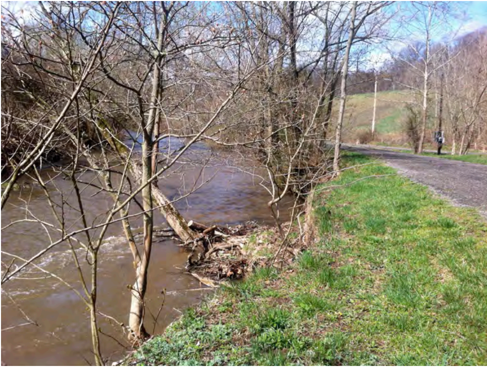
PCL31 - Bank erosion on the right ascending bank of Peters Creek is beginning to undercut the Montour Trail and impact the sewer interceptor under the trail. Jefferson Hills received a PA DEP Growing Greener grant to stabilize the banks and mitigate the problem utilizing Natural Stream Channel Design techniques. This project is scheduled to be completed in 2014.
