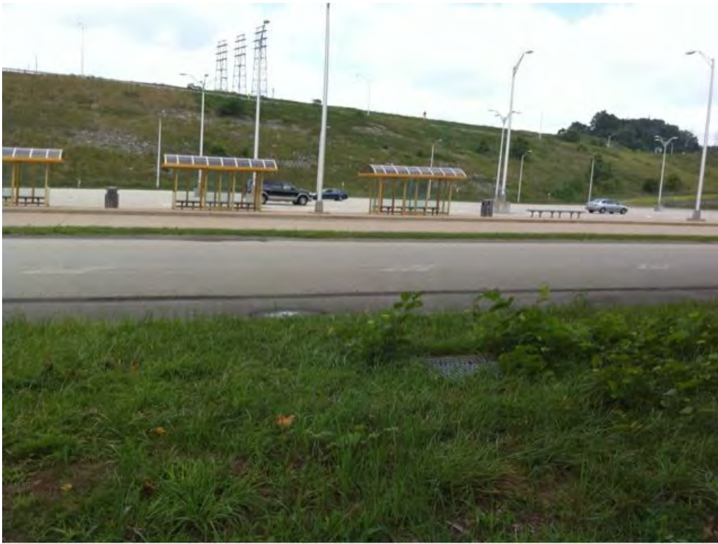
PCL40 – An approximately six acre park & ride lot with bike lane included (part of Montour Trail) was constructed as part of the Mon-Fayette Turnpike project on Peters Creek’s right ascending bank. A one acre constructed wetland detention basin was installed to control storm water runoff from this impervious surface as well as from the expressway on top of the hillside behind the parking area.
