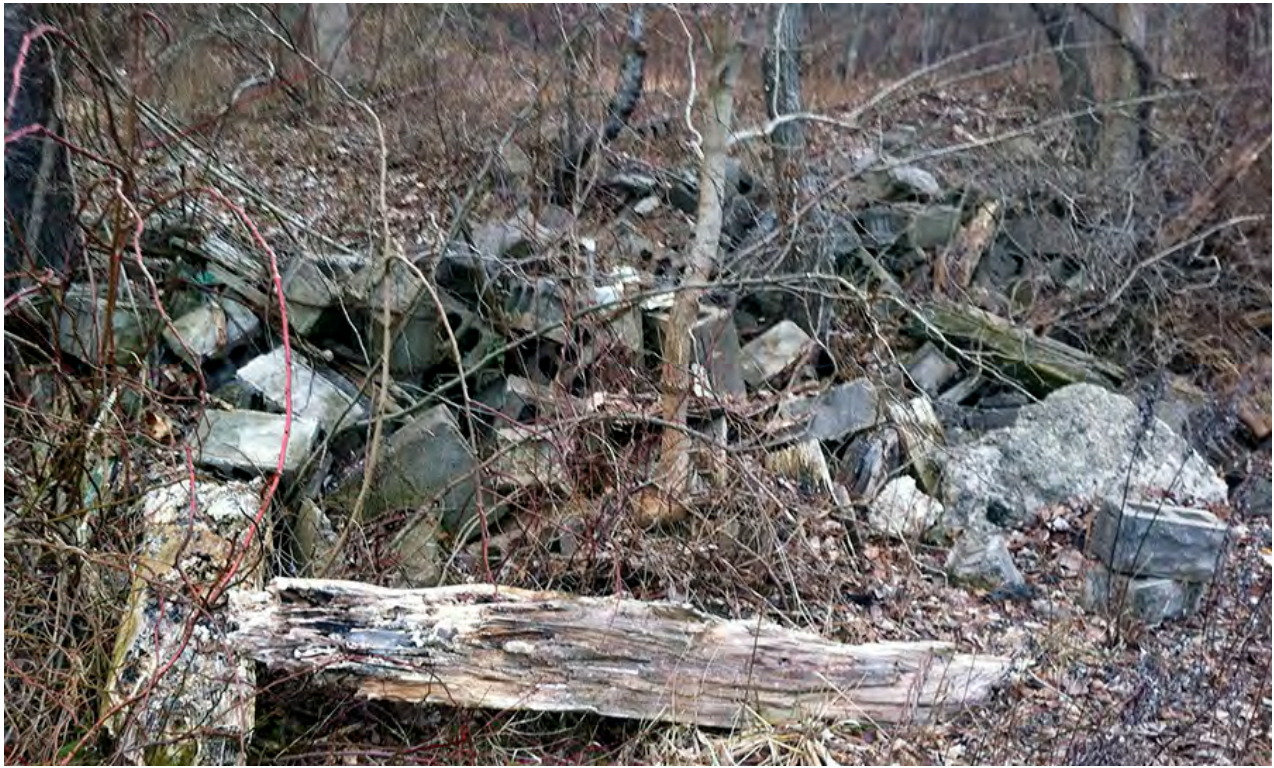
JMT06–JMT07 – Numerous piles of construction debris and rubble within the Jefferson Memorial Tributary's left and right ascending floodplain along this section of stream. Some of the debris piles appear to be recent and some appear to be of some age. It appears that the area has been utilized for illegal dumping for some time.
