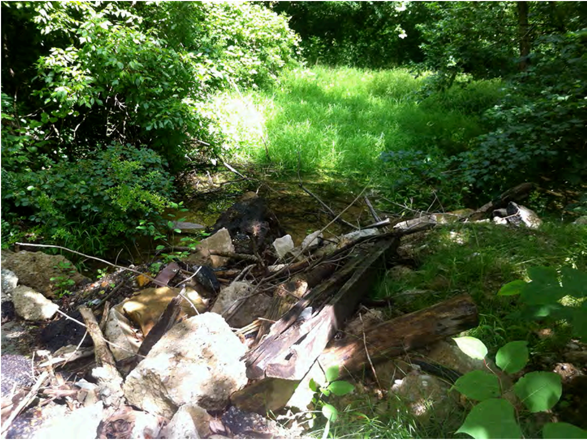
PF25 – Landowner pushing concrete rubble and other assorted debris into a wetland along the Montour Trail downstream of the new Montour Trail bridge crossing of Piney Fork east of Triphammer Rd.
