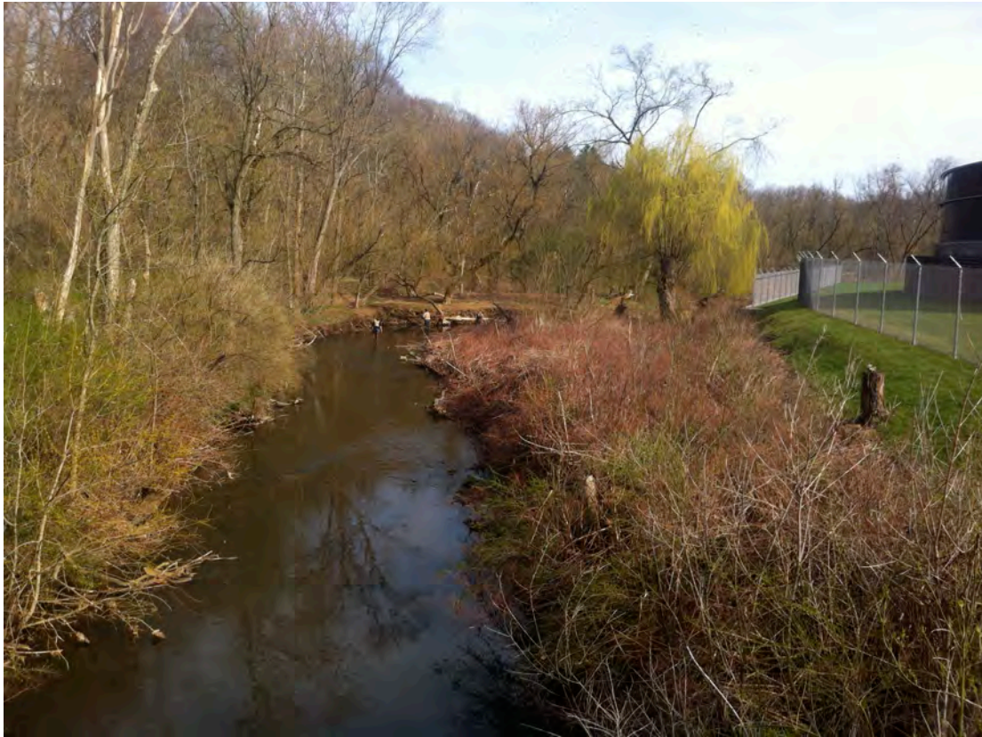
PF40 – A view of Piney Fork just downstream of the Piney Fork Wastewater Treatment Plant outfall. The Tri-Community Anglers and South Park Township stock this portion of stream with trout. Part of the upgrade to the treatment plant can be seen in the right of the photo.
