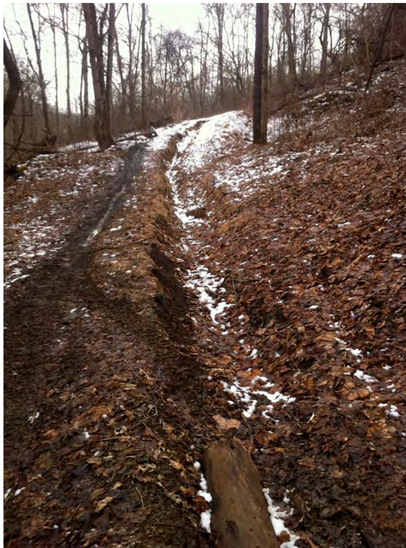
BR26 – An erosion channel created by off-road activity transports stormwater and sediment into Beam Run.
