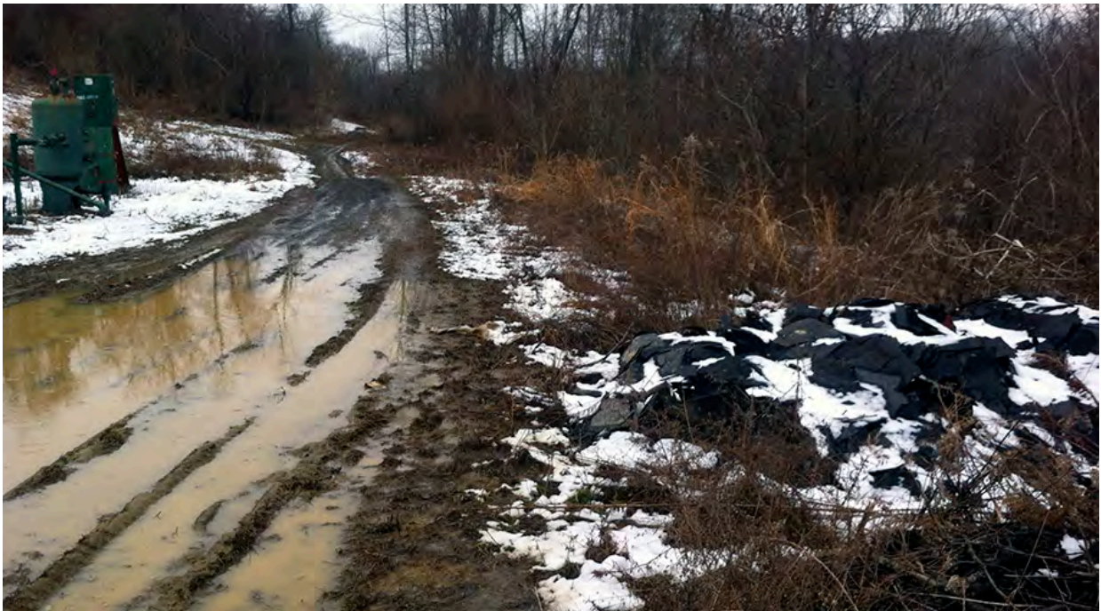
BR13 – An illegal dump site along a gas well access road that is heavily eroded by heavy off-road activity near the top of Beam Run's western slope.
