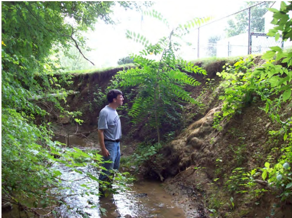
TFT10 – Stream bank erosion along the Trax Farm Tributary. The stream is detached from the floodplain. The landowner is contributing to organic enrichment by dumping grass clippings into the stream channel.
