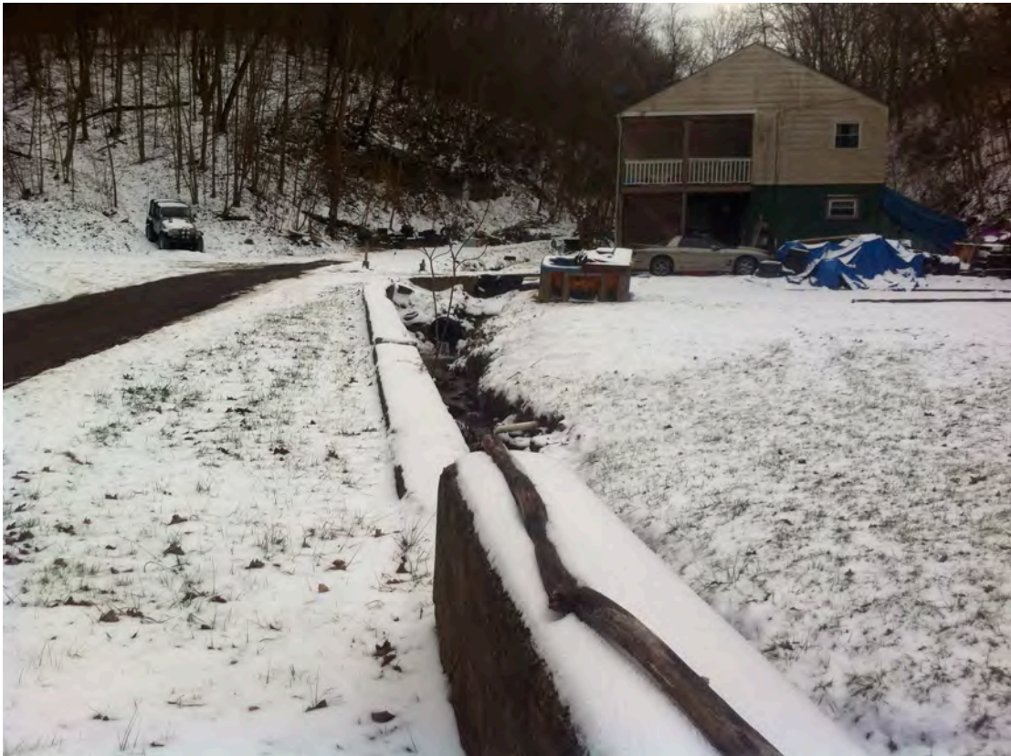
SCR16 - Scotia Run is culverted under a private driveway. A concrete wall constrains the left ascending bank for a few hundred feet downstream. The stream continues upstream in a southerly direction in a steep narrow wooded valley paralleling Rt51.
