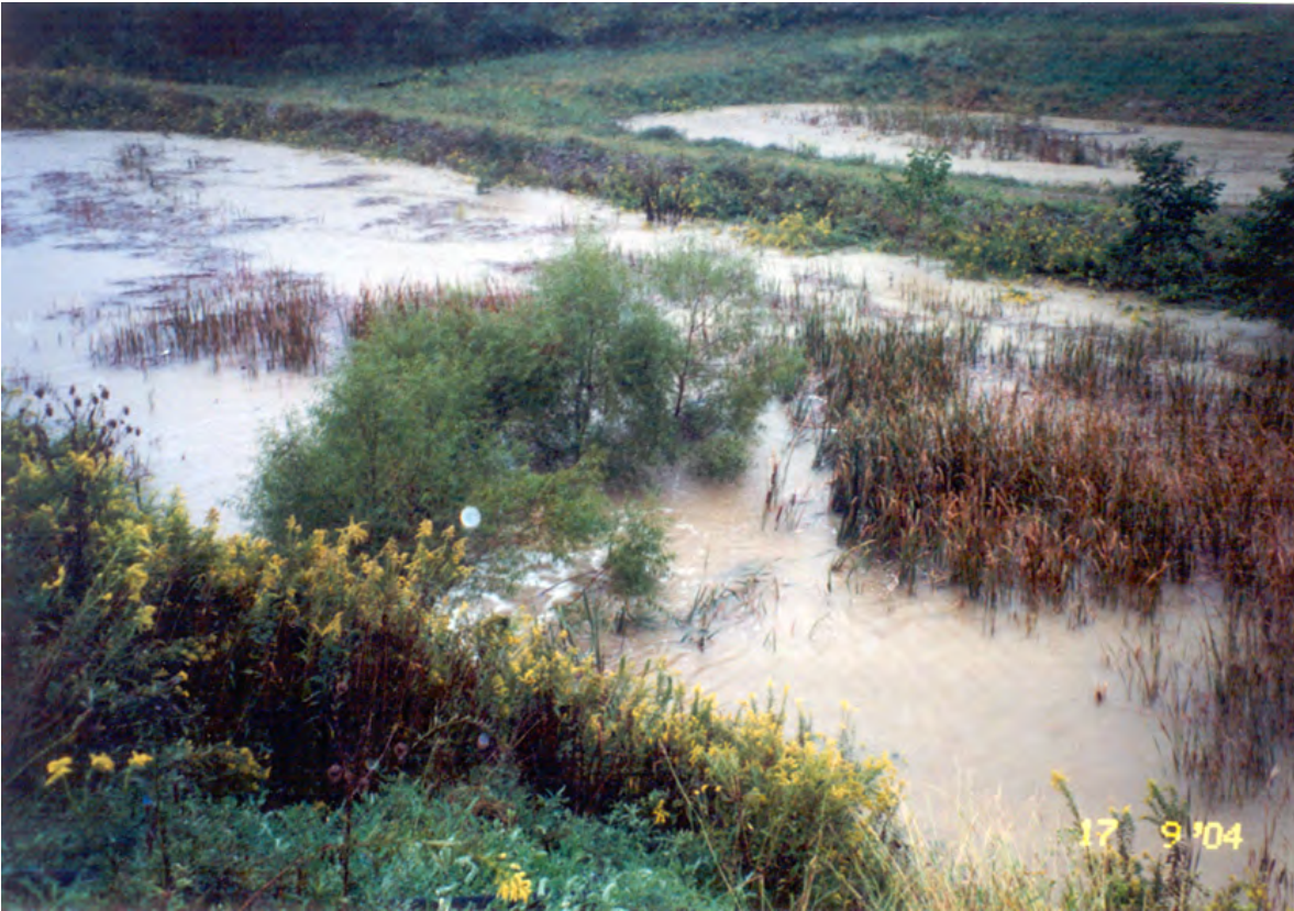
CRB14 – Two large over-engineered stormwater detention basins along the King’s School Village community in Bethel Park serve a regional stormwater function. The extra capacity of these basins helps to protect homes and infrastructure downstream during severe flooding events. The detention ponds did not overflow during the flooding of September 2004 due to remnants of Hurricane Ivan as seen above. Adequate stormwater controls are especially essential within the steeply sloped upper reaches of the Clifton Road branch of Piney Fork.
