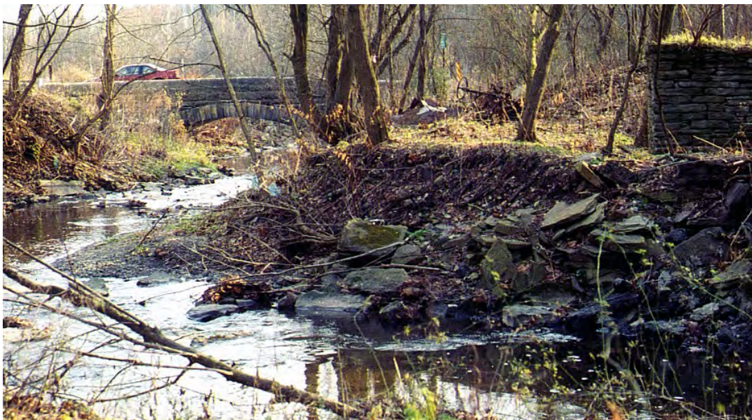
LR20 - The Cochran Mill Road Bridge is listed as stone arch bridge S-2 in the Pennsylvania Historical and Museum Commission survey of PennDOT bridges that have significant historical value. The structure is described as "segmental arch of high quality rock, faced ashlar construction; voussoirs dressed; parapet finished with curved course." The survey entry reports the date as 1901. Remnants of the the saw and grist mill of Joseph Cochran on Lick Run just upstream from this bridge can be seen in the upper right of the photo. The mill race - the water diverted from the stream to power the mill - ran to the west of the stream, through the mill near the western end of the bridge site.
