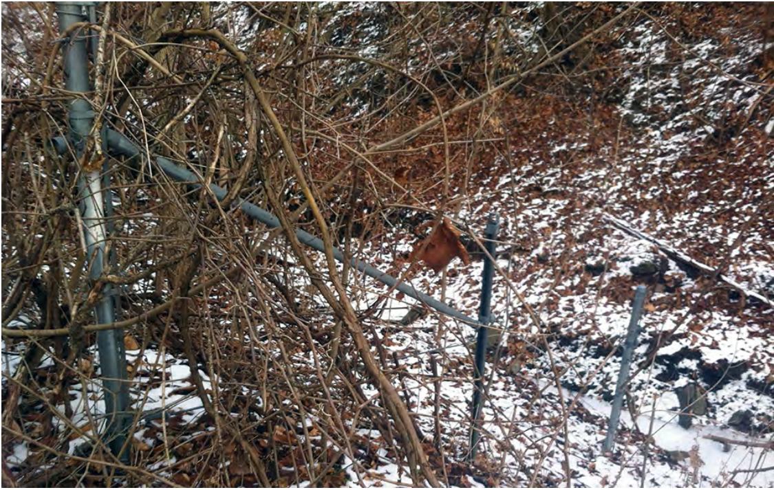
PCLT06 – Remnants of fencing installed as part of the Mon-Fayette Expressway project just downstream of the erosion gully. This fencing was placed across the stream channel. The value of this fencing in this location is questionable. The fencing is often vandalized by local off-road enthusiasts. There is little to no maintenance provided following installation and the unintended affects on local wildlife can be quite negative.
