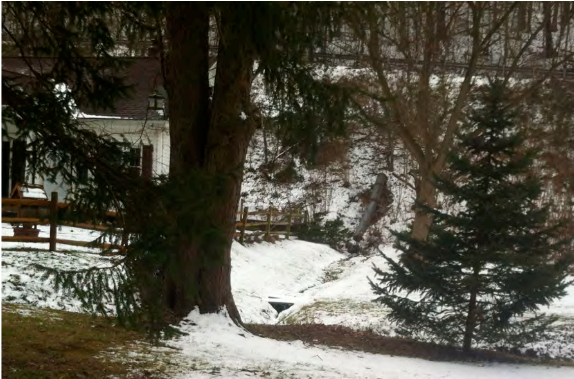
SCR12 - A storm water outfall from Rt51 along the steep hill in the upper part of photo is piped to Scotia Run's right ascending floodplain. It flows across the floodplain in an open drainage channel and enters Scotia Run which flows between the house and McGrew Rd. A number of such outfalls from Rt51 exist along this section of Scotia Run.
