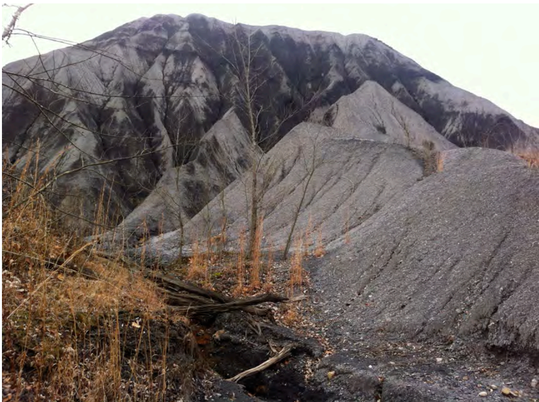
PCL21 – This 30 acre, 120 foot coal waste pile of approximately 100 million tons encroaches on Peters Creek’s southern shore for nearly 3,000 feet from just upstream of the Ravensburg Bridge to the western portal of the Ravensburg Tunnel. Material from this waste pile erodes into Peters Creek and metals and other chemicals leach into the creek. The waste pile was created by United States Steel Clairton Coke Works as part of a coal cleaning operation. The exact composition is unknown since it was created prior to modern regulations.
