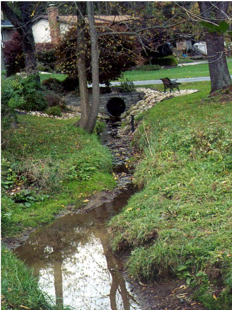
CRB37 – Piney Fork flows through front and back yards of residences along Clifton Rd. The stream is also culverted at a number of locations along Clifton Rd.
