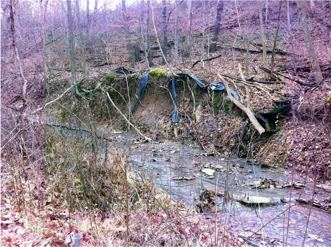
MRT11 – Eroding right ascending bank of Mineral Run. Remnants of silt fence that is little more than refuse.
