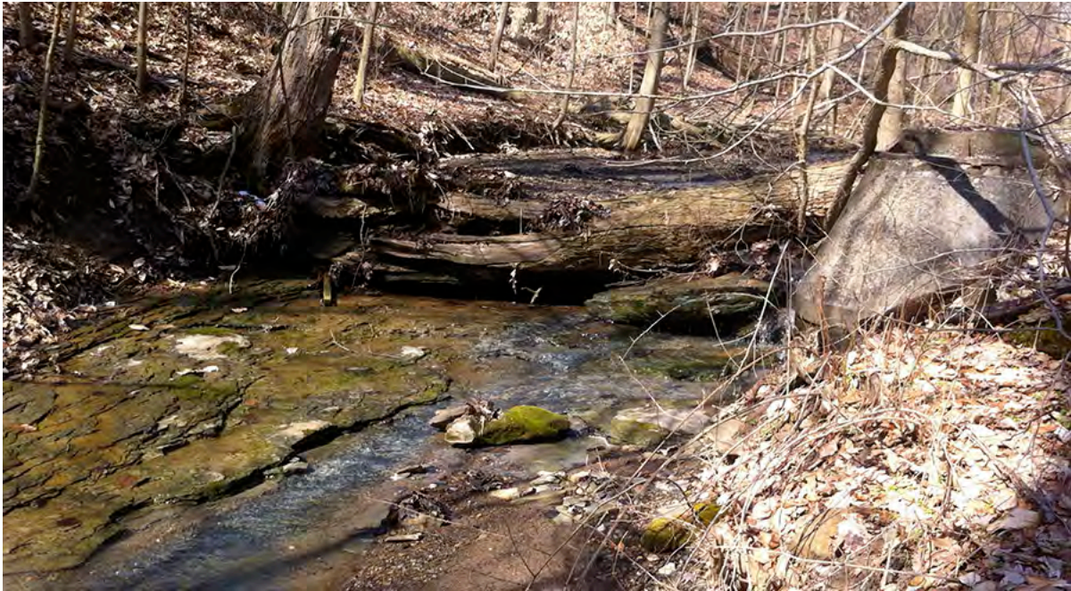
BR56 – Sanitary sewer infrastructure runs the entire length of Beam Run to Peters Creek. At a number of locations the infrastructure encroaches on the stream channel as seen above or stream bank erosion has exposed the sewer line as at BR15. Sewer infrastructure within the stream channel often leads to raw sewage within the stream.
