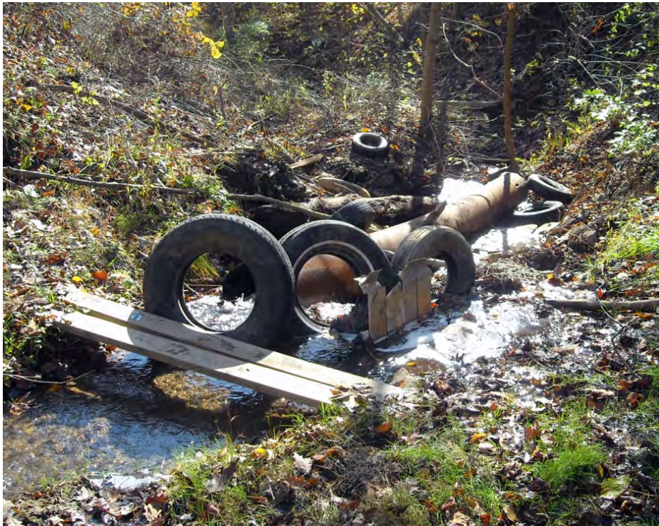
Illegally discarded tires and other debris accumulates at a non-functional pipe blocking the channel of the Jefferson Hospital Tributary. There is also an abandoned truck along this section of stream.
