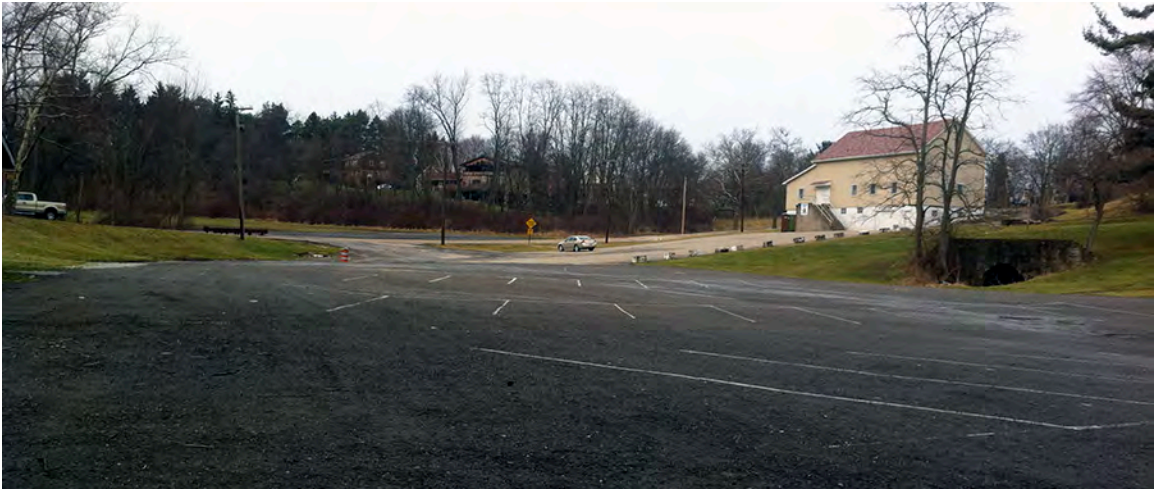
CRT27 – Catfish Run's East Branch Tributary is culverted for approximately 700 feet under this asphalted parking area and the Haunted House facility. A structure holding a natural spring can be seen to the right of the parking area. The spring flows into the East Branch under the culvert. The East Branch initially enters the culvert just north of Hundred Acre Drive.
