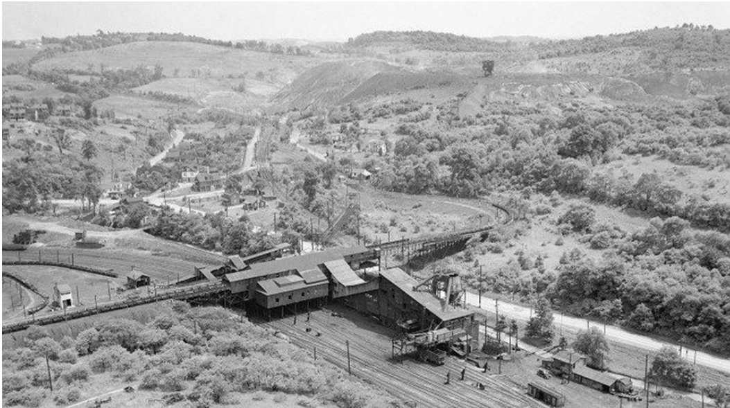
A 1946 view of the Montour No. 10 Mine operation in Library along Piney Fork. The railroad tracks run under the tipple. Piney Fork and Brownsville Rd are to the right of the tipple and pass under tracks that lead to the coal waste pile.
