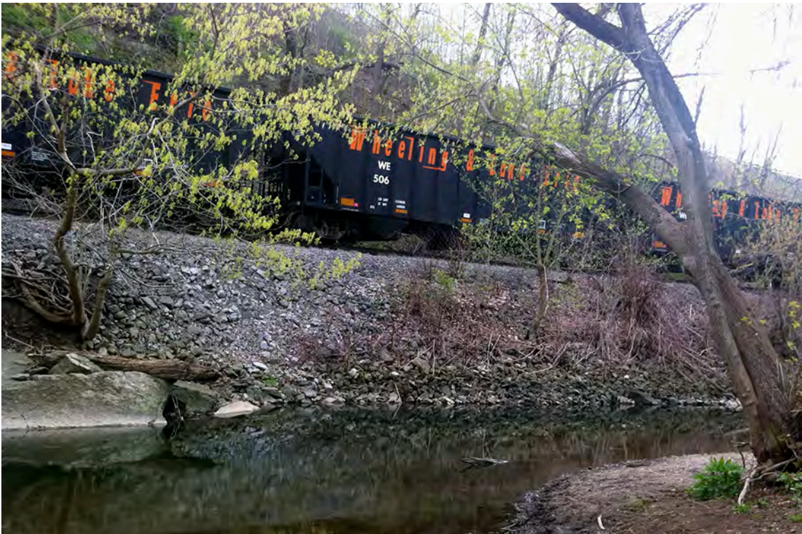
Just downstream of PCM35 the Wheeling & Lake Erie Railroad Clairton Branch tracks severely encroach on Peters Creek's channel on the left ascending bank at the site of a popular fishing hole. Large concrete debris has been placed along the bank to mitigate erosion and ballast erodes into the creek.
