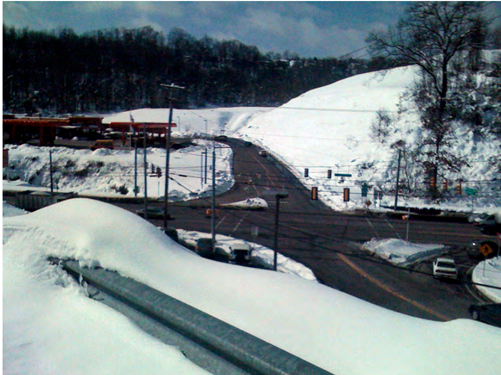
LW40 – This section of Rt51 at its junction with N Lewis Run Rd floods during heavy rain events. Lewis Run meets the RT51 Tributary just to the right of the photo and is immediately culverted under Rt51 and the Sheetz access road.
