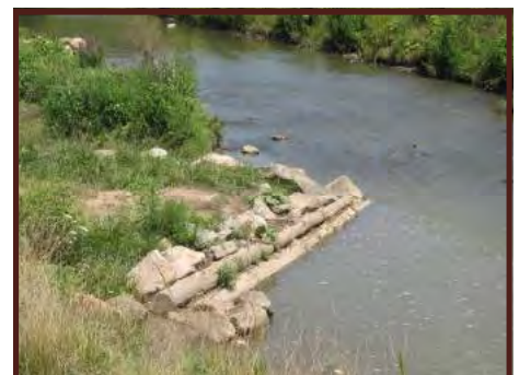
Stream Deflector placed in Pine Creek near Roessing Bronze Site
