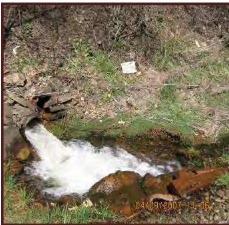
AMD Treatment System Outflow, Willow Run
