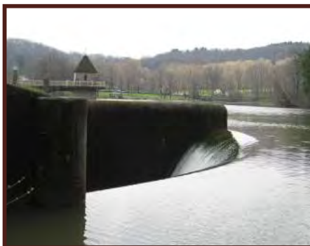
North Park Lake Spillway
