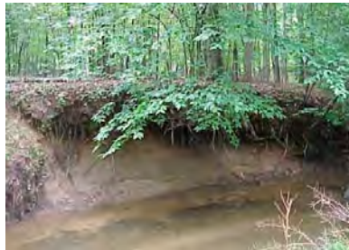
Significant Erosion due to Excess Runoff
