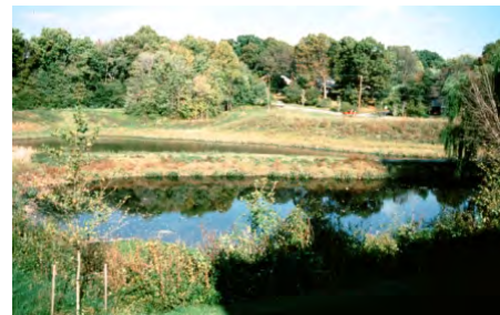
Wet Pond BMP to Reduce Erosion
