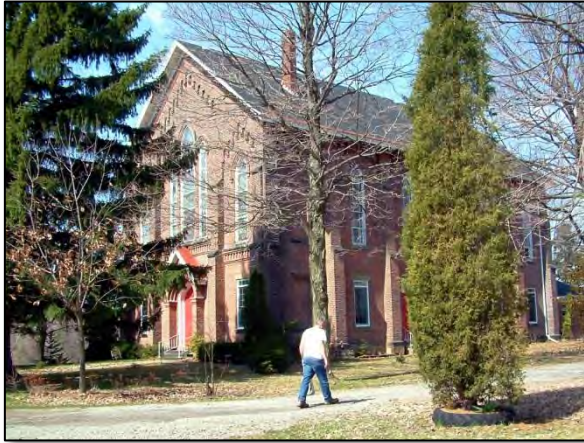
Figure 6.38: Robinson United Presbyterian Church, Washington Road, Robinson Township, 4/5/2005.
