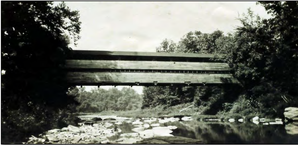
Figure 6.33: The Potter Bridge, a covered wooden span built in 1865, carrying the Frankfort Road over Raccoon Creek near its mouth; collapsed on Sunday, August 5, 1923. Photo courtesy of James G. Camp III, Director, Beaver County Department of Public Works.
