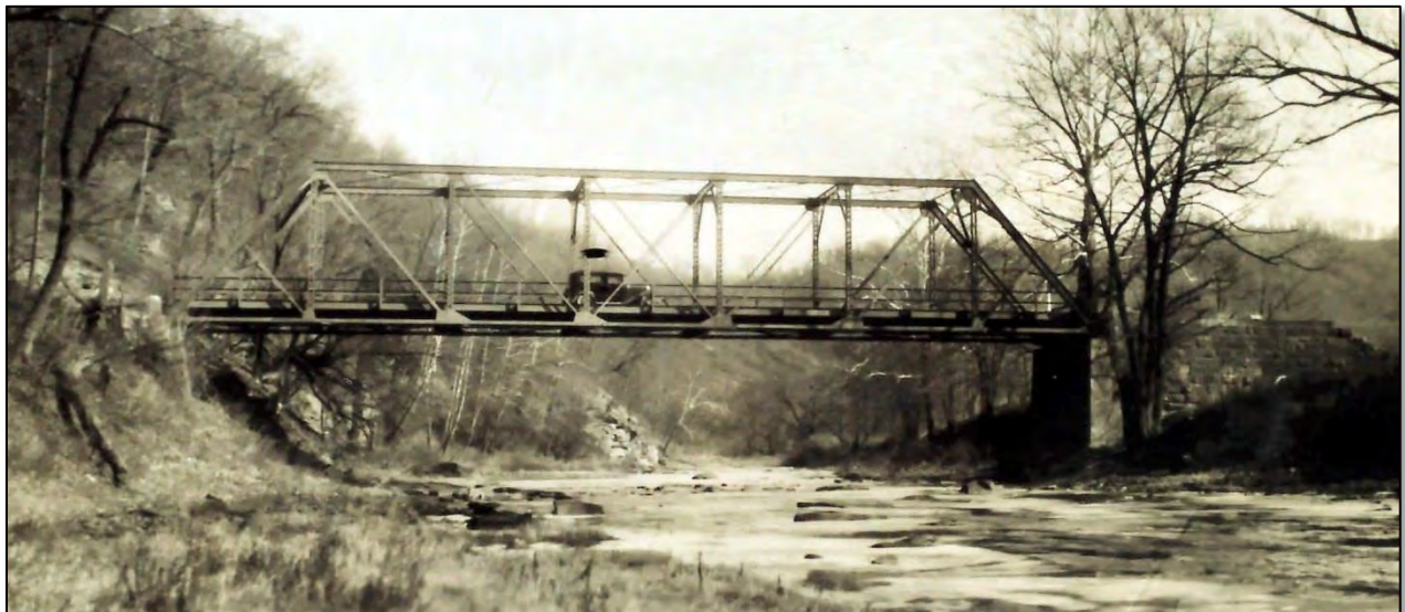
Figure 6.32: Potter Bridge in Potter Twp. pre-1936; moved in 1938 to Independence Twp. to serve as Link's Bridge until 2006. Note the "new" car on the bridge and the photographer's vantage point, now under several feet of water due to the higher pool of Montgomery Dam. Photo courtesy of James G. Camp III, Director, Beaver County Department of Public Works.
