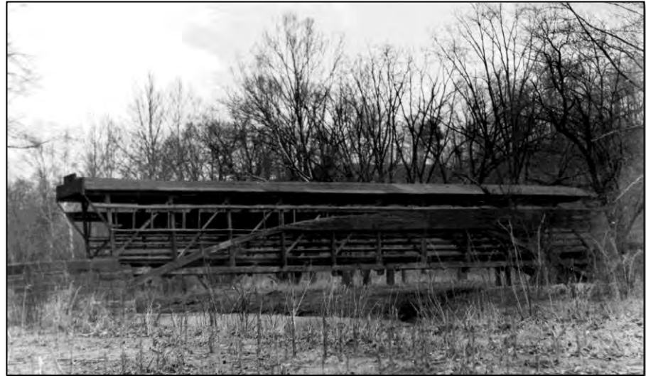
Figure 6.31: Link's Bridge over Raccoon Creek in Independence Township, Beaver County, built in 1887. This wooden structure was replaced in 1938 by relocating the metal Potter Bridge from twenty miles downstream. Photo courtesy of Raccoon Creek State Park Archives.
