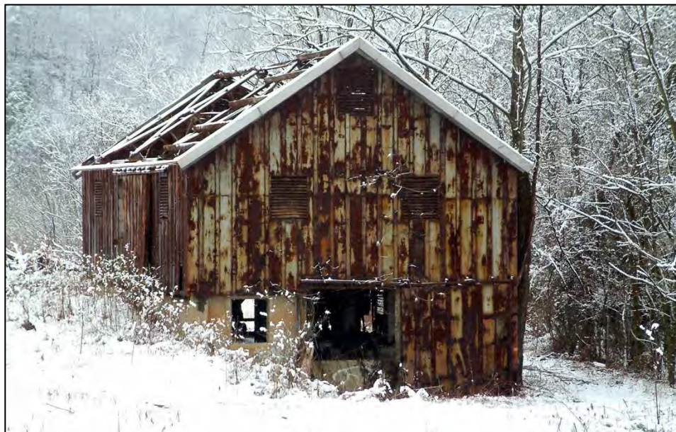
Figure 6.29: The Monaca Tank Farm's Blending Barn #1 awaits a new purpose; 3/11/2011.
