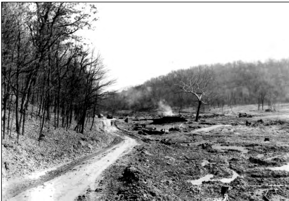
Figure 6.8: Beginning construction of Raccoon Lake, ca. 1948-49. Photo courtesy of Raccoon Creek State Park Archives.
