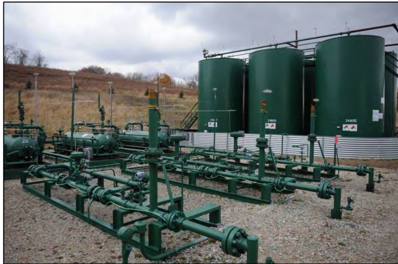
Figure 7.1: Storage tanks and piping at one of the natural gas wells in Cross Creek County Park. Copyright ©, Pittsburgh Post-Gazette, 2014, all rights reserved. Reprinted with permission. Story: 12/13/2013.
