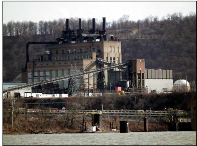
Figure 1.29: AES Beaver Valley's 125-megawatt power generating plant, formerly the boiler and powerhouse of "Kobuta."
