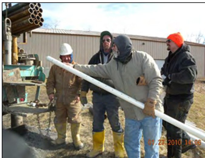
Figure 8.7: Bruce Leavitt prepares the piezometer screen for test site EP1 as Randy McKay, John Rigger and Tim Danhey look on, 1/27/2010. Photo courtesy of BioMost, Inc.
