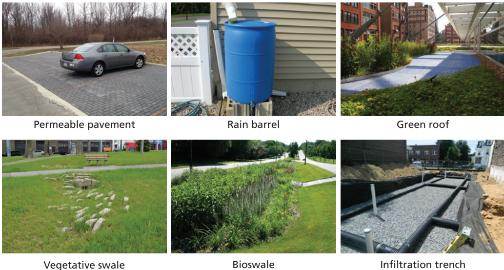
Figure 2.3 Examples of Green Stormwater Infrastructure
