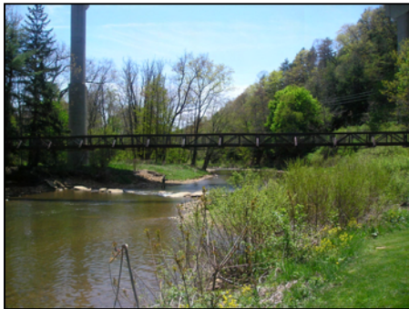
A footbridge crossing North Fork Redbank Creek
