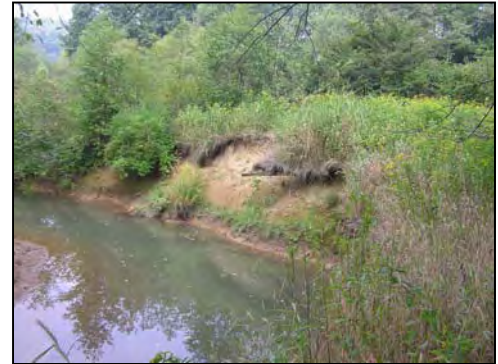
Eroding streambank along Redbank Creek
