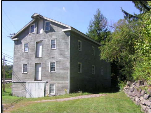
Humphrey's gristmill, located in Port Barnett, is the seventh oldest gristmill in the Lumber Heritage region
