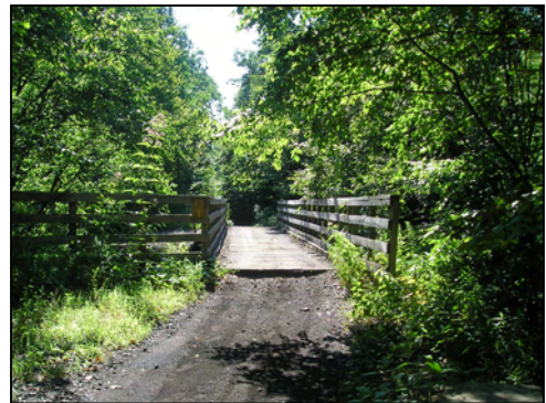
Armstrong Trail crossing Mortimer Run
