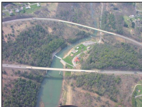
Aerial photo of Interstate 80 crossing North Fork Redbank Creek in Brookville
