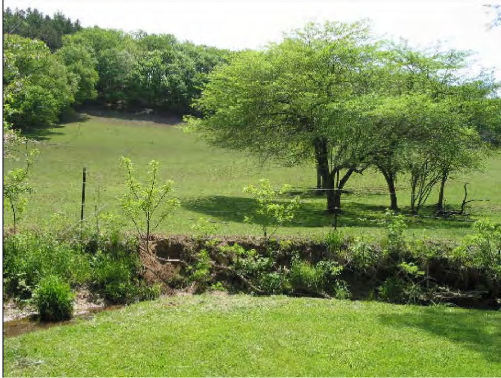
Figure 27. Stream bank instability and storm water incision
