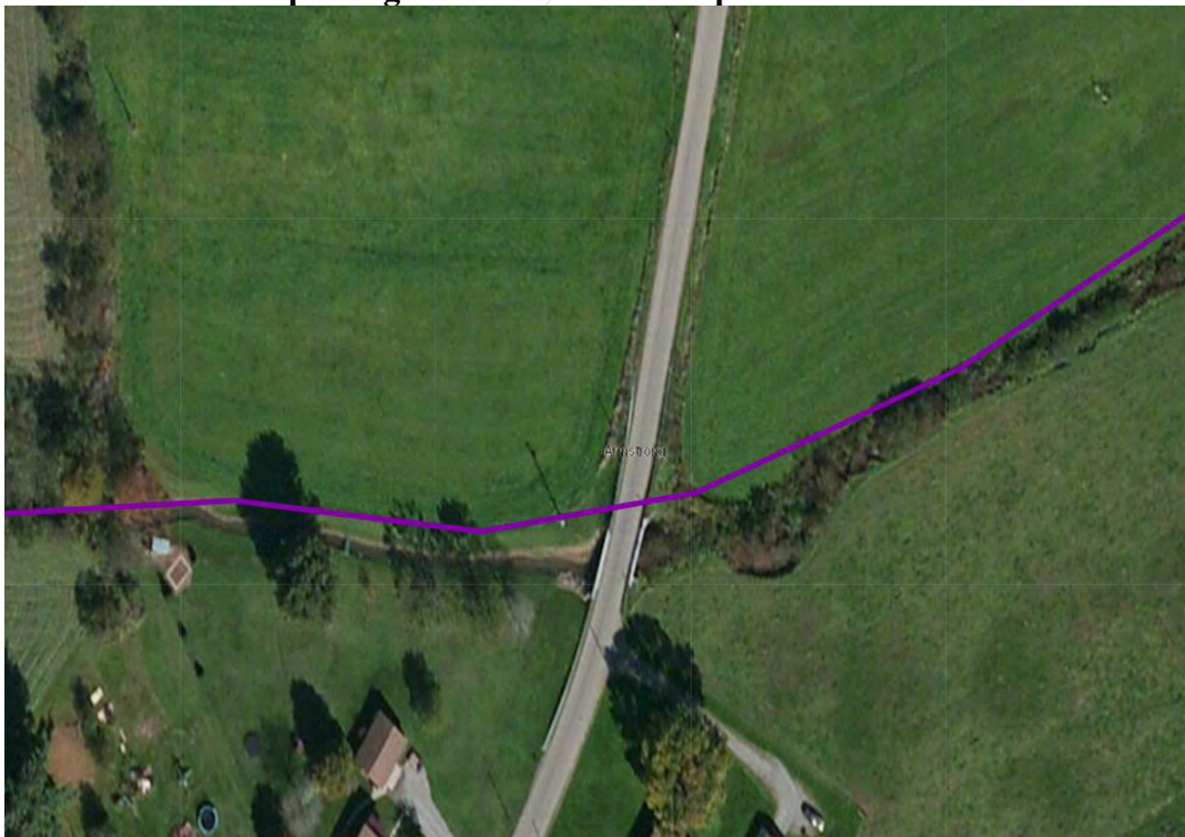
Figure 34. The lower stretch of the SBSF Pine Creek (adjacent to SR 1028) show pooling and instream development of wetlands
