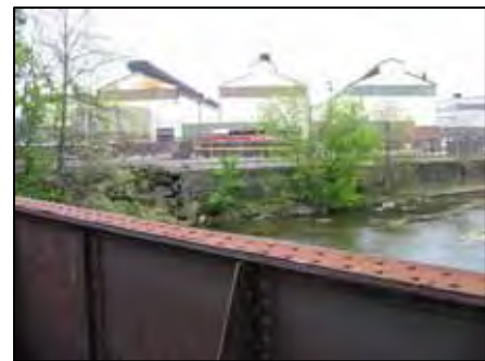
Industrial plant along the Shenango River
