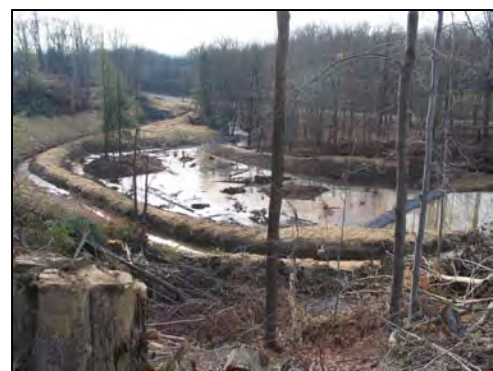
Fox Run AMD Passive Treatment System (photo courtesy of Mercer County Conservation District)
