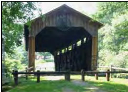
Kidd's Mills Covered Bridge
