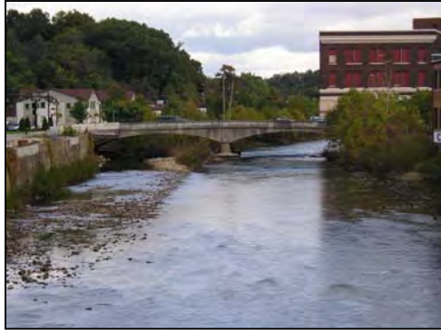
Gravel bar developing on Neshannock Creek as a result of erosion and sedimentation
