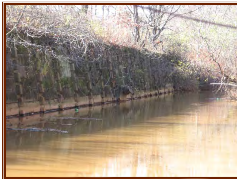
Retaining walls (MR-4 Photo 4)
