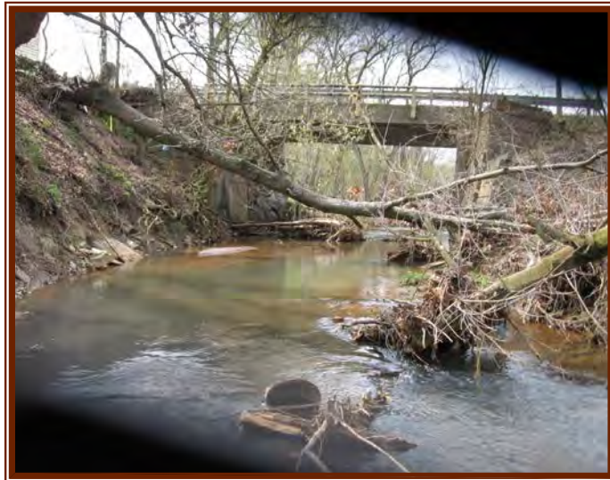
Multiple stream crossings in section (RR-8 Photo 9)
