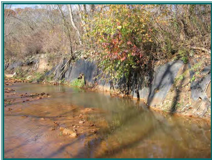
Area of stream bank erosion (MR-2 Photo 2)
