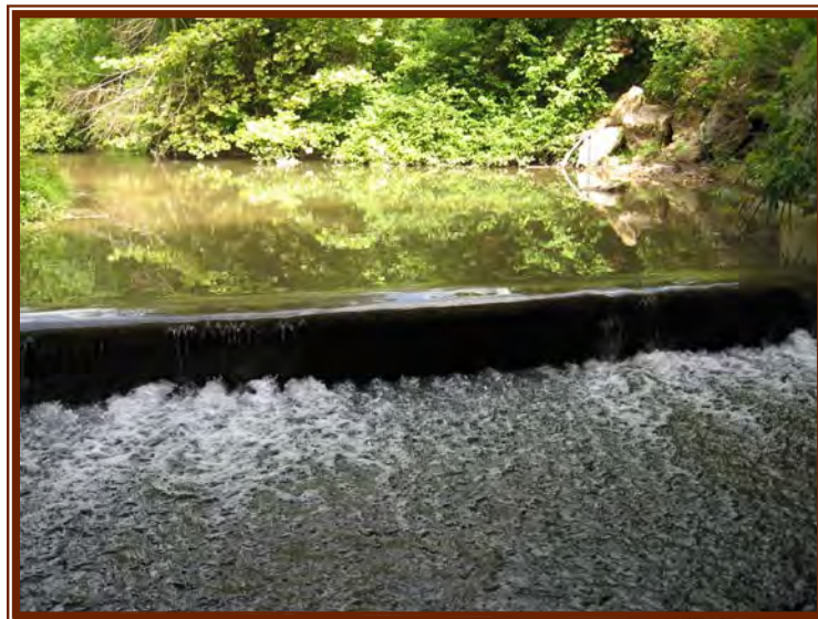
PA 50 Bridge and spillway (MR-13 Photo 8)
