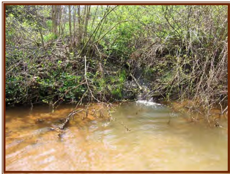
Drainage (RR-10 Photo 6)
