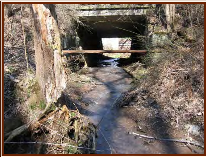
One of many crossings (RR-6 Photo 4)
