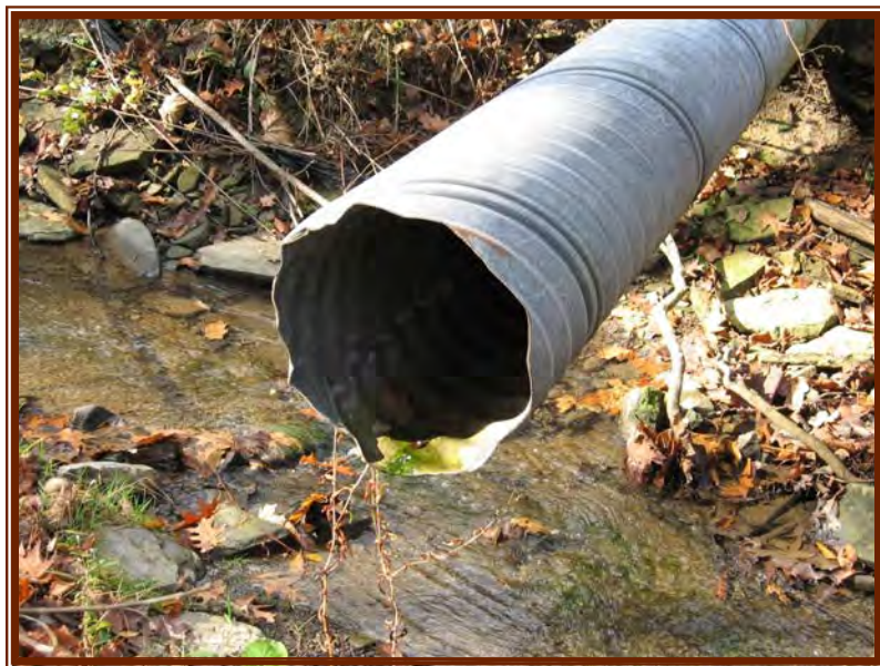
CMP Pipe outfall directly to Coal Run (CR-3 Photo 4)
