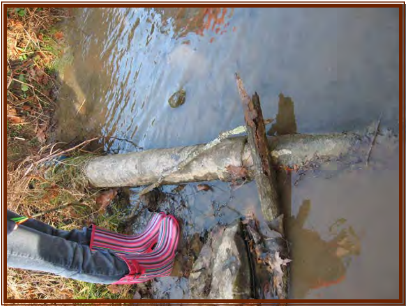
Sewer line crossing in stream (CR-5 Photo 1)
