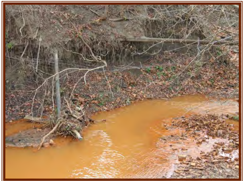
Exposed Pipes (MR-6 Photo 16)
