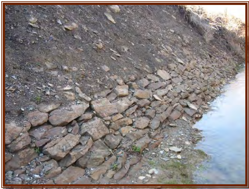
Trail stabilization (RR-4 Photo 2)
