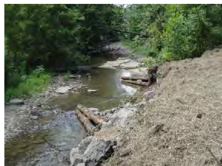
Land disturbed by the construction is properly restored and seeded.
