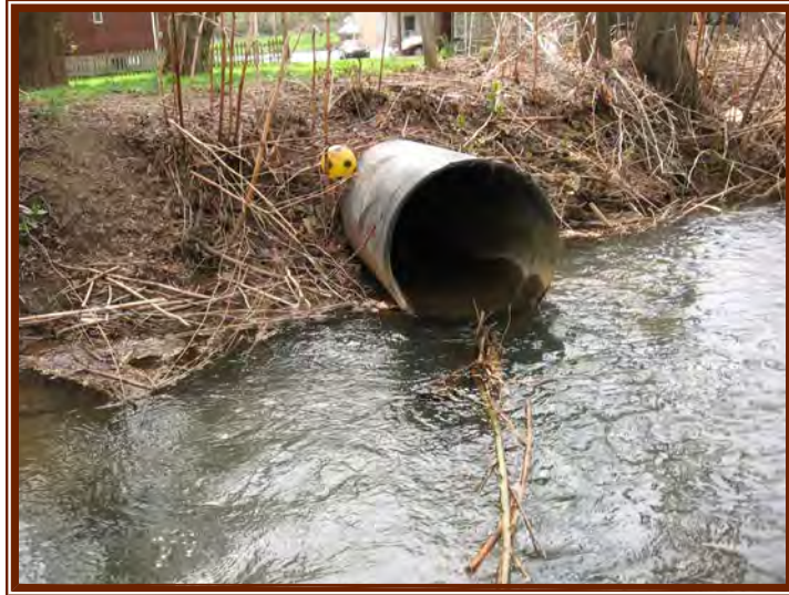
One of many outfalls (RR-8 Photo 3)
