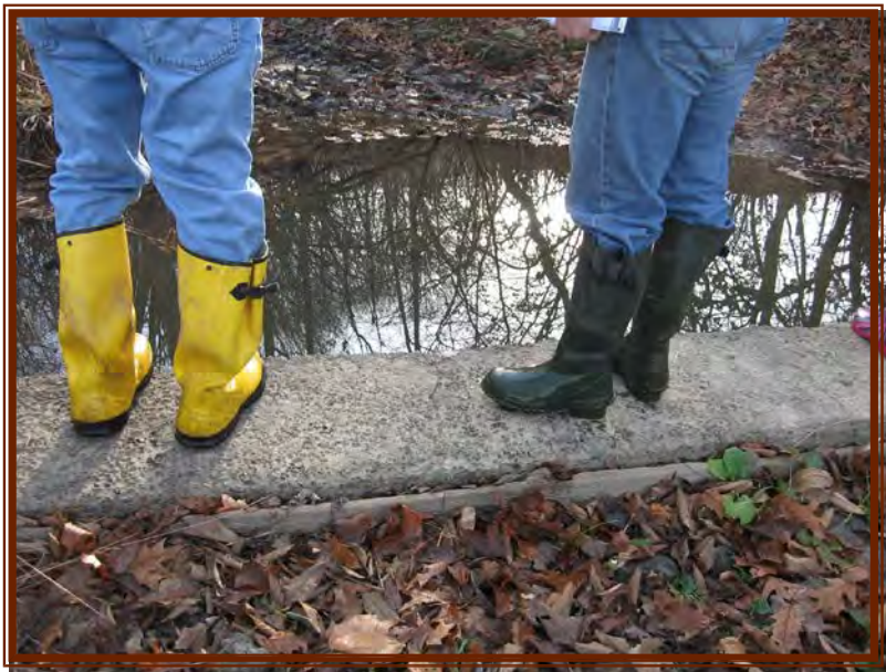
Concrete encased pipe (CR-4 Photo 2)
