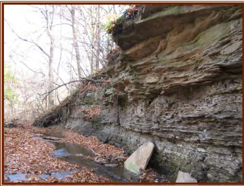
Severe bedrock erosion (CR-3 Photo 6)
