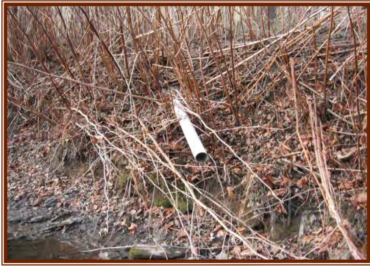
Pipe Outfall (RR-2 Photo 5)
