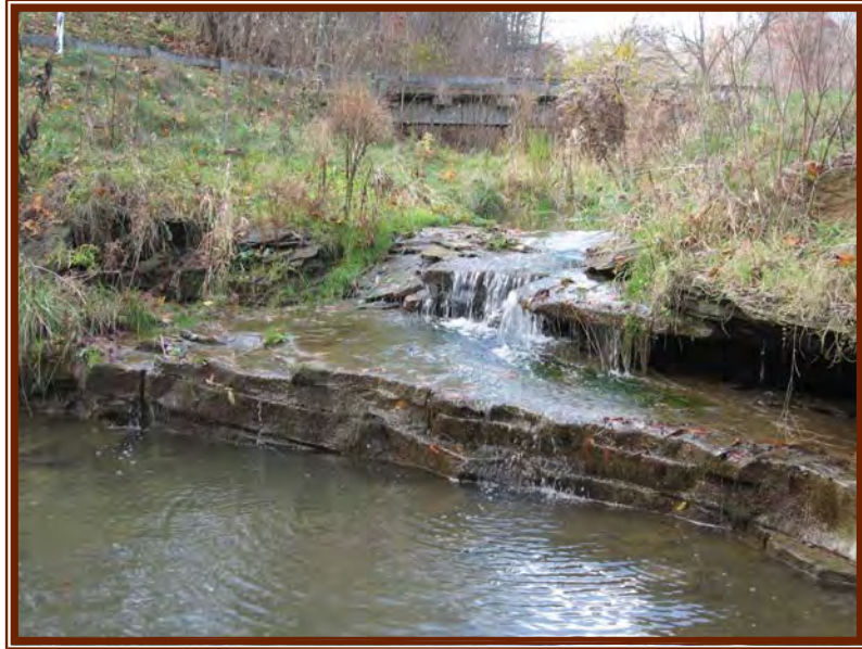
Concrete barrier (CR-3 Photo 15)
