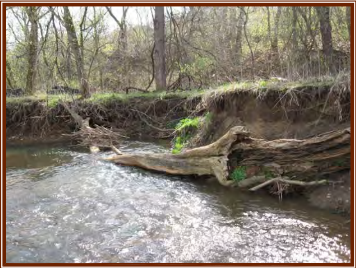
Bank erosion (RR-7 Photo 6)
