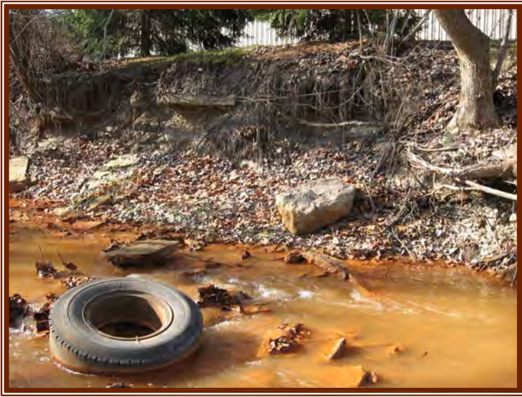
Obstructions (MR-10 Photo 14)
