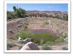
The primary stormwater management benefit of dry extended detention basins (left and right) is peak rate control. Water quality benefits can also be achieved when water is held for an extended period.
