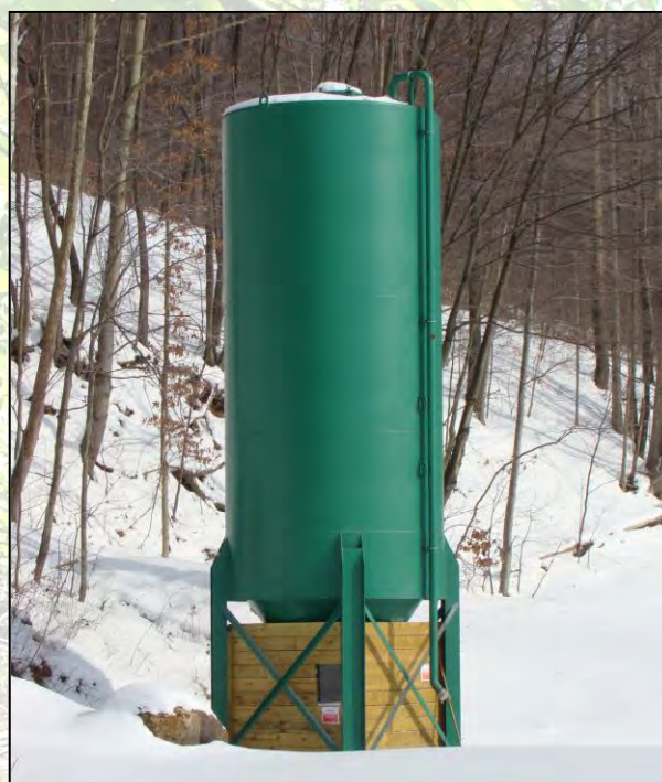
Figure 31. Limestone doser like the one that will be installed on Tubmill Creek to treat the Stanton Bridge AMD discharge. Photo by Melissa Reckner.
