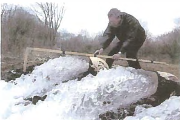
Spreaders Sending Mine Water to Ponds
