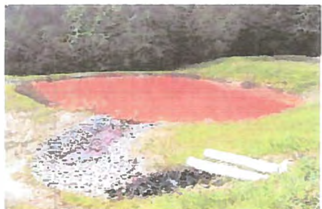
Mine Water Emptying into a Limestone Channel then into the Primary Treatment Pond
