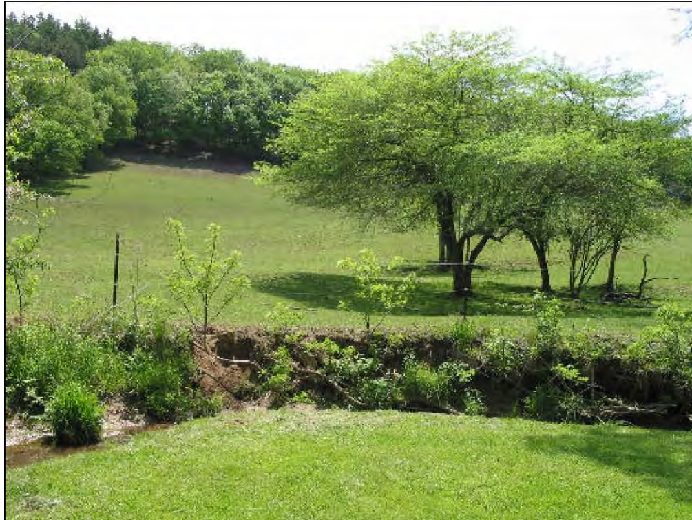
Figure 27. Stream bank instability and storm water incision
