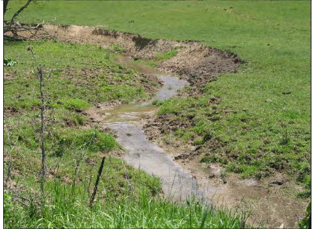
Figure 33. Elevated stream banks of silt cause in place pooling and downstream flooding
