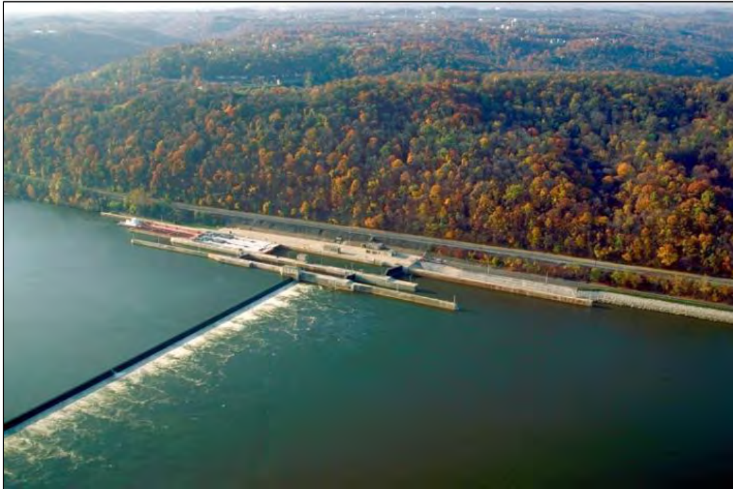
FIGURE ES-6 Dashiels Locks and Dam today
