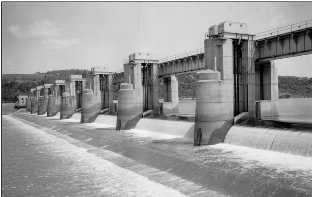
Photo 3-2: Emsworth Main Channel Gated Dam, 1938
