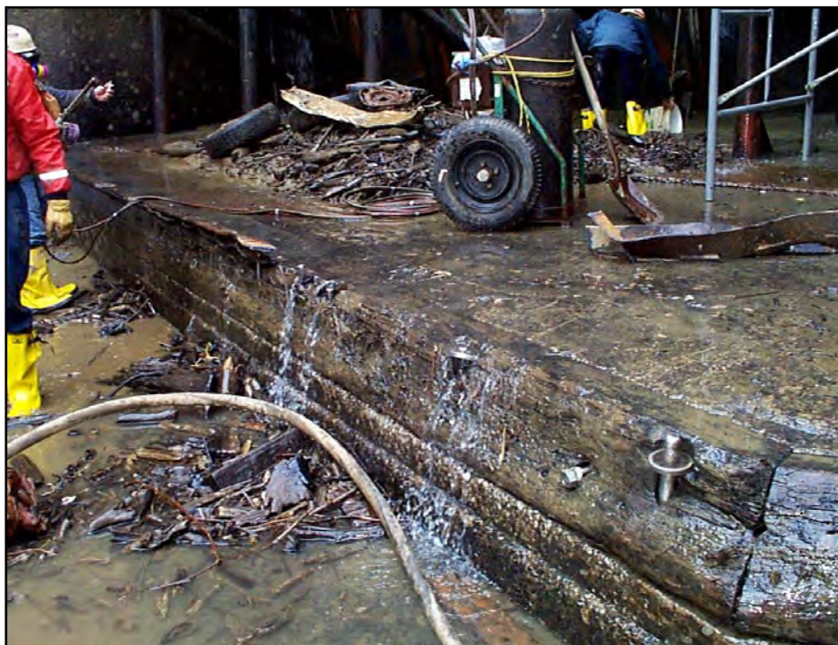
Photo 4-2: Miter Gate Sill, Emsworth Auxiliary Chamber
