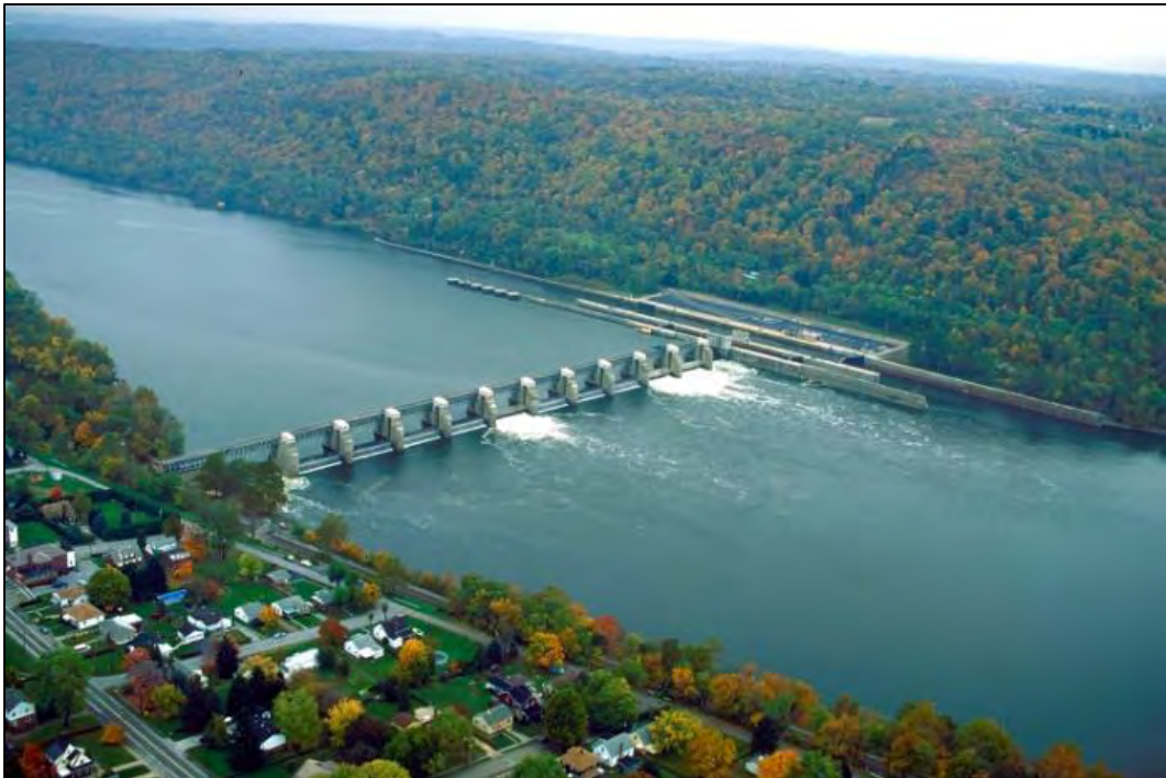
FIGURE ES-5 Montgomery Locks and Dam today
