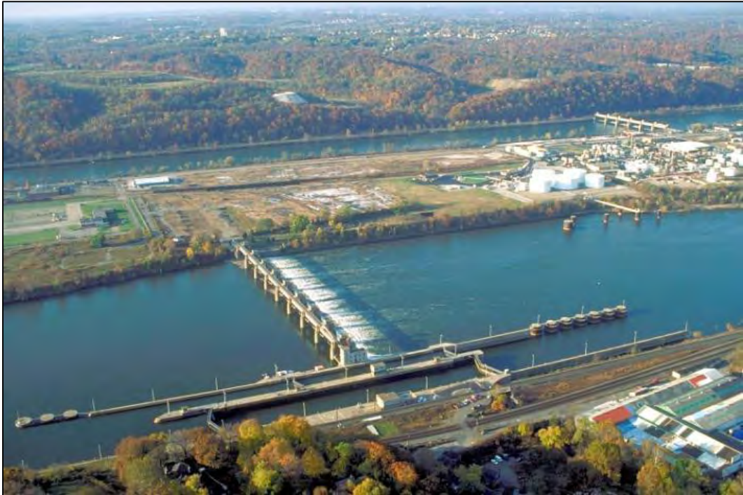
FIGURE ES-4 Emsworth Locks and Dams today
