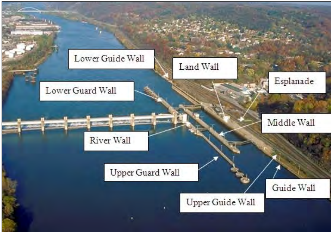
Photo 4-1: Lock Wall Component Nomenclature
