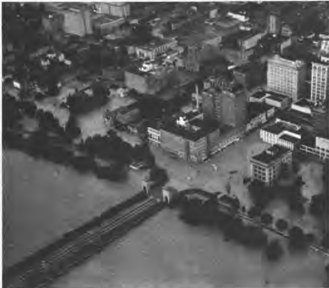
Wilkes-Barre, Pennsylvania. Flooding in the area of Market Street and the public square caused by tropical storm Agnes in June 1972.
