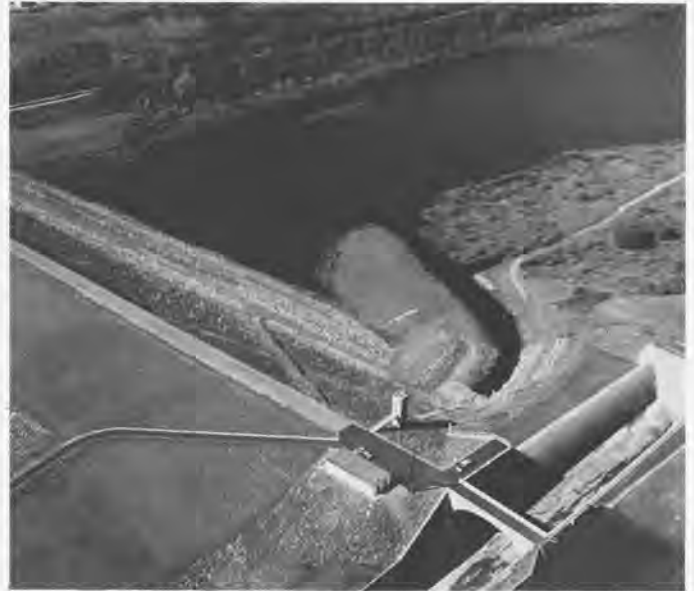
Stillwater Lake. Embankment with side-channel spillway to right. Highway at left shown is Pennsylvania Route 171.
