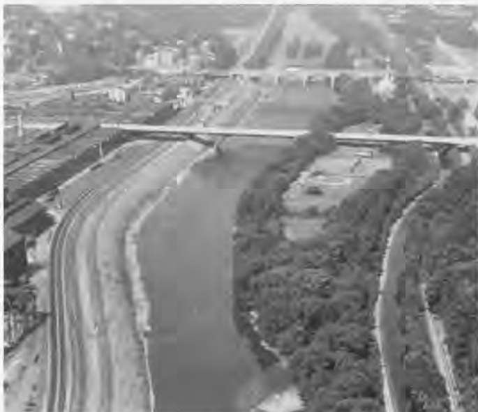
Flood control project at city of Bethlehem (at left) includes levee and pumping stations. View is looking upstream on the Lehigh River.
