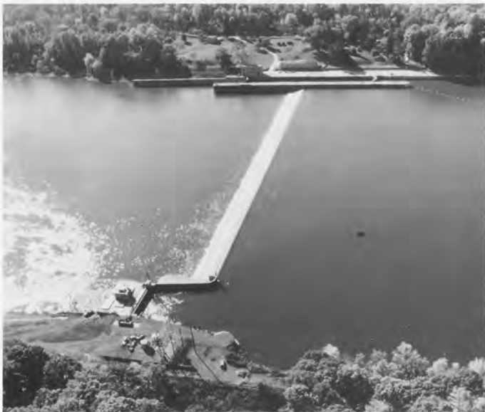
Lock and Dam 6, Allegheny River. In the foreground is the hydro-power facility.
