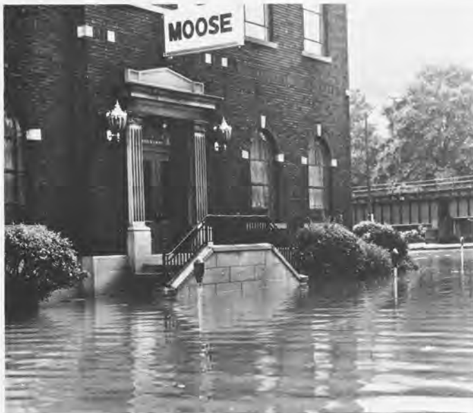
Tyrone. Flooding on South Logan Avenue in vicinity of Moose Hall during tropical storm Agnes in June 1972.
