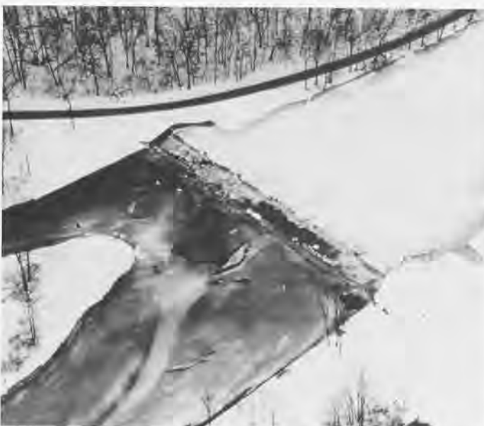
Oil City, Ice Control Structure—note the fixed concrete weir on Oil Creek.
