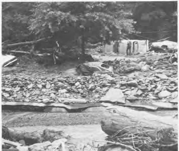
Flood Damages in Johnstown.
