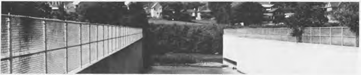
Scranton local flood protection project, floodwall and outlet flume for Roaring Brook.
