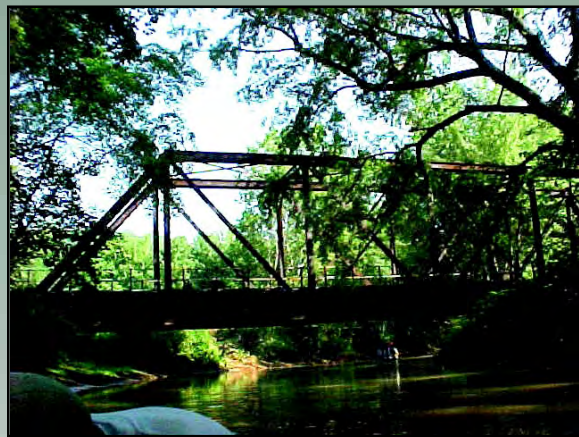
Baltimore & Ohio Railroad Bridge over Crooked Creek near Creekside
