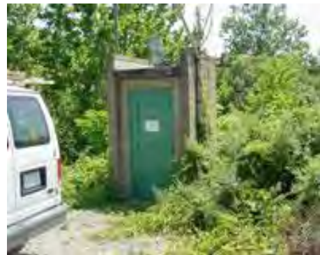
USGS Gage 03085500 Chartiers Creek at Carnegie, PA Source: USGS, 2010
