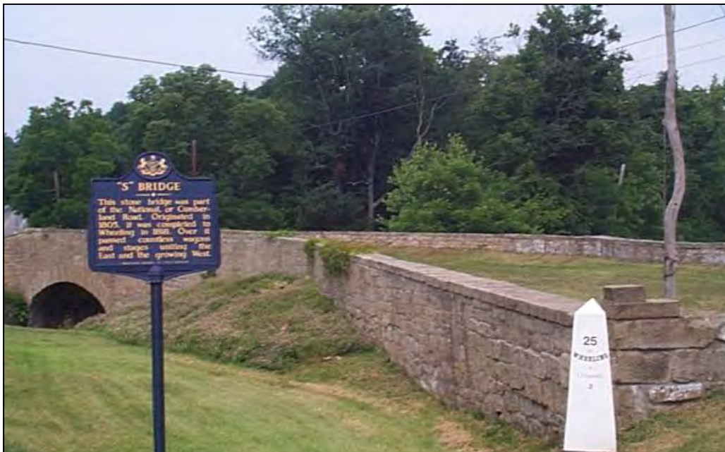
US Route 40 National Road S Bridge, 2002
