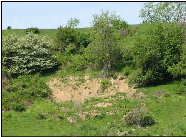
Landslide in Washington County, 2006
