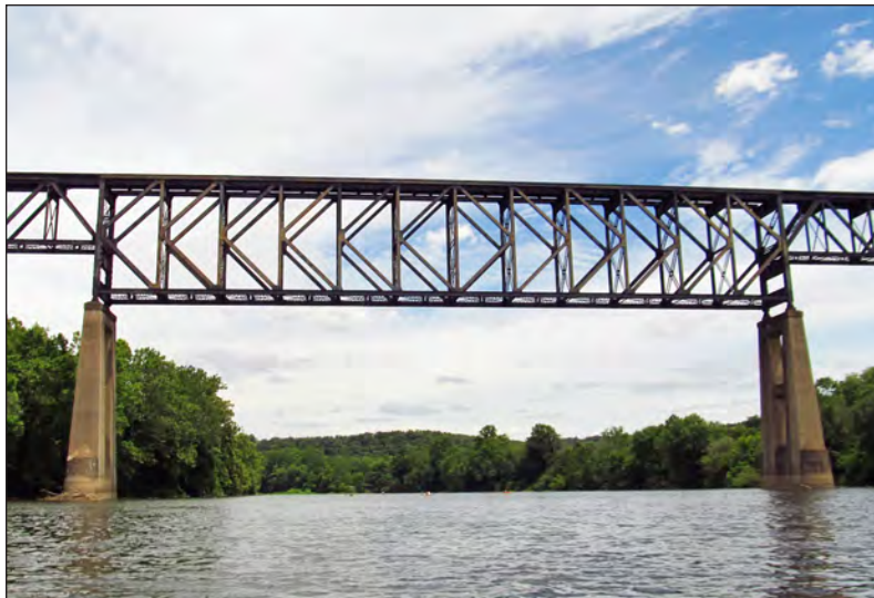
Bridge over the Youghiogheny River at its confluence with Jacobs Creek
