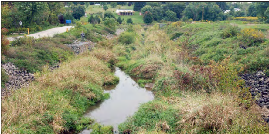
Jacobs Creek - Stream Stabilization
