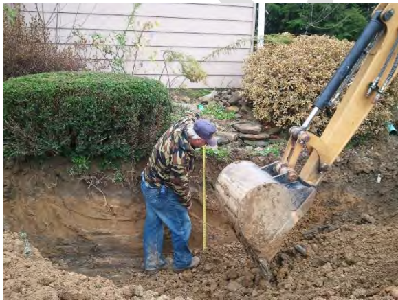
Excavate a drywell at least 10' from foundation
