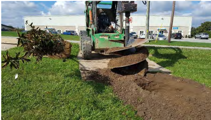
Plywood sheets protect lawn from compaction
