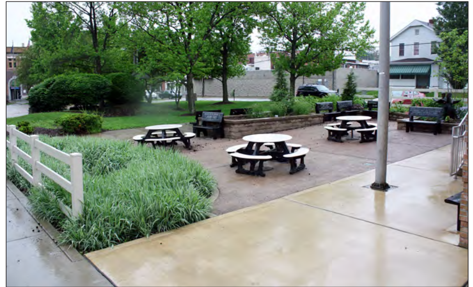
Rain garden and permeable paving in Scottdale Library's reading garden funded by EPA 319, 2011
