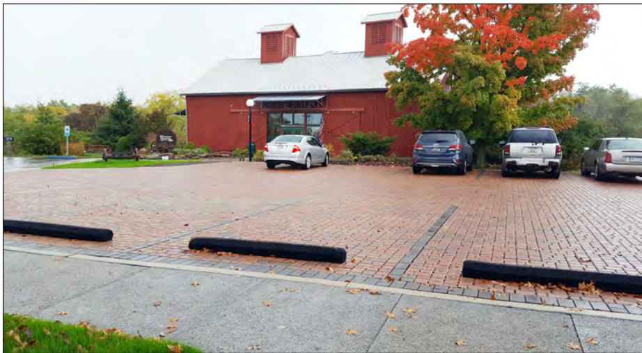
Permeable paving parking demonstration at the J.Roy Houston Conservation Center funded by Richard King Mellon Foundation, 2016.
