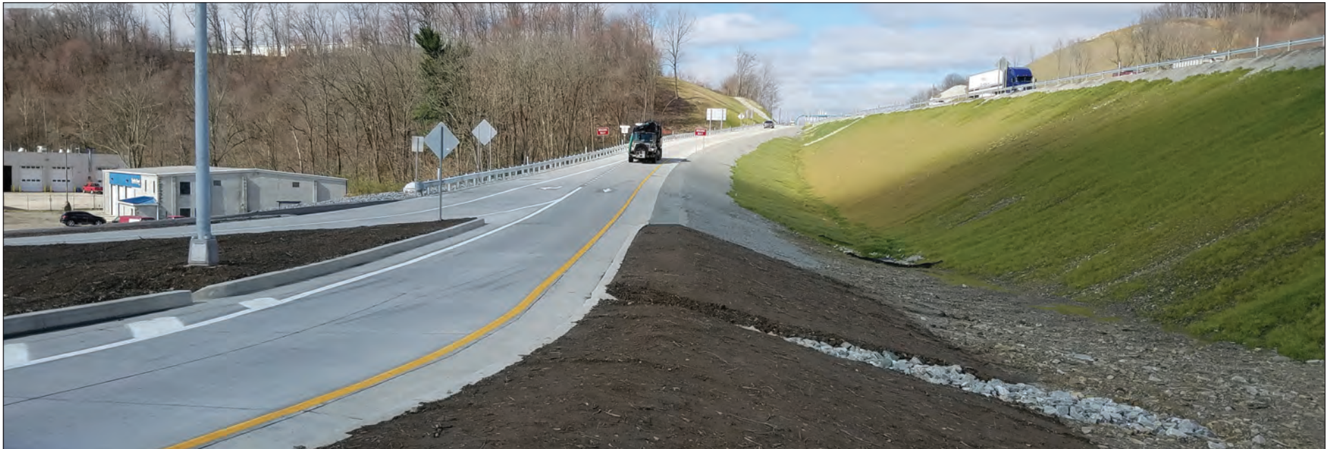
A view of an eastbound off-ramp at the improved Interstate 70 near New Stanton, PA
