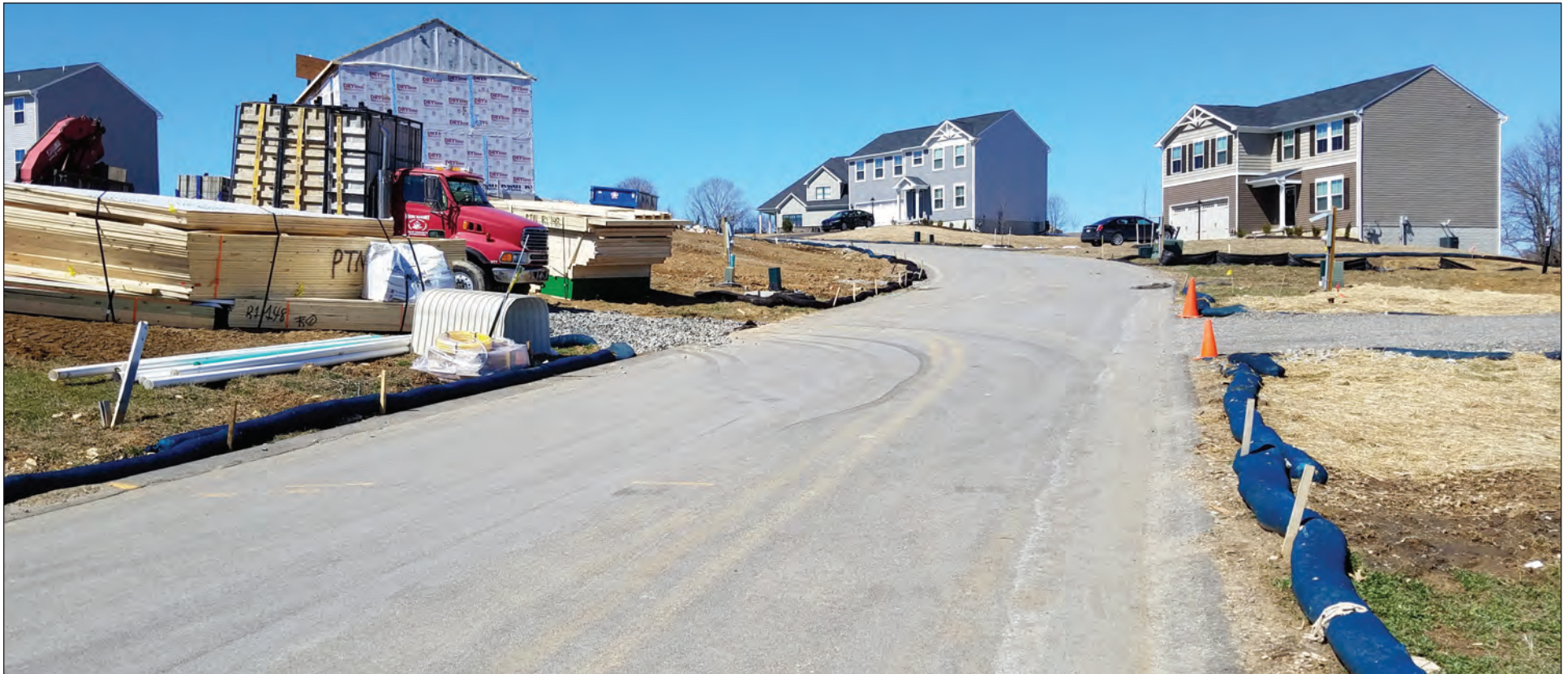
Erosion control barriers prevent sediment-laden water from leaving construction sites under Chapter 102.
