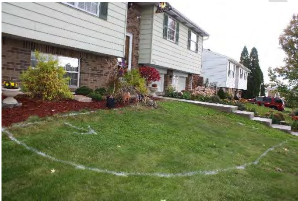
Mark rain garden location to avoid utilities
