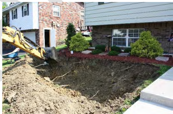
Excavate rain garden at least 10' from foundation
