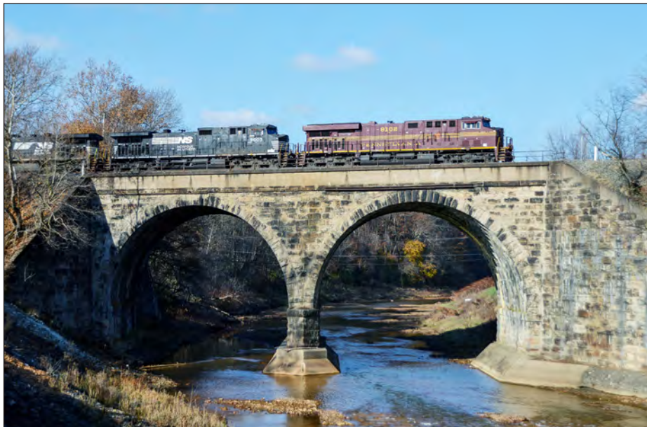
The Pennsylvania Railroad built bridges and tunnels, moved mountains and relocated streams, bending nature to their will for many years as the economic powerhouse in the state. Today many of the civil works of the railroad remain in daily use, well over a century after their construction.
