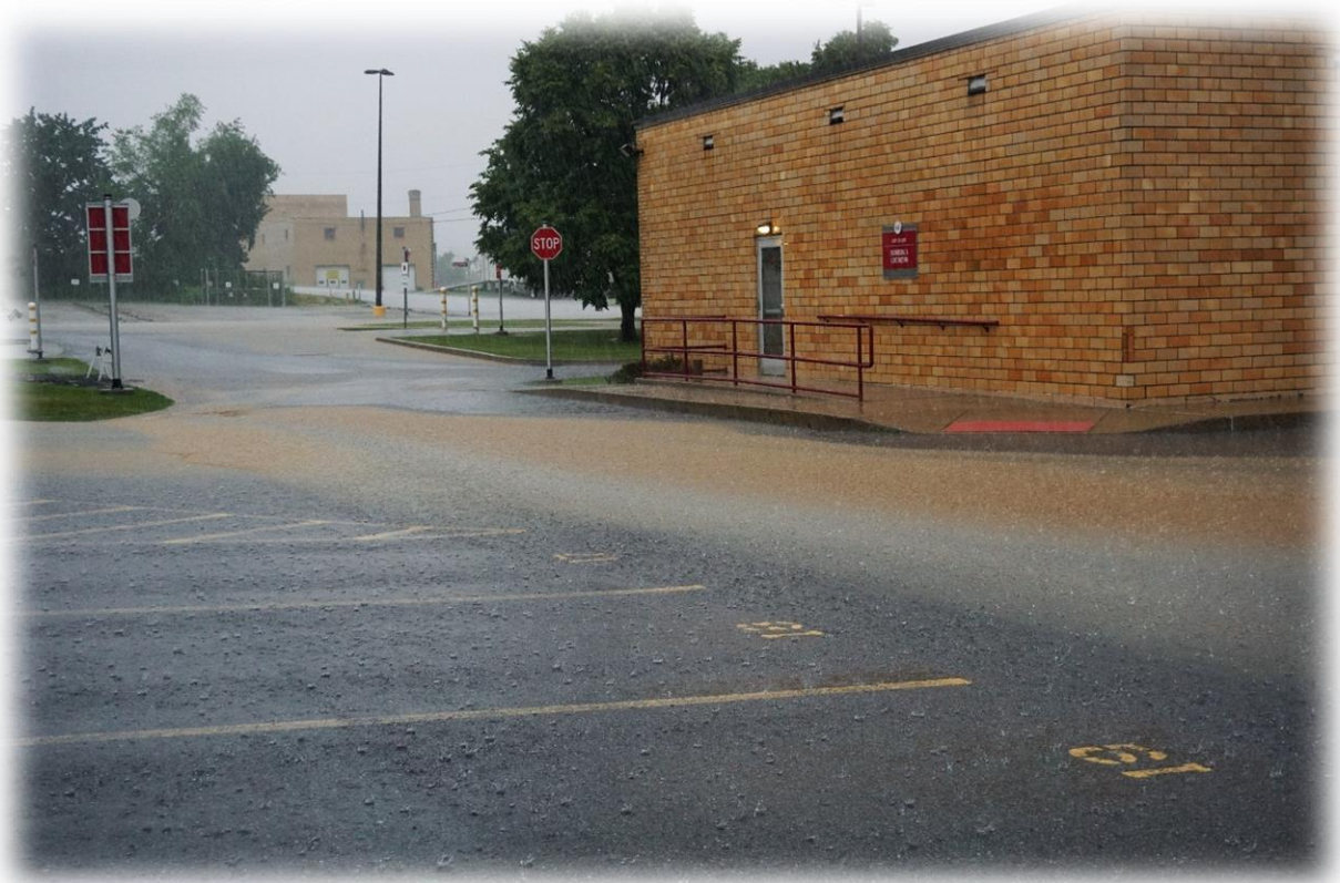
Figure 183 – Stormwater created a stream in a parking lot at Indiana University of Pennsylvania and caused flash flooding during a deadly storm on June 22, 2017
