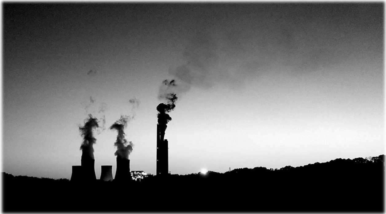
Figure 25 – Keystone Generating Station at dusk
